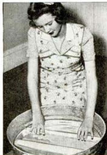
Left, immersing strip of wallpaper in tub to wet the adhesive on back. Right, unrolling moistened paper on the wall and sliding it into place
