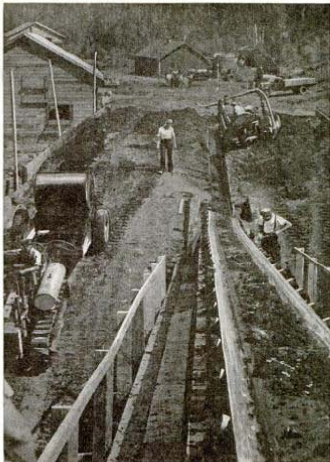
Rubber belt on conveyor lifts tarlike sand from pit to processing plant. Below, a geologist is lowered by rope on sand cliff
