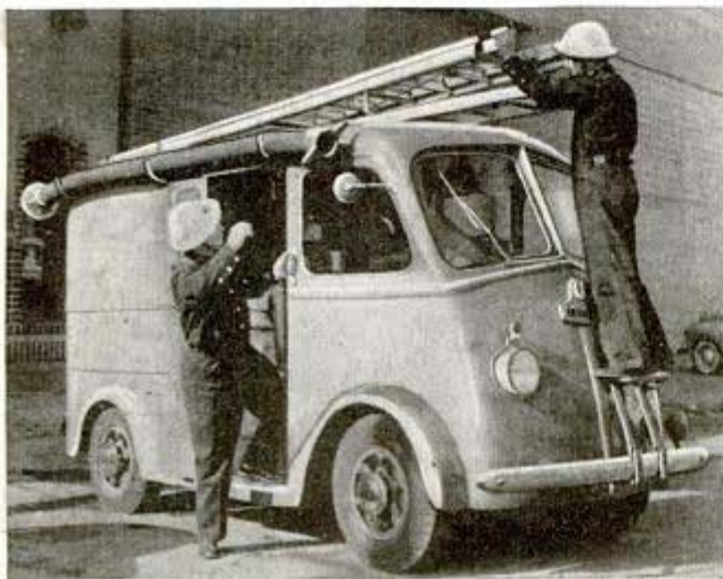
Truck type familiar as a delivery car carries auxiliary firemen's equipment
