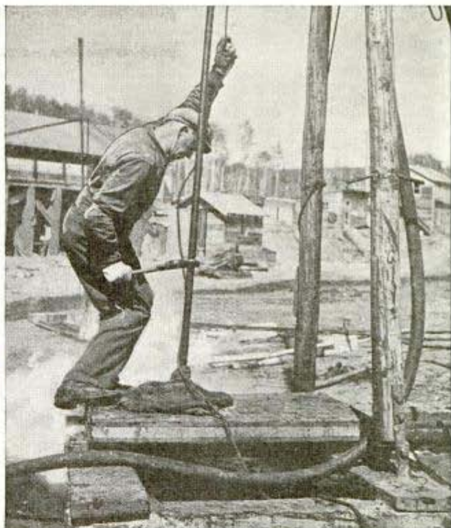
Steam drill making deep hole for dynamite to loosen sands
