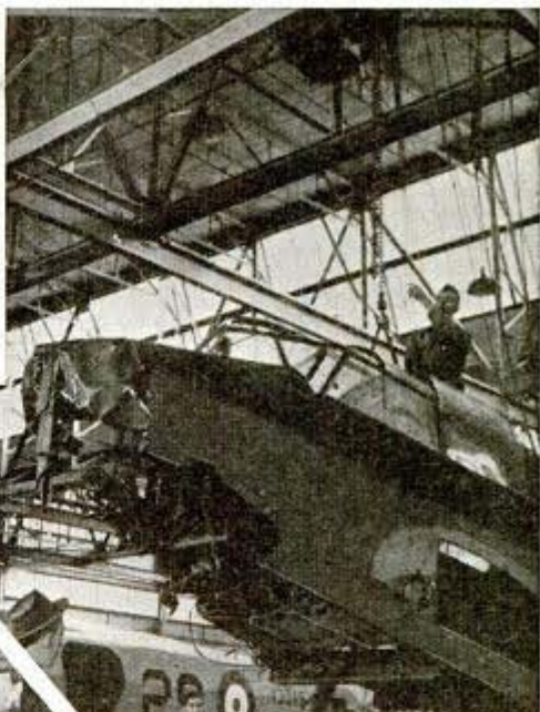
Wrecked in crackup or combat, (above) planes are shipped from overseas zones of combat. Often wings are nearly shot off, or noses smashed, but in about three weeks of "face-lifting" they emerge, almost as good as new
