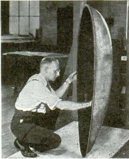
Half of a droppable fuel tank—a Duramold product
