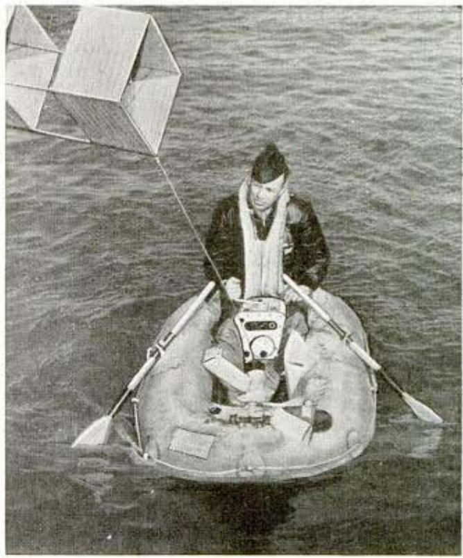
Box kite serves as aerial for automatic radio that sends out distress signal from life raft which will support two fliers
