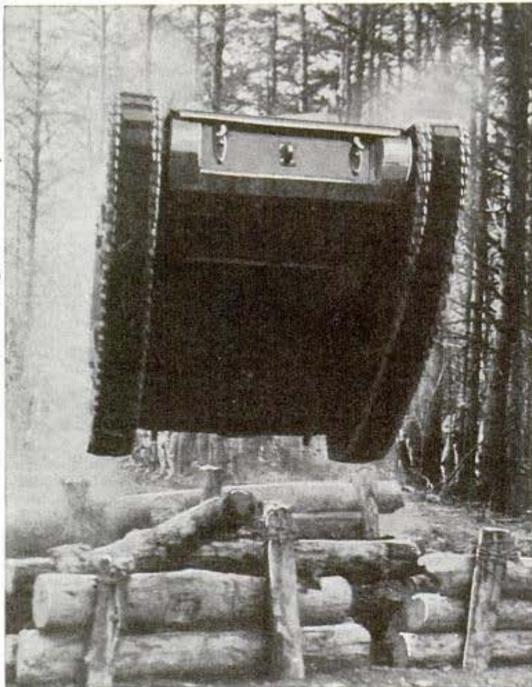
Timber barricade thrown up by army engineers hurls trapped tank in air
