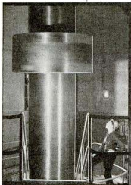
↑ This mighty shaft, four feet in diameter, 73 feet high and weighing about 200 tons, enables waterwheel of Grand Coulee's turbines to turn generators
