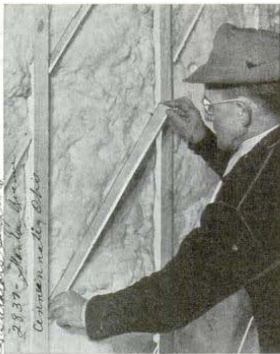
Slot in end of retainer fastens it in place over nail
