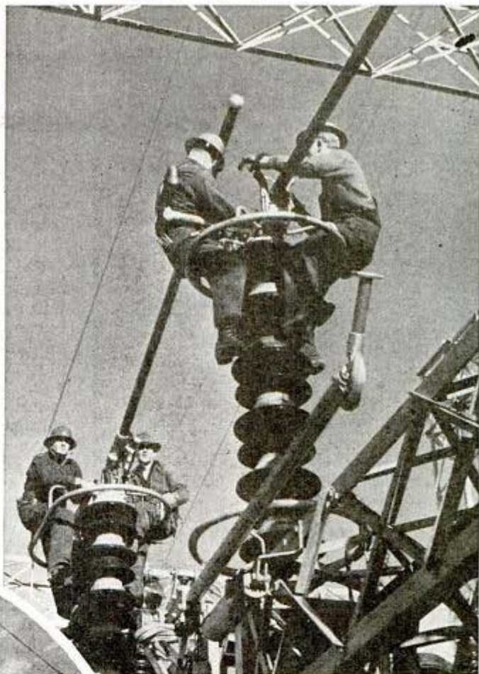
The warriors above wear helmets, too, but their job is not killing Japs or Nazis. They are constructing switches outside power plant
