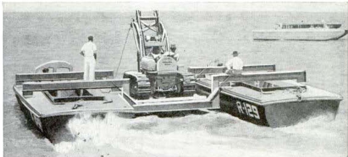
Such heavy machinery as tractors and bulldozers, needed immediately to build airfields or prepare the ground for cantonments, are landed directly behind invading troops by landing-barge ferry
