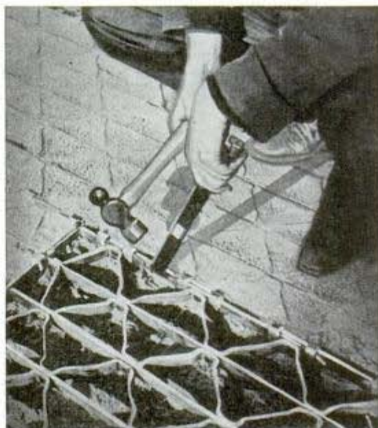
Hammer and pronged tool lash road gratings together
