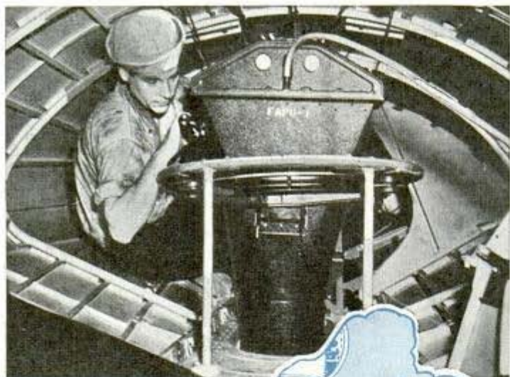
This big mapping camera is shooting earthward from a "Catalina"
