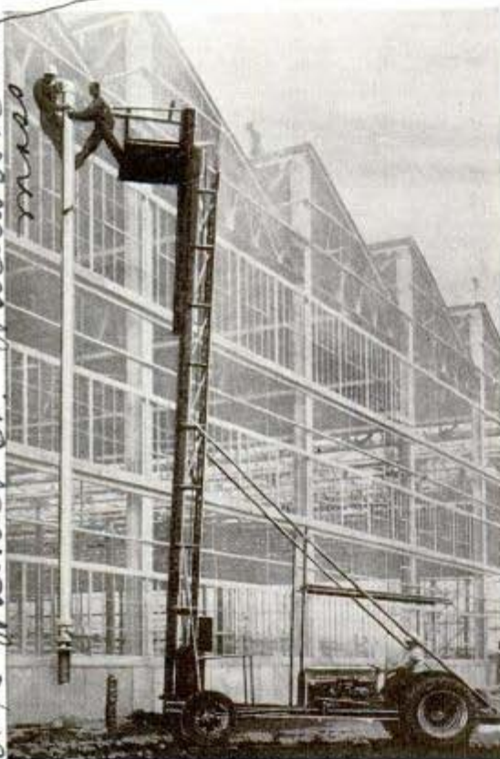
Cranes lower 142-ton locomotive to its chassis. Below, 40-foot telescopic platform extends man's reach
