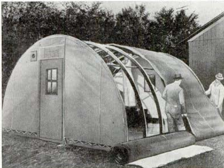
Fireproof walls of shelter roll up like blanket, pack easily in plane
