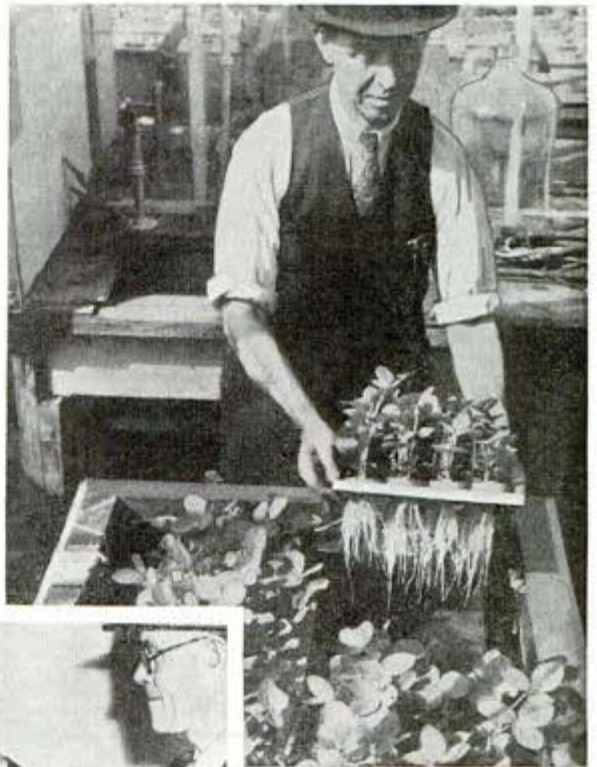
The vegetables above are being grown in controlled water baths to test the amount of minerals necessary for all-around growth
