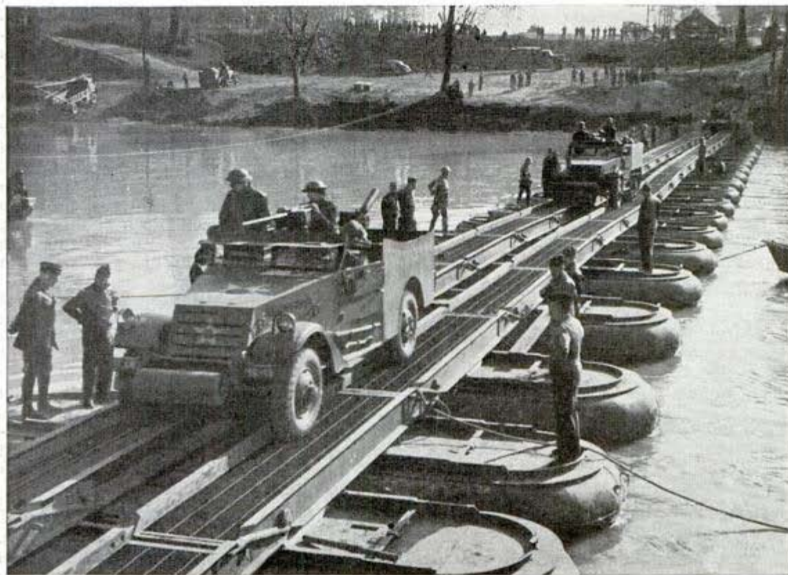
Temporary ponton bridge of rubber rafts filled with carbon dioxide gas carries armored cars across a stream U. S. Signal Corps photo
