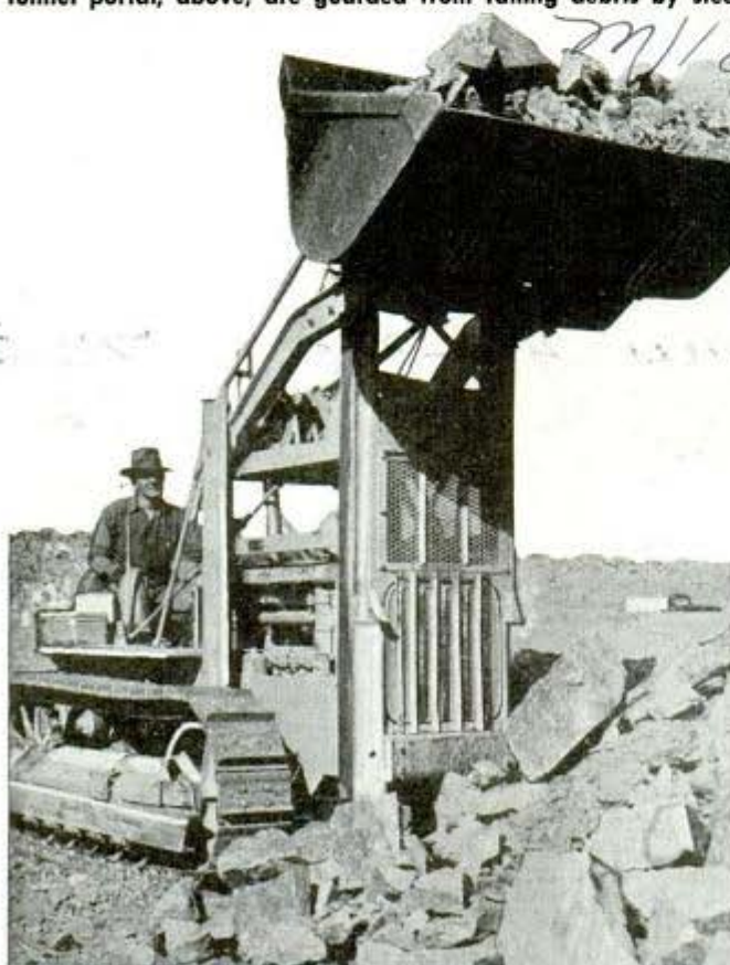
War "orphans" some highways, requires building of others. Workers at tunnel portal, above, are guarded from falling debris by steel shield
