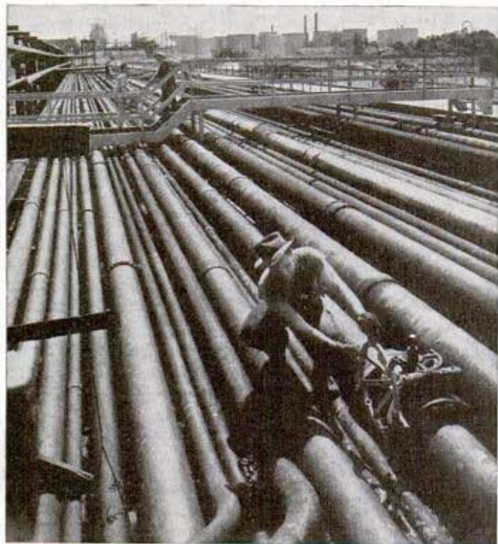
Top, a worker turns valve controlling flow of crude oil at new catalytic cracking plant which has few moving parts, machines or wheels in motion. Below, pipe lines leading to "cat cracker" Standard Oil of New Jersey photos
