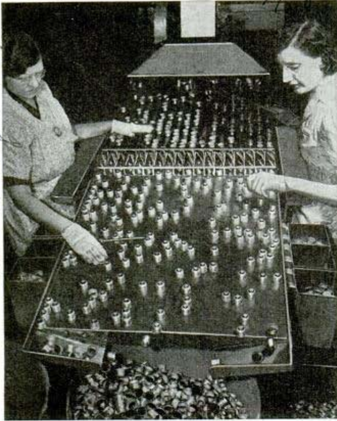
Inspectors' sloping table vibrates to keep lamp bases moving
