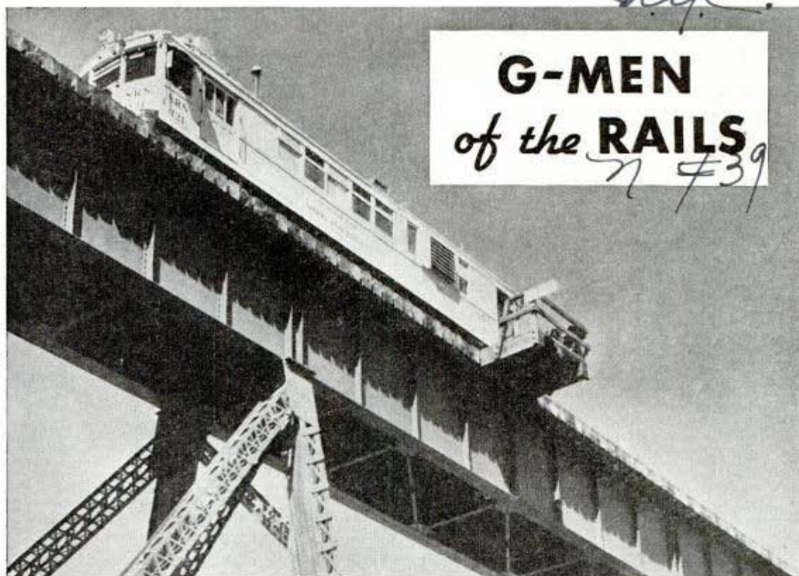
High on the rails and also high in the respect of railroad men is this detector car, one of a fleet guarding lives of passengers by finding tiny rail defects invisible to the human eye
