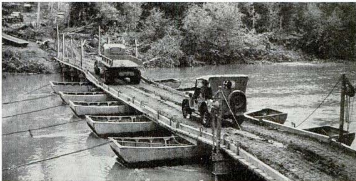
Scale models of new bridges, such as one shown above, are not possible on hurry-up job like the Alaska Highway, where pontoon span (below) was built
