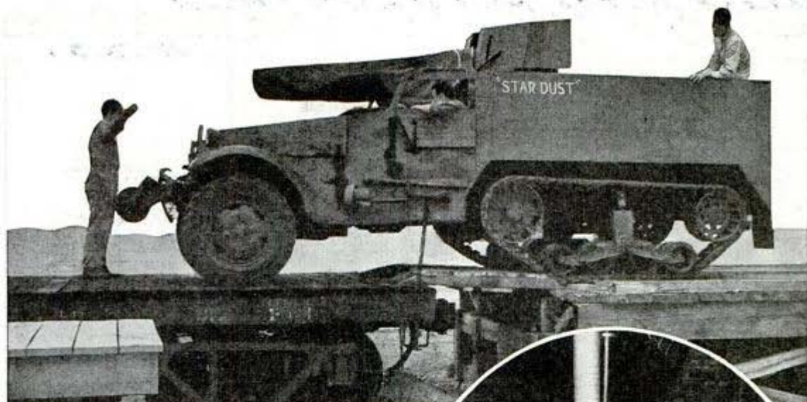
One of the army's "half-tracks" crosses the spanner from ramp to flatcar of the "Berlin-Tokyo Express"
