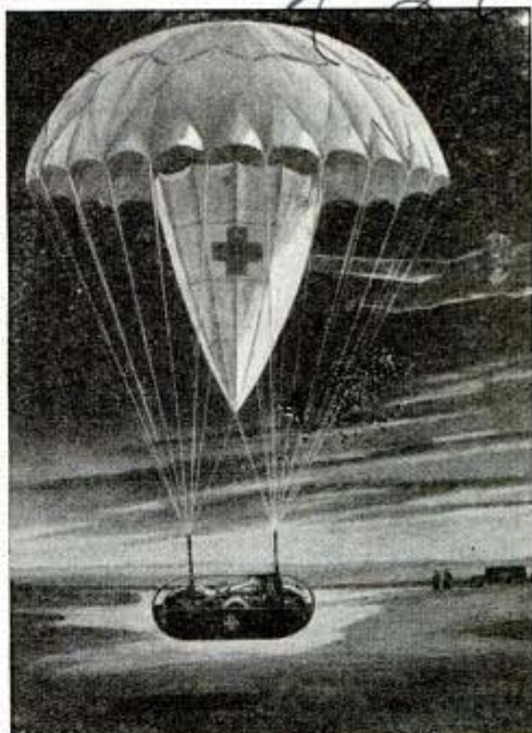
Inverted cone directs air into slits in parasol, relieving the shock when new parachute opens, even at low altitudes, (above). At right, it drops motorcycle in its own trailer
