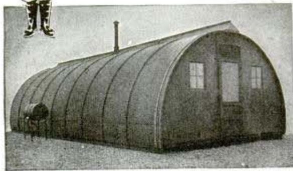
Prefabricated, demountable Army hutment for 16 men. Made by Pacific Huts, Inc., Seattle, Wash. Curved ribs laminated with CASCO-RESIN (liquid) Resin Glue.
