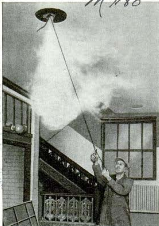
Hot steam melts covering on old wire stuck to tube
