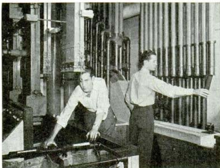
Blueprints are shot to various departments at Douglas by these tubes
