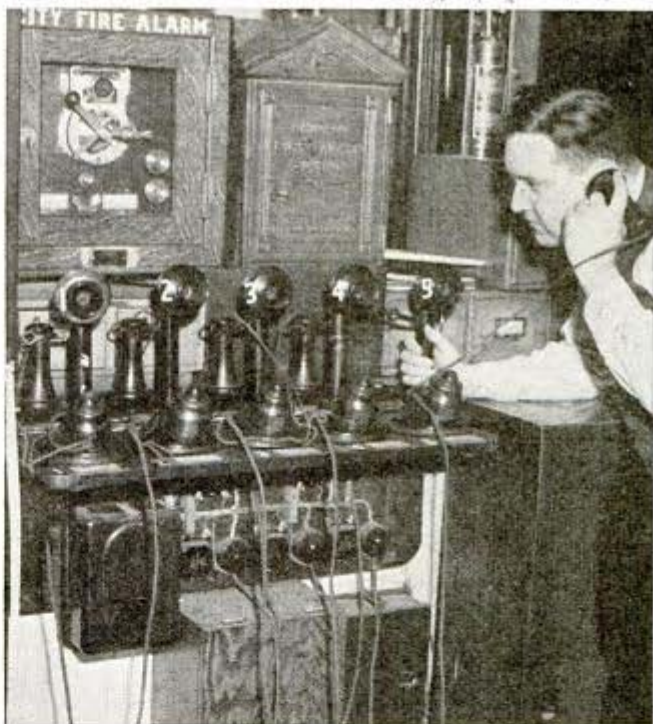
↑ These "blackout" phones with red bulbs on base are used by fire department to contact 13 air raid watch stations
