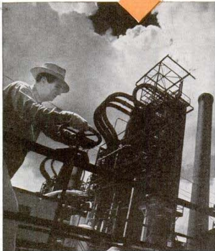
Top, a worker turns valve controlling flow of crude oil at new catalytic cracking plant which has few moving parts, machines or wheels in motion. Below, pipe lines leading to "cat cracker" Standard Oil of New Jersey photos
