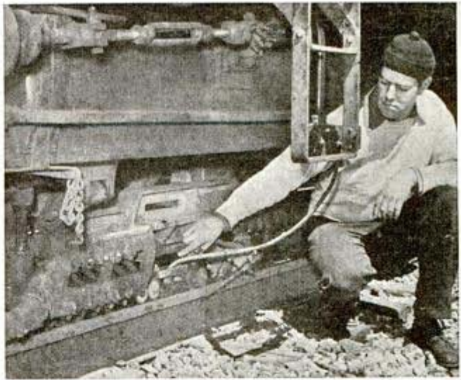
Rail G-man points to unit under car which automatically sets off paint gun to mark defective point revealed by "searcher"
