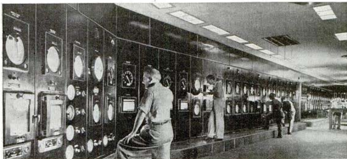
Eight of the nine men needed to run a huge "cat" cracking plant are shown in control room above. Right, cost of a gallon of high-octane gasoline has dropped from $20 to 15c
