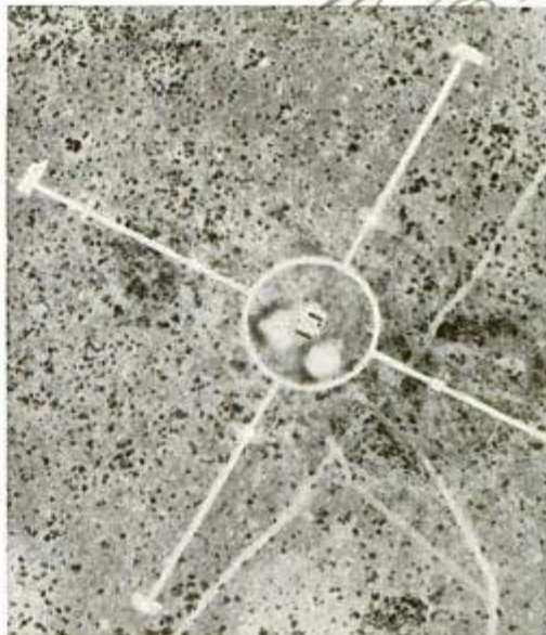
Aerial view of target range (above) shows how four microphones are placed in square pattern. Top left, map model of range. At left, closeup of "pillbox" for microphone
