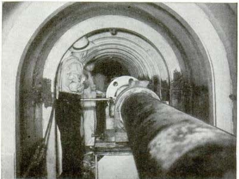
Skid frame (left) holds life raft poised ready to slide into water at instant rope is cut. Below, outfitting engineers line up propeller shaft with boring of frame
