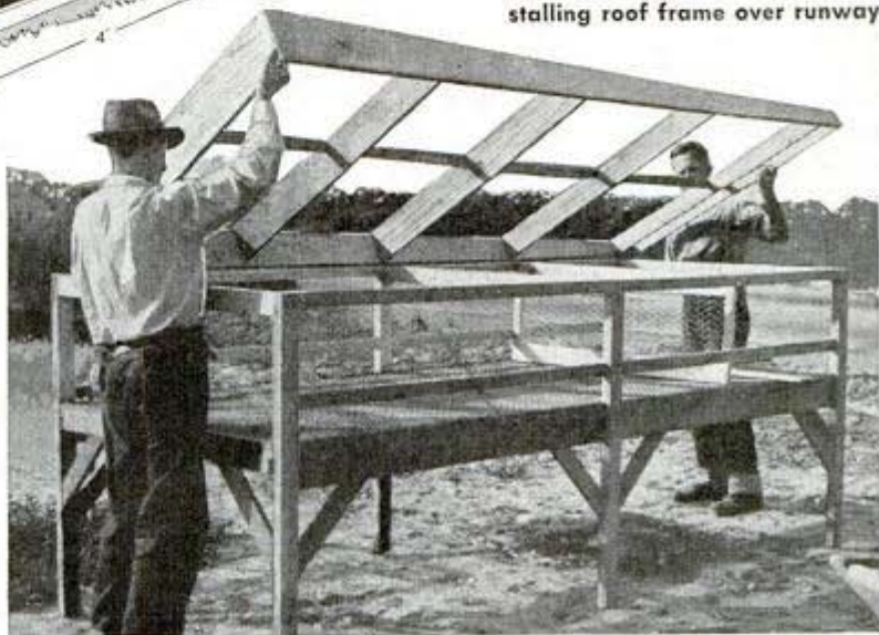
Brooder, shelter house and runway are designed so they may be latched together. Below, installing roof frame over runway
