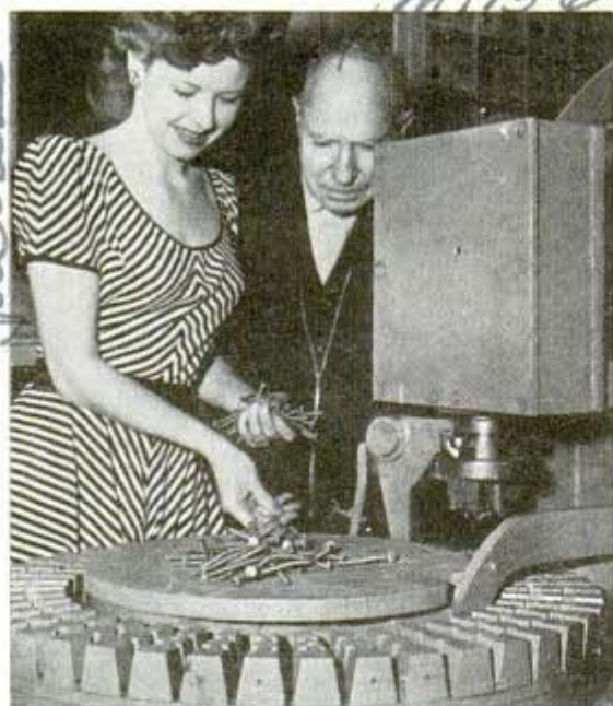
Straightener removes kinks to reclaim bent nails
