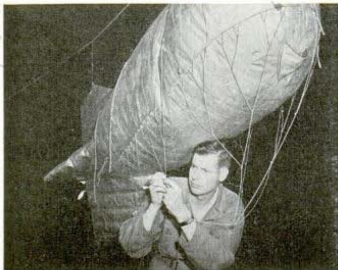
Down she comes, as a motor-driven winch winds in the steel cable holding balloon
