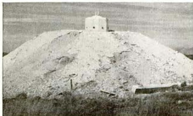
Aerial view of target range (above) shows how four microphones are placed in square pattern. Top left, map model of range. At left, closeup of "pillbox" for microphone
