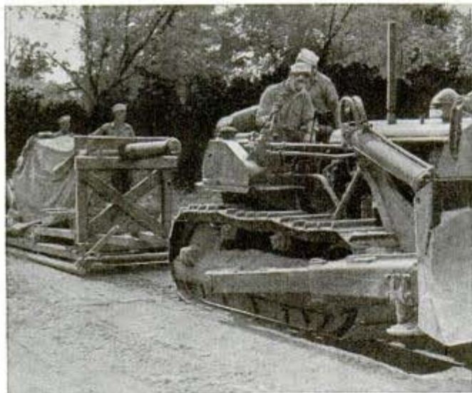
Once the Marines have seized a beach, Seabees move in to fortify it. Above, towing 4-inch gun on skids with bulldozer
