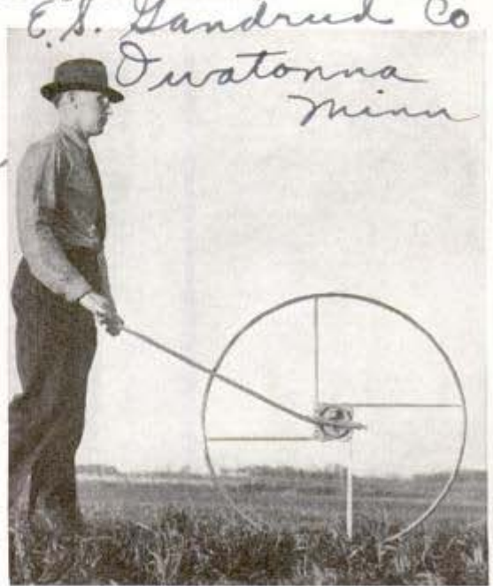
Large wheel measures in 10-foot lengths as it rolls
