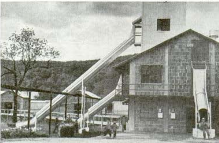
The tubular chutes leading from this U. S. Army munitions loading plant are emergency exits
