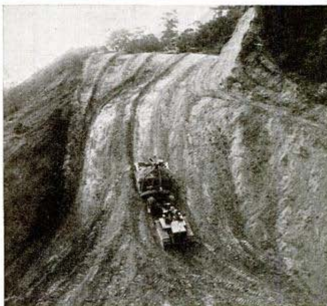
A fleet of ten Caterpillar tractors pulling scrapers is making the cut at right on the highway to Panama in Costa Rica
