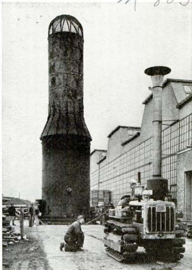
Incinerator weighing 100 tons starting 300-foot journey at tractor plant
