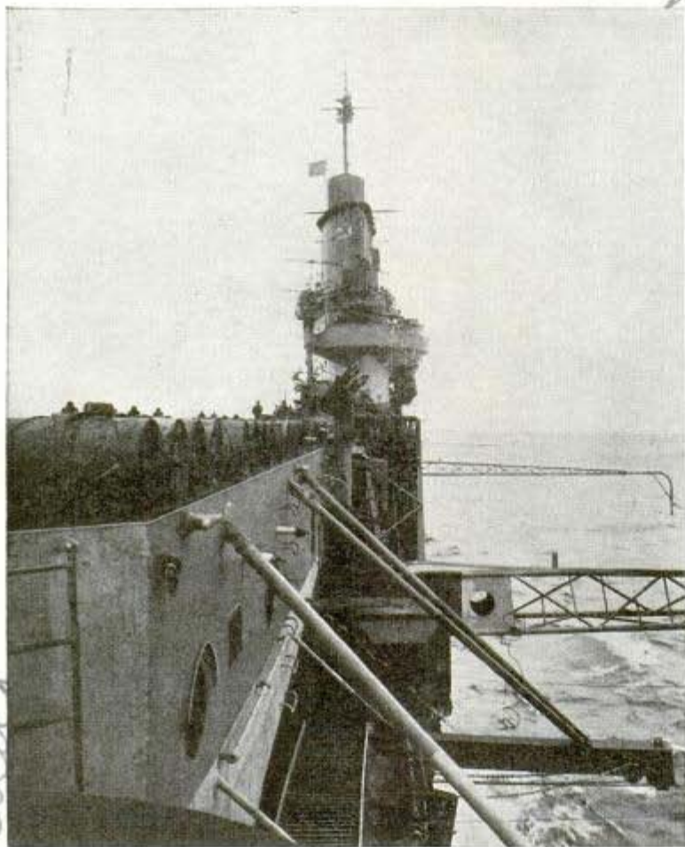
Starboard view of giant aircraft carrier headed toward sea, the control tower—or "island" as navy men call it—rising high above the deck. Officers of the flattop direct operations from vantage point of tower
