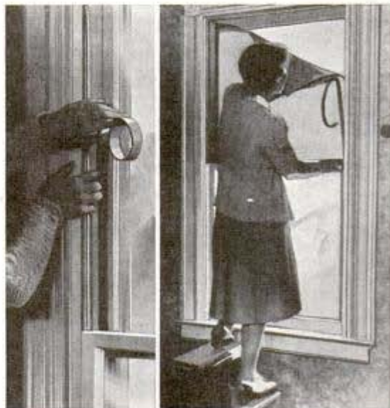
Sealing crack with tape (left), and applying shield
