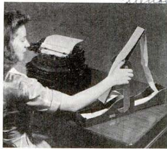
Rotating easel holds Stenotype note tape at eye level of typist. Twirling the wheel turns arm end over end, causing it to deposit finished portion of tape into one tray and pick up fresh notes with little loss of time
