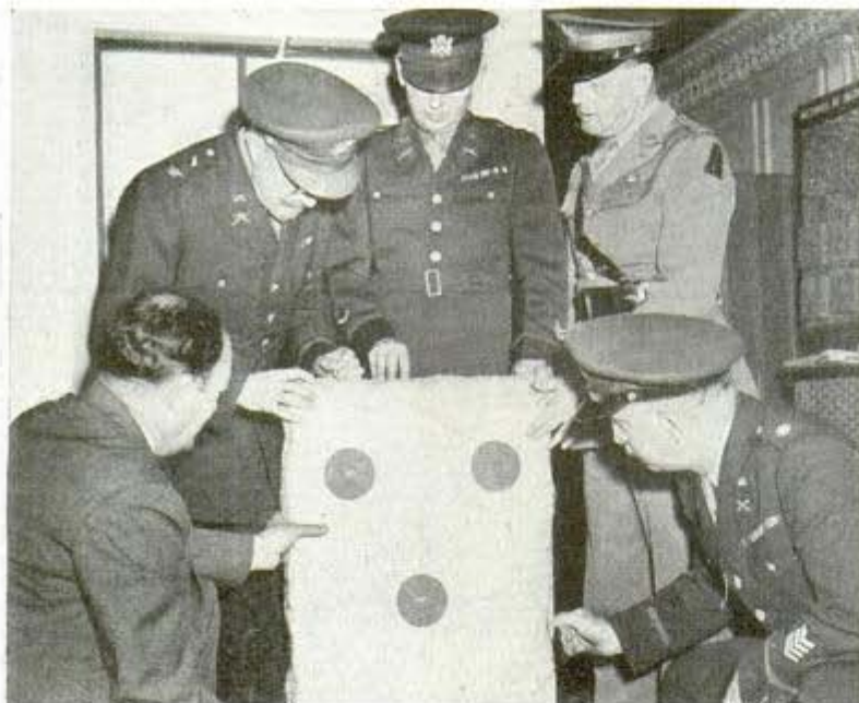
Made of a blast-cushioning glass fiber material, this mattress was designed to protect electrical switchboards and instruments from bombings
