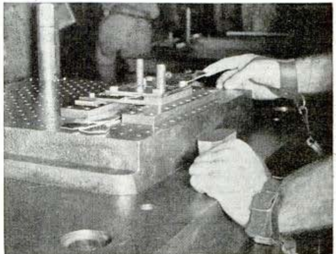
Dirt and fumes in the eyes, ears, nose and pulmonary tract would wear down and slow down the worker, so this American Airlines man is masked as he cleans motor parts with air gun
