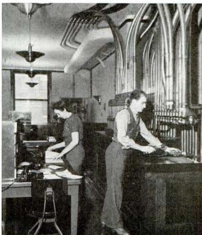
Pneumatic tubes at a railway telegraph office dispatch train orders to train crews
