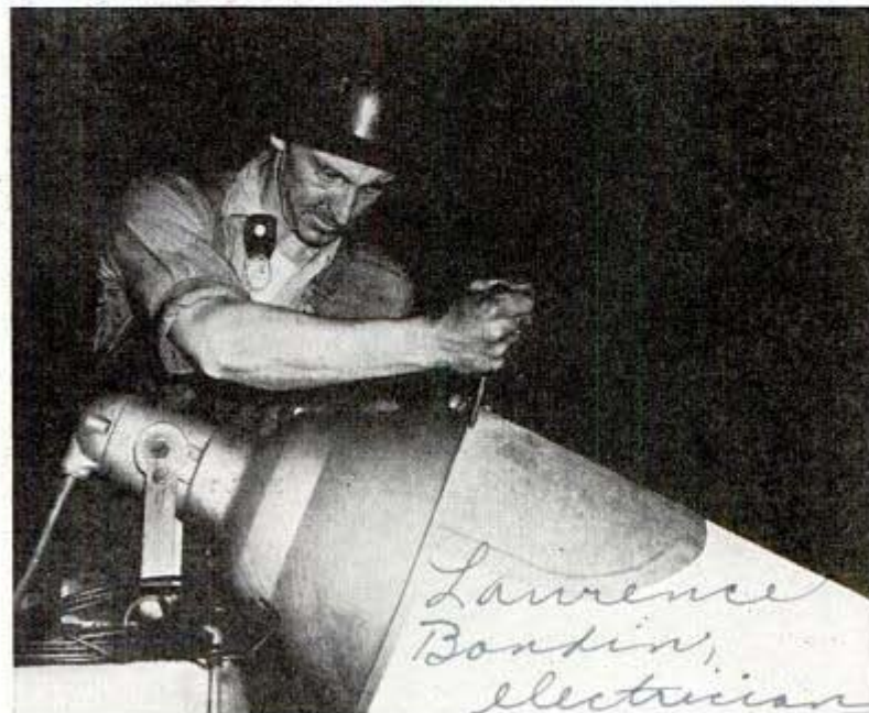
Attaching visor to a floodlight in shipbuilding yard on coast hides the glow from subs and permits night workmen to "keep 'em rolling"
