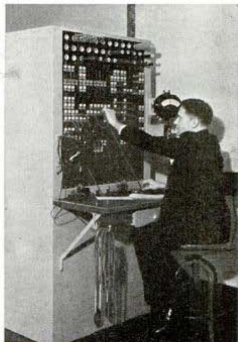
Inside the railway post office car, left, clerks are busy sorting and distributing the last-minute mail. The wire chief of the Santa Fe railway, right, tests telegraph circuits essential to on-time operations
