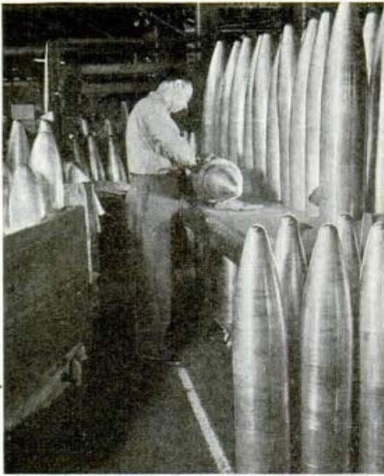
Powder containers for 15-inch shells are of aluminum
