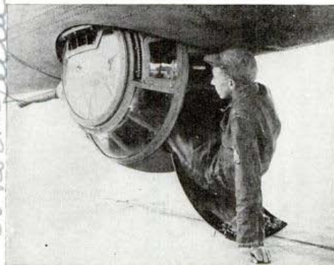
Gunner curling himself into "belly bubble" to man bomber gun
