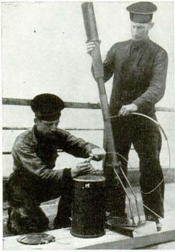
These rocket projectors send aloft parachutes from which wires dangle to ensnare enemy planes
