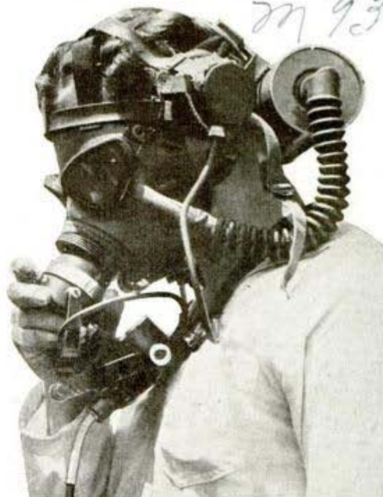
Navy gunner talking by means of gas-mask "mike"
