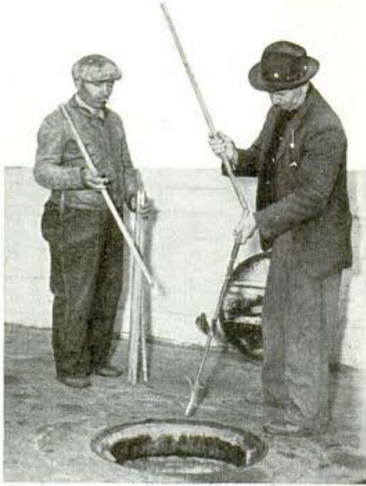
Sunlight is made to turn corners with mirrors and safely illuminate hundreds of feet of sewer conduits Cleaning a clogged pipe with harpoonlike instrument
