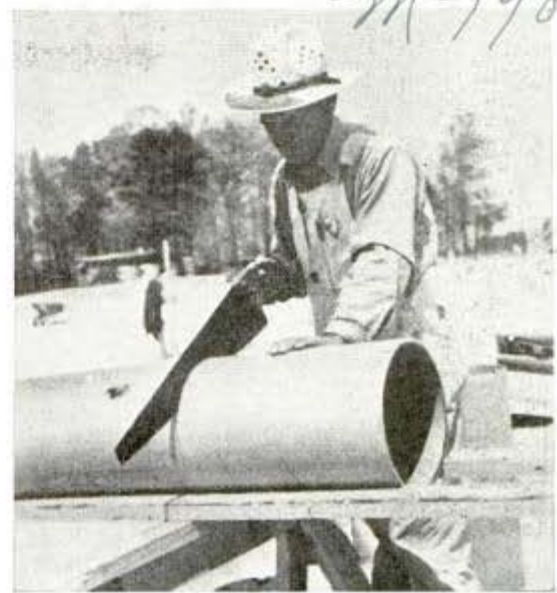
Sawing a tube to required length for building pier
