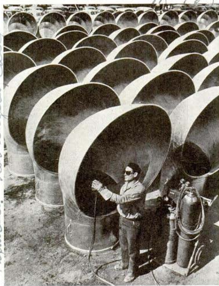
Ventilators get visit from welder who applies needed reinforcement
