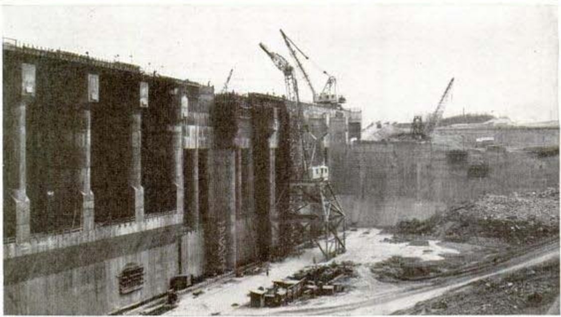
When Kentucky dam, near mouth of the Tennessee river, is completed it will create new inland lake of 256,000 acres. The $107,500,000 dam will be 166 feet high and 8,650 feet long
