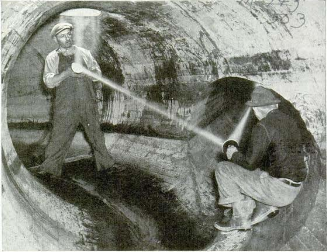
Sunlight is made to turn corners with mirrors and safely illuminate hundreds of feet of sewer conduits Cleaning a clogged pipe with harpoonlike instrument
