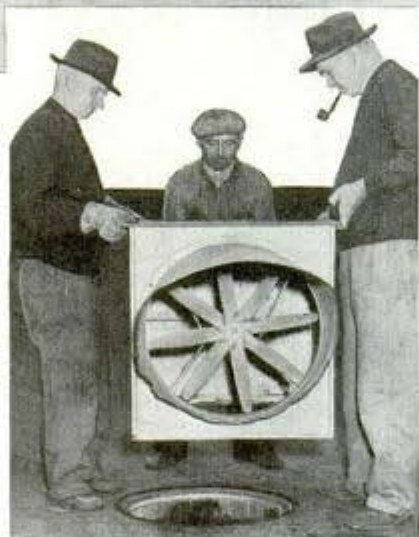
An electric fan is placed over a manhole to blow fresh air below to workmen combatting the fumes of sewer gas
