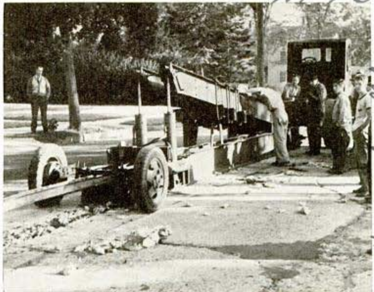
Hydraulic lifters raise beam to uproot tracks from city's paved streets
