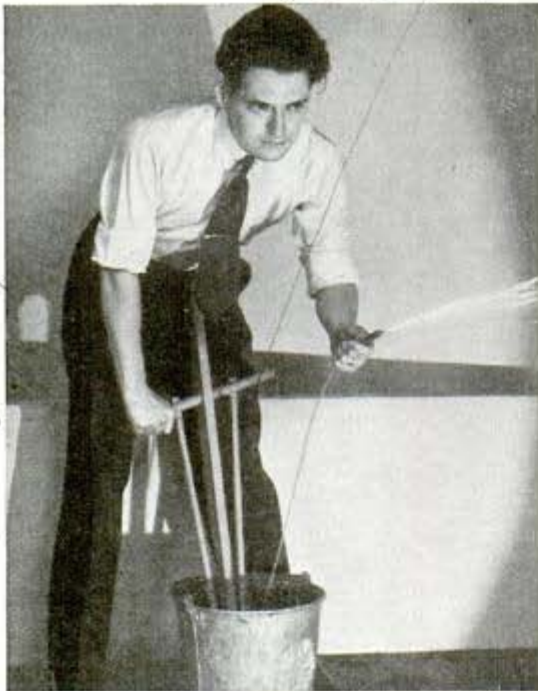
Wooden "victory pump" for extinguishing bombs, small fires or watering garden uses no critical metal
