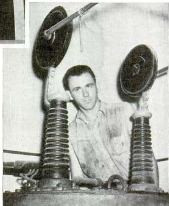
Below, inspecting huge insulators above a transformer for big electrical precipitator
