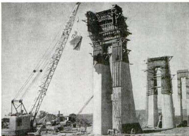
Diesel-operated dragline with 90-foot boom sets forms for a rail bridge
