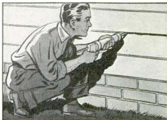
ALL CRACKS AT DOOR AND WINDOW FRAMES, AND THOSE BETWEEN WARPED SIDING, SHOULD BE FILLED WITH CALKING COMPOUND.
