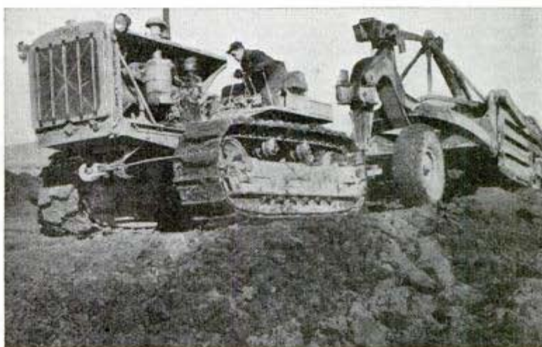
Scraper carrying 13-yard loads helps grade land for a new ordnance plant
