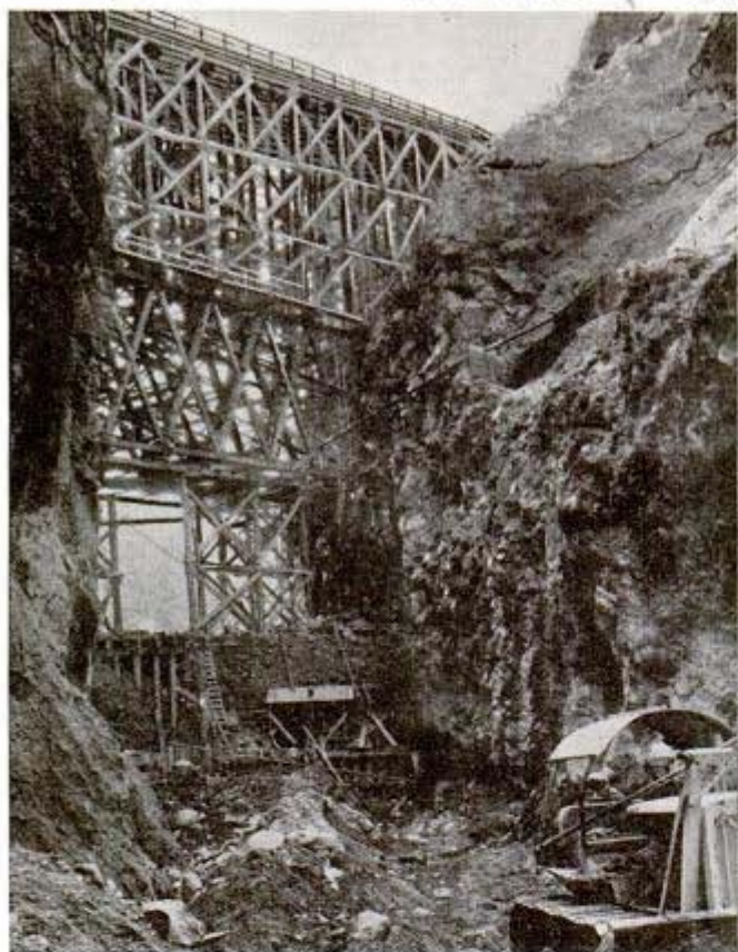
Diesel equipment works at bottom of a new dam in northwest
