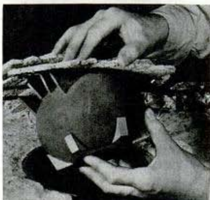
James C. Boudreau, head of Pratt Institute Art School, operates machine which duplicates sun-shadow conditions at any given moment of year
