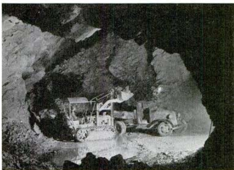
A compression-ignition excavator "mines" limestone for war construction
