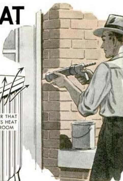
ALL CRACKS AT DOOR AND WINDOW FRAMES, AND THOSE BETWEEN WARPED SIDING, SHOULD BE FILLED WITH CALKING COMPOUND.
