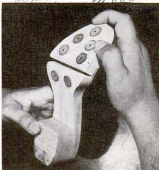
Hinges give flexibility to wooden sole for war shoe
