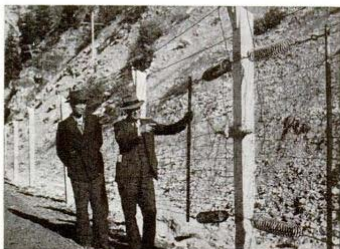
↑ Electric slide detector fence warns the engineer of landslide
