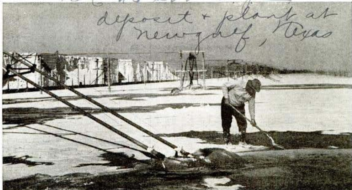
Hot molten sulphur flowing from mine into six-acre vat to form solid "cliffs" like those in background
