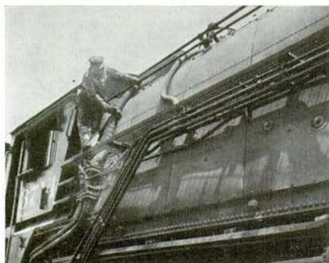
Making careful inspection of engine before setting out from Denver for Salt Lake City via lofty passes, tunnels, desert
