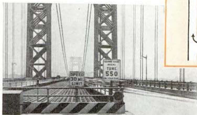
Diagram shows the radio traffic control installations used in a test on the George Washington Bridge in New York City. A sign on the bridge, left, tells motorist where to set his auto radio dial to receive the broadcast
