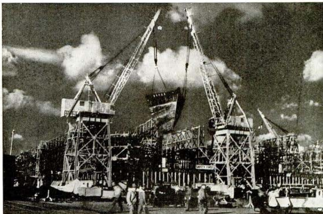
Cranes lowering the completed forepeak in place on ways
