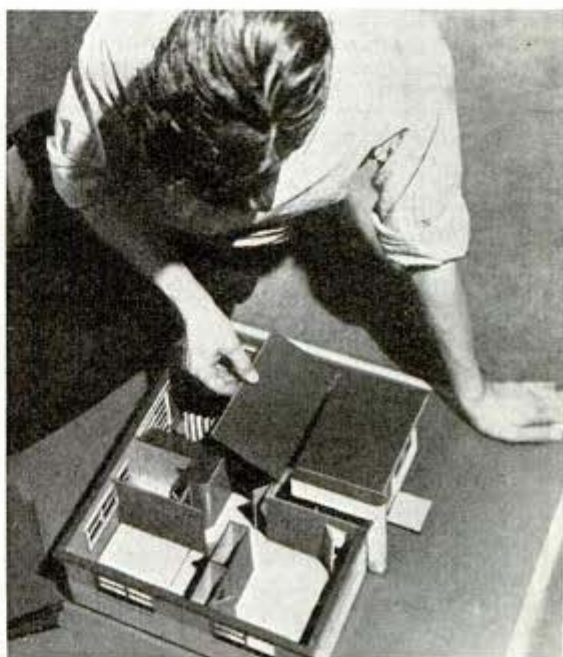
Lifting off the roof and tipping back the walls of the model at left shows a prefabricated bathroom unit. Right, examining a Norman Bel Geddes model home featuring a roof that comes complete in just six sections
