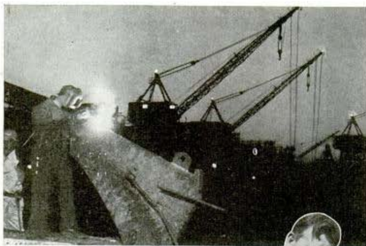
Welders on night shift complete the forepeak section in shipyard
