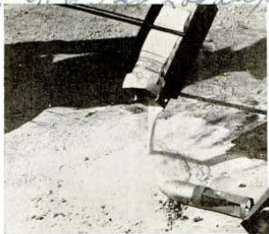
Extinguishing an incendiary by pouring chemically treated sand on it from a long handled holder
