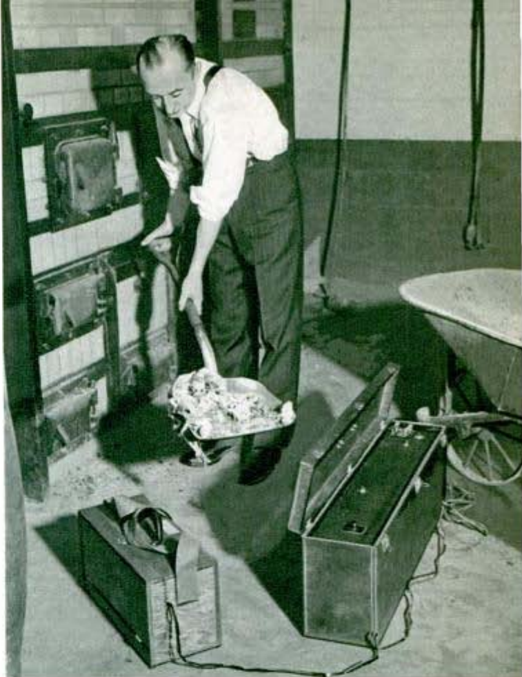
Frank Hartman, Philadelphia "radium detective," hunts lost radium in ashes from hospital incinerator with his "electric bloodhound." Below, making a radiograph of a metal casting with radium encased in aluminum "bomb"
