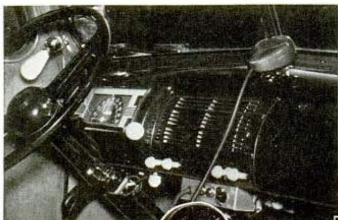
The instrument panel on your postwar auto may look like the one above equipped with a Link short wave set. Note microphone, top
