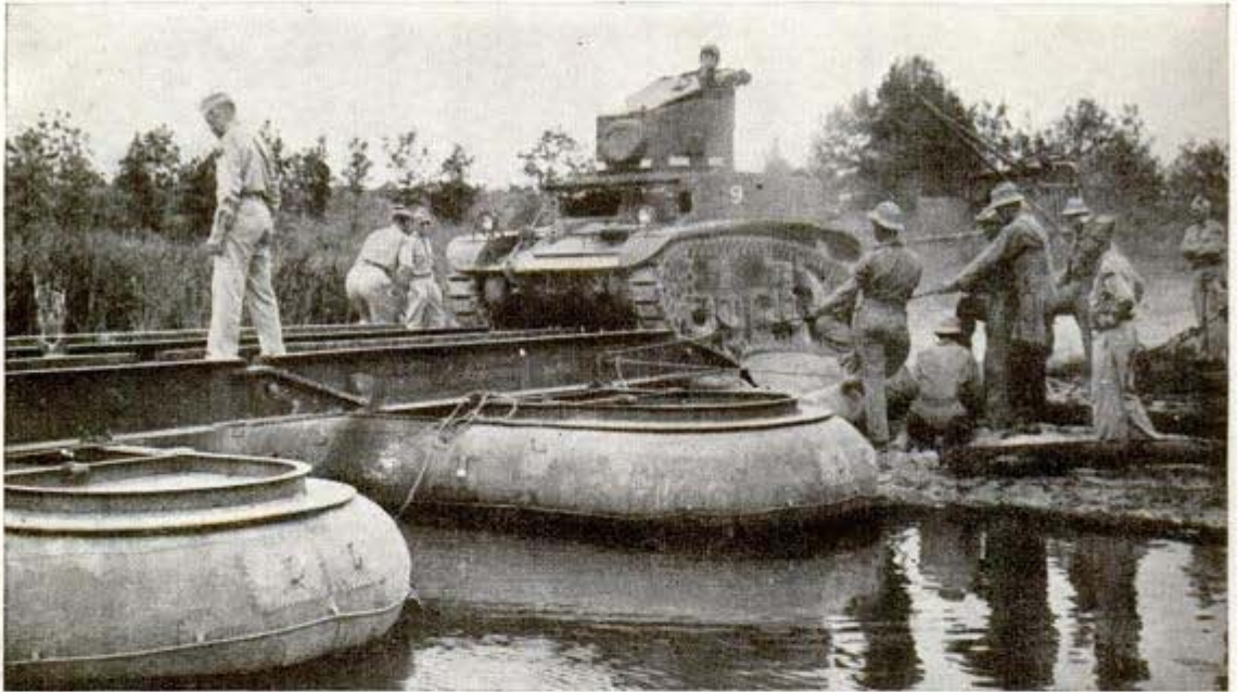
Tank moving across bridge made of heavy steel treadways supported by big rubber pontoons inflated with air
