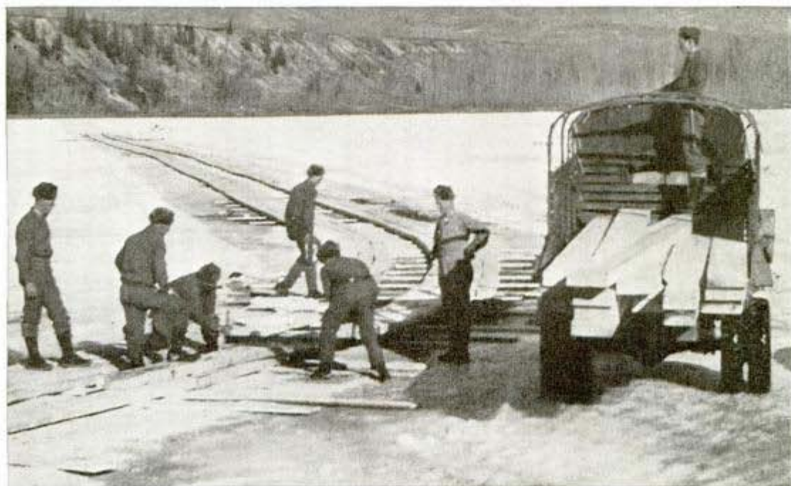
U. S. Army men lay planks across a frozen river in northwest Canada to help support the loads of road building material rushing north before the ice thaws
