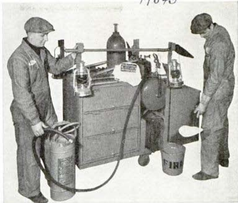
Completely equipped fire cart, handy for industrial plants and large buildings, can be wheeled in a hurry to any point endangered by bomb
