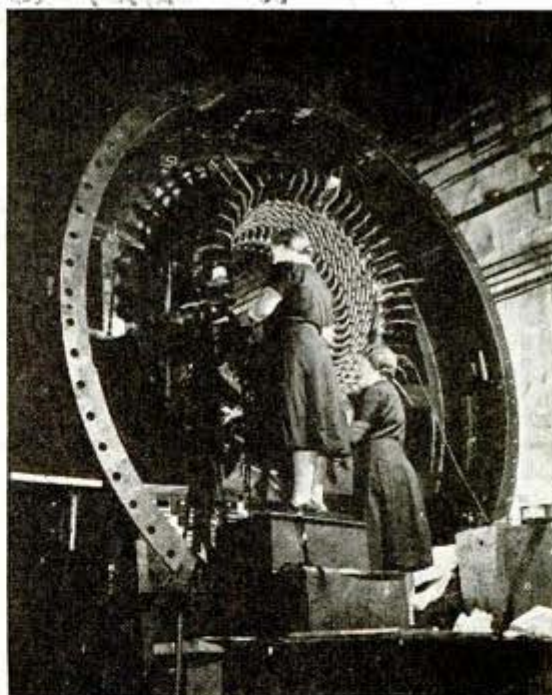
↑ Women's dexterous fingers excel at a job like this, winding insulating tape on a huge Westinghouse turbine generator that develops 65 million watts
