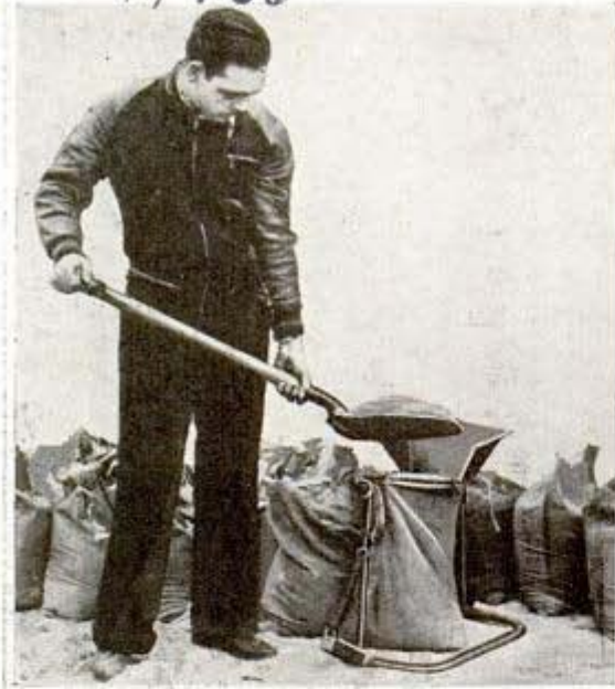
Adjustable holder has trough to guide sand into bag
