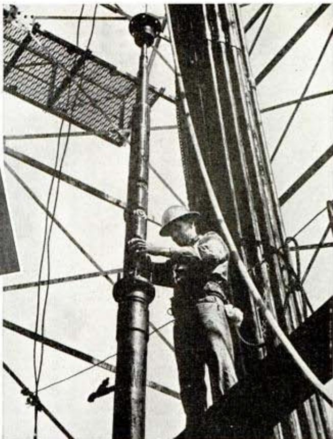
Photo from Lane-Wells Co.
