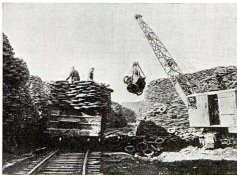
Eating into the great piles of cast-off auto tires is a crane used for loading cars that shuttle between the storage yard and reclaiming plant
