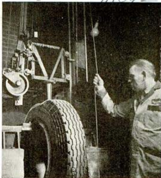
Testing a truck tire for resistance to sharp blow
