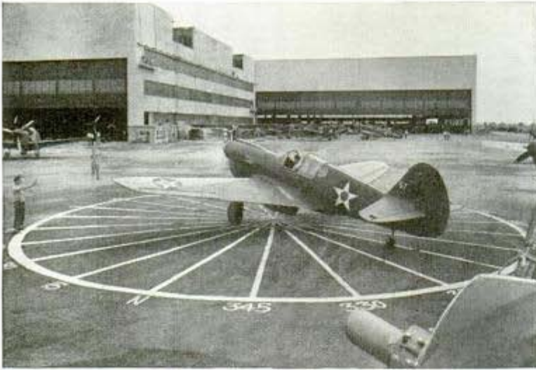
Compensating compass of a plane on compass rose at Curtiss-Wright plant
