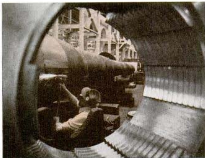
Through the breechblock seat of one big gun (above) you see a worker tailoring another major-caliber rifle barrel with a flexible-shaft grinder. Below, inspecting a huge naval casting
