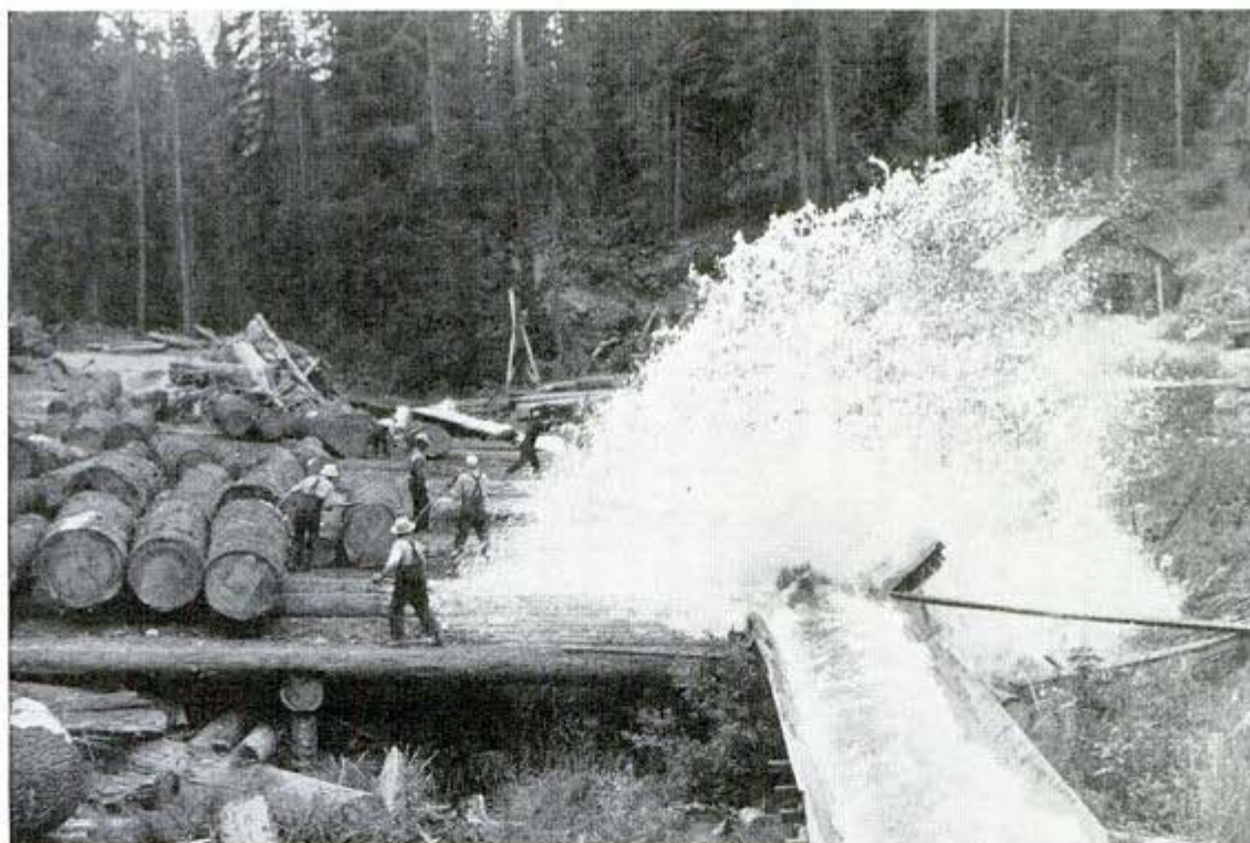
Into the flume goes a big timber as the crews prepare for the start of a drive down the river; the logs are carried in this manner to the deep, roaring water for the trip downstream to the sawmill
