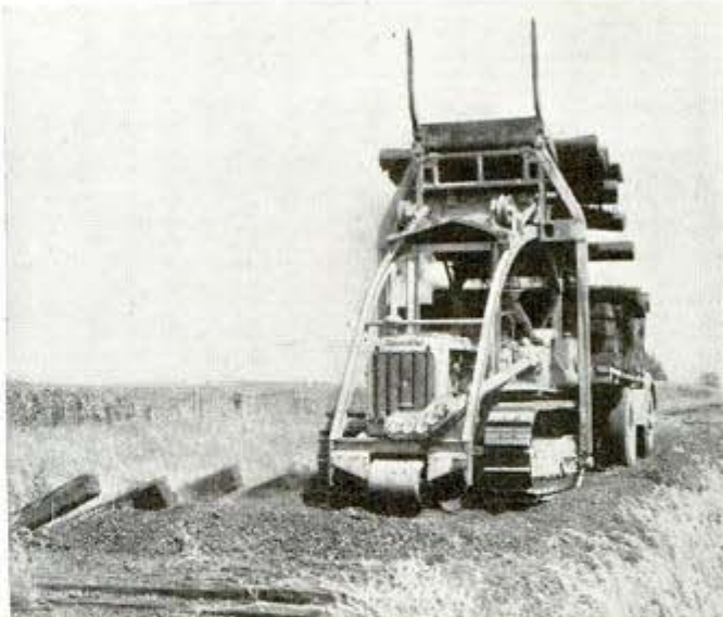
Caterpillar Diesel uprooting and salvaging ties from a 60-mile abandoned railroad, loading ties into truck at rear. Below, an Elwell-Parker loading truck carries a pipe into a boxcar
