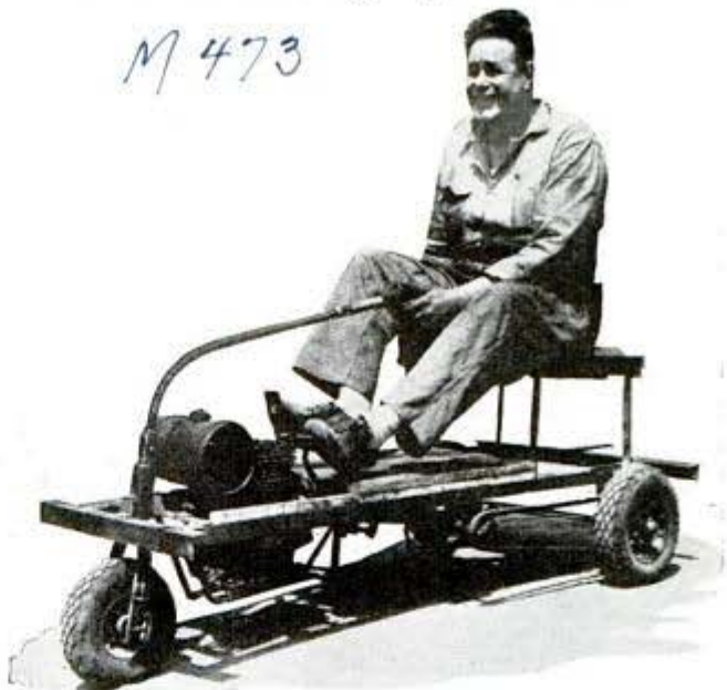
Homemade car travels 40 to 50 miles on gallon of gasoline
