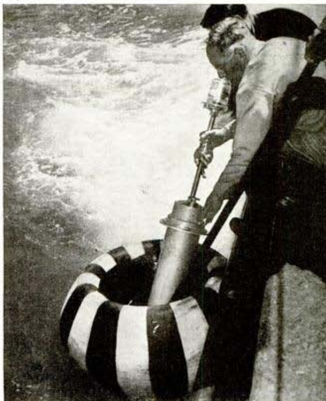
Photo from Westinghouse Radio controls lights in "doughnut" buoy marking seaplane base
