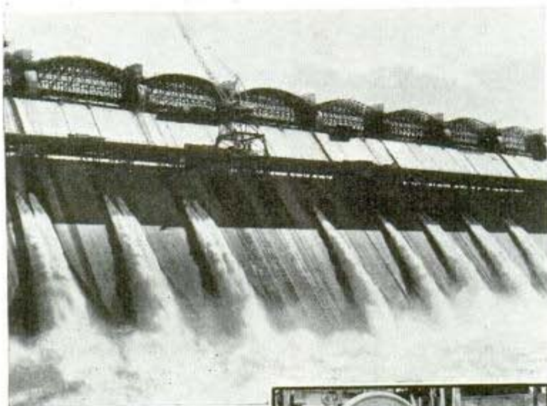
Floodwaters flow through Grand Coulee dam while work is progressing on the overflow spillway
