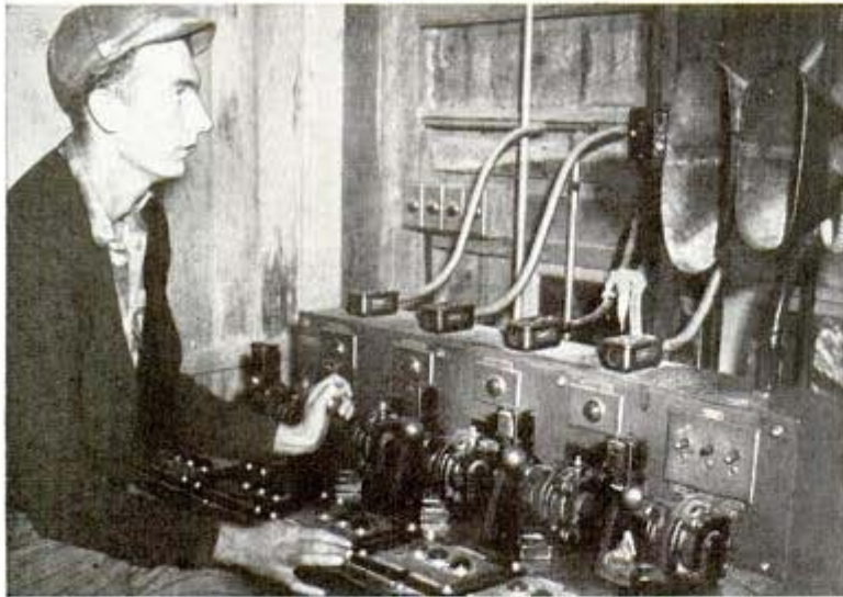
From this control table, concrete ingredients are weighed for the mixers
