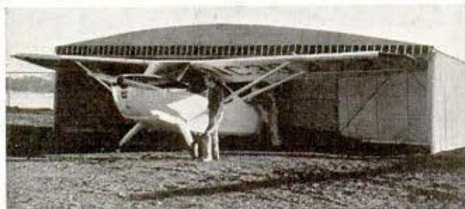
Top, a metal-clad Luscombe lightplane makes a front-yard landing. Center, a Piper Cub tandem trainer. The canvas hanger below, with steel frame and roll-up door, can be erected in five hours
