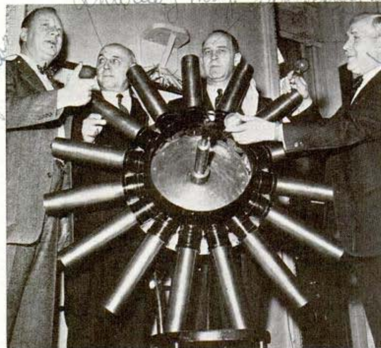
Spinning beneath an airplane, this bomb thrower could hurl 5,000 bombs a minute. Inventor, right, shows thrower to House and Senate members
