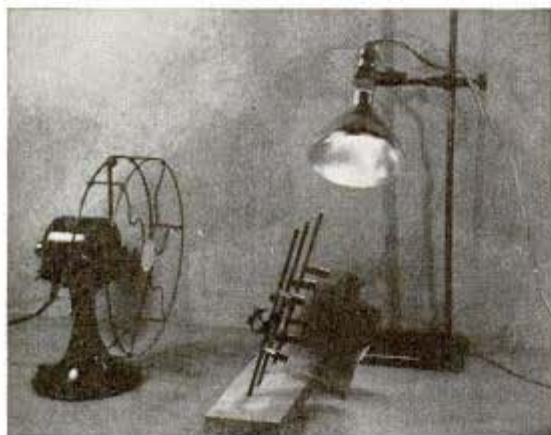
Drying photographic films with 250-watt lamp. The fan speeds drying and prevents damage to emulsion
