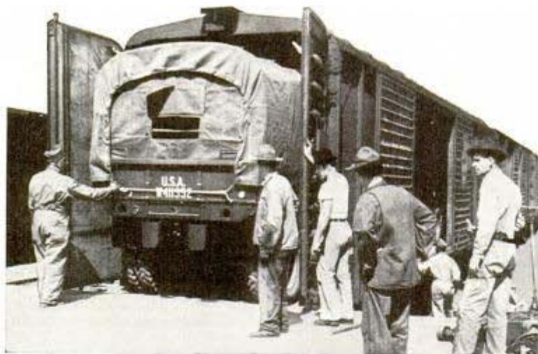
The railroads supply end-loading box cars to accommodate army trucks
