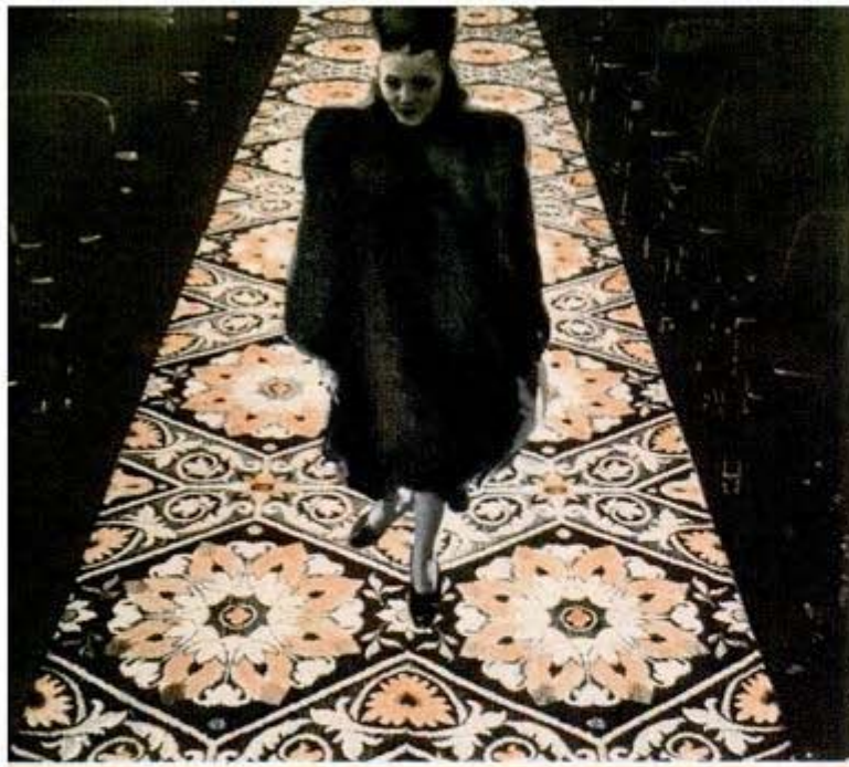
Carpet treated with fluorescent solution glows with eerie brilliance under ultra-violet radiations. Black-light lamps are concealed on each side
