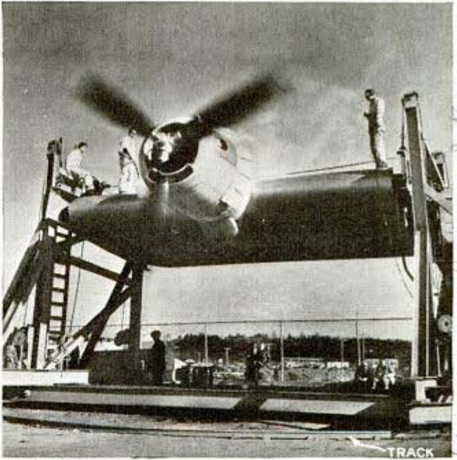
Rotating stand for testing engine, above, rolls on a circular track. Left, the "flight crew" is watching result of a test
