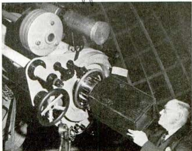
Installing camera box at focus of large refracting telescope
