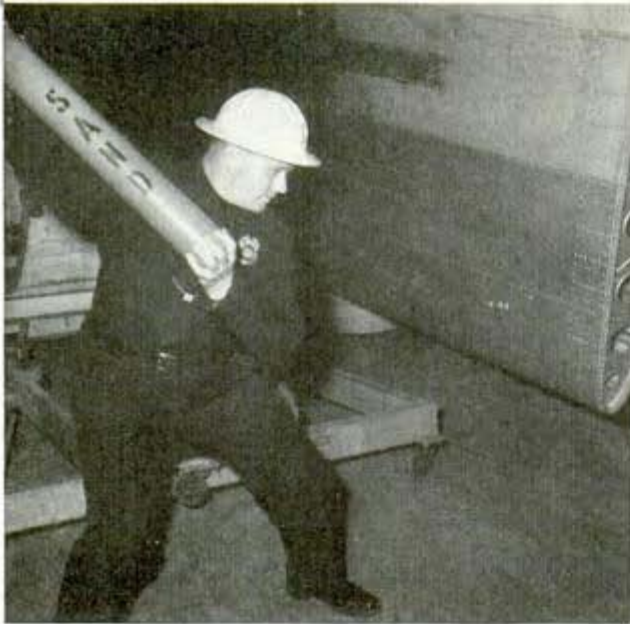
Demonstrating how sand is thrown out of tube to blanket fire like that of burning magnesium
