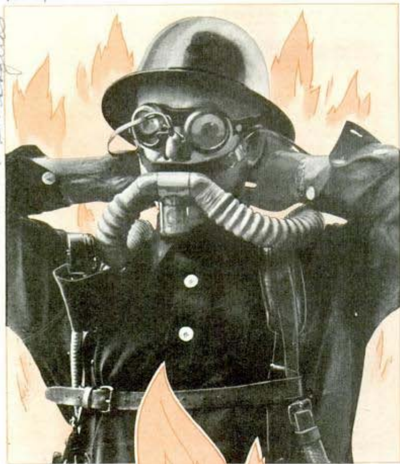
Fireman adjusting self-contained oxygen apparatus as protection from dangerous fumes at industrial fire
