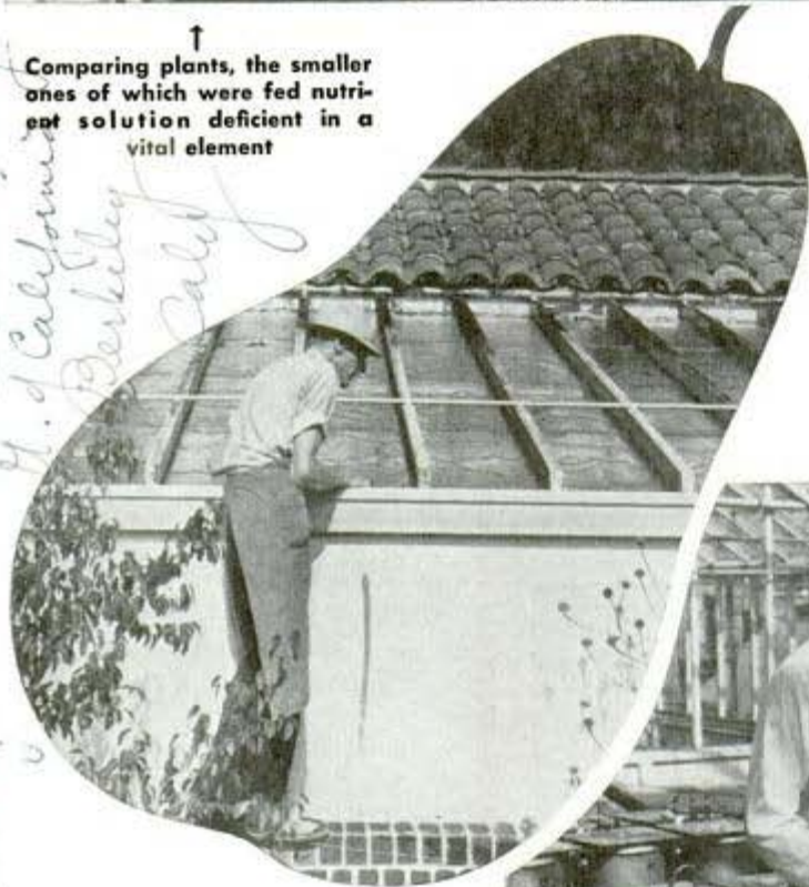
↑ Water curtain on glass roof admits sunlight to growing plants but excludes heat
