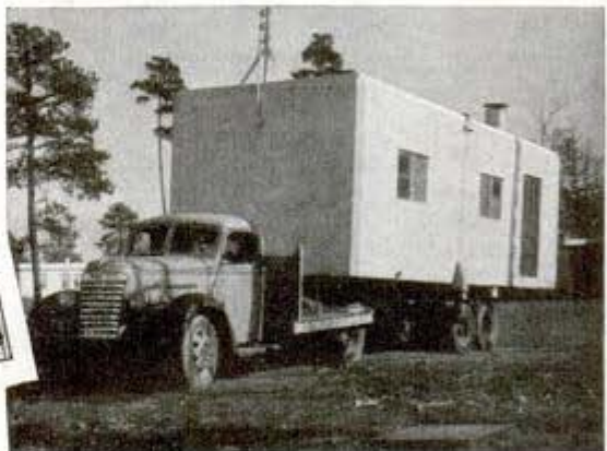
At lower right a truck hauls the ready-built house to its site, where a crane lifts it to concrete foundation piers (top). At far end of living room (lower left) is kitchen unit and doors to bedroom and bathroom
