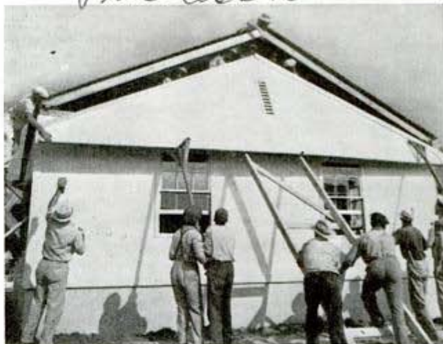
Four trucks, above, moving dismantled house from one site to another. Right, group of men removing one of the gable ends of the house; bottom, house rebuilt at new site and needing only a few finishing touches
