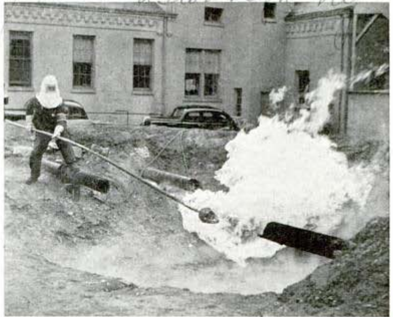
Plugging a broken gas main in a "dress rehearsal" for air raid
