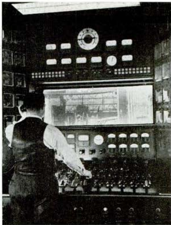
Engineer in control room of laboratory has at his fingertips 150 knobs, buttons and dials to regulate power creation and flow
