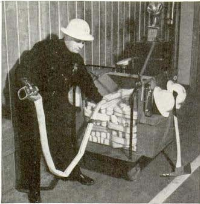
Portable fire-fighting equipment of type used in airplane factory
