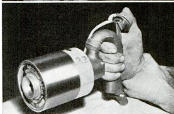
Magnetic hammer (bottom) does away with helper shown at top
