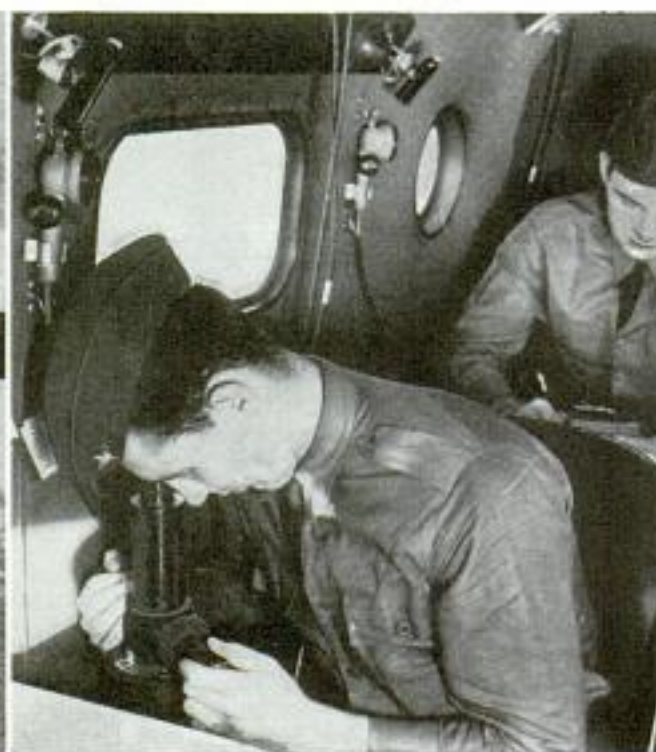
Sighting with drift indicator in flying classroom
