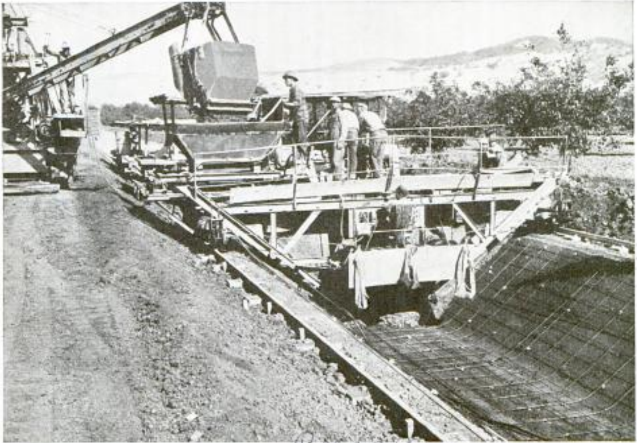
Mechanical concrete spreader straddles canal as it lays concrete bed and trowels it to smooth finish
