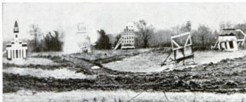
Cardboard buildings being blown up in breaking ground for factory site
