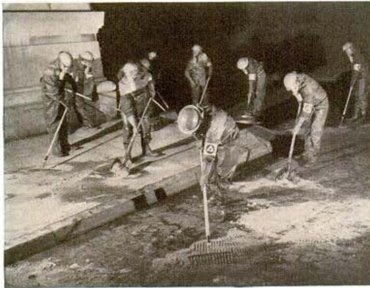
← Volunteer decontamination squad neutralizes a gassed area with sand and chloride of lime
