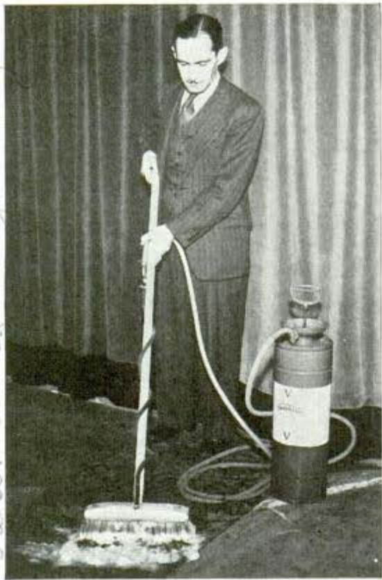
Tank at right has pump to force suds through brush
