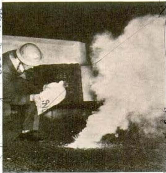
Holding a sandbag in front of his face for protection, a civilian fireman drops it on an incendiary bomb. This should smother it in two minutes
