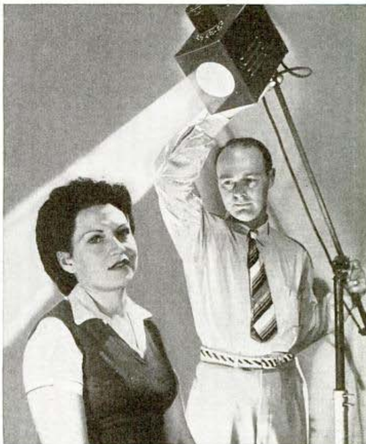
Homemade spotlight has a built-in fan to keep the powerful bulb cool and thus prolong its life
