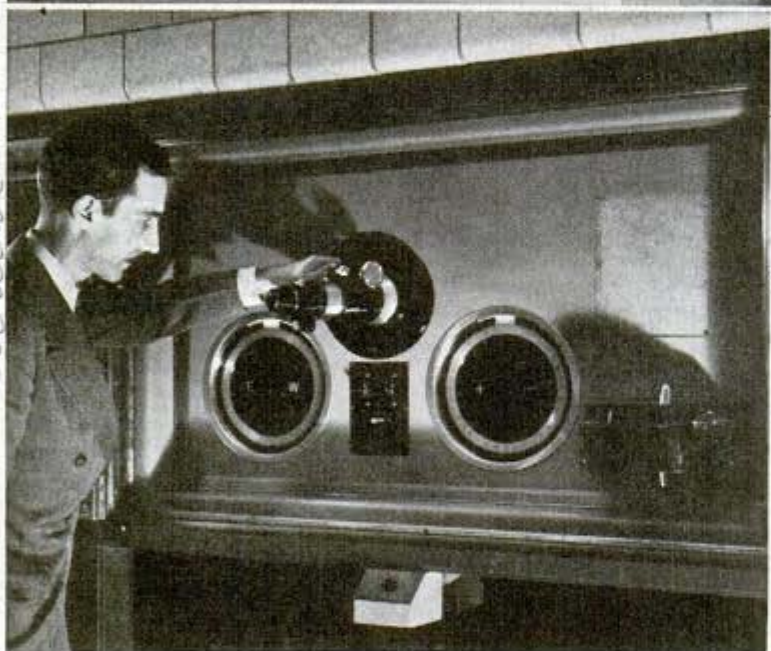
↑ Mirror, center, may be turned to bend ray from any star into ten-inch lens of telescope ← "Seeing end" of telescope. Dials, left and right of eyepiece, control movement of mirror
