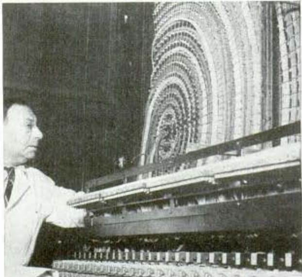
Behind the strip map of a flight recorder is this bewildering maze of electrical wiring
