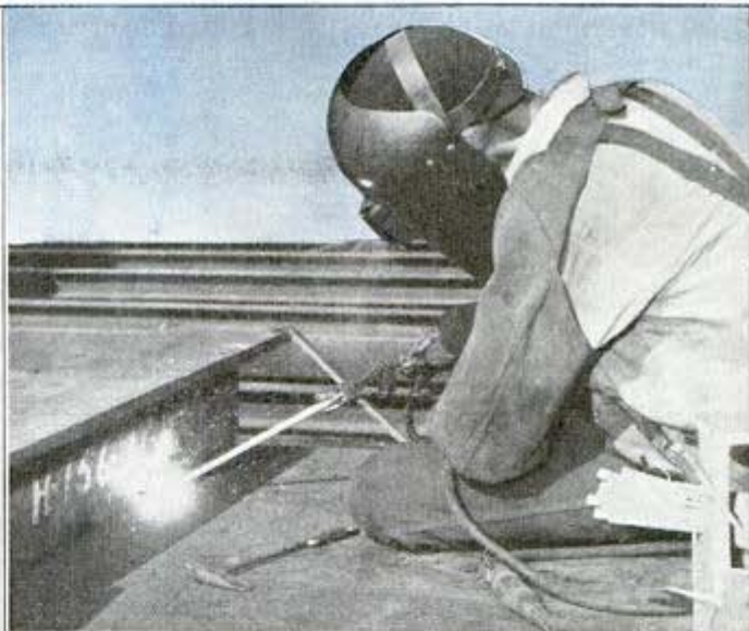
Above, a welder assembles a prefabricated part of a ship. Left, a crane moves a prefabricated section into position
