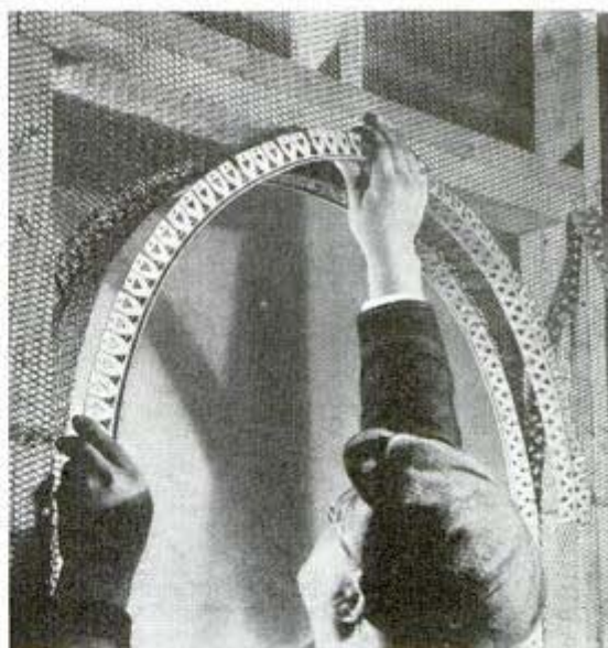
Fitting plaster bead over doorway to form an arch
