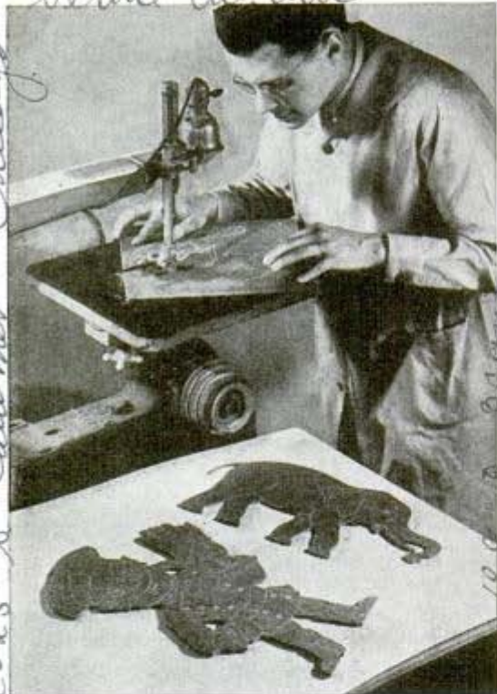
Sawing figure from plastic sheet requires only care in following the outline. Foreground, two samples
