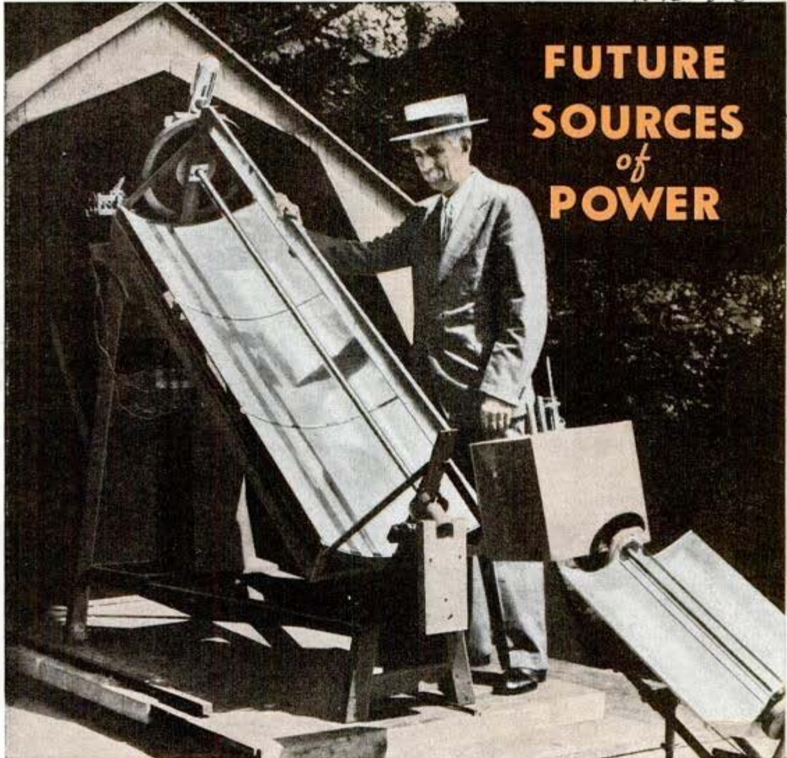
Dr. Charles G. Abbot of Smithsonian Institution standing beside flash boiler—a solar power plant. In foreground is toy cooker in which tiny cakes can be baked. Mirrors concentrate sun's rays
