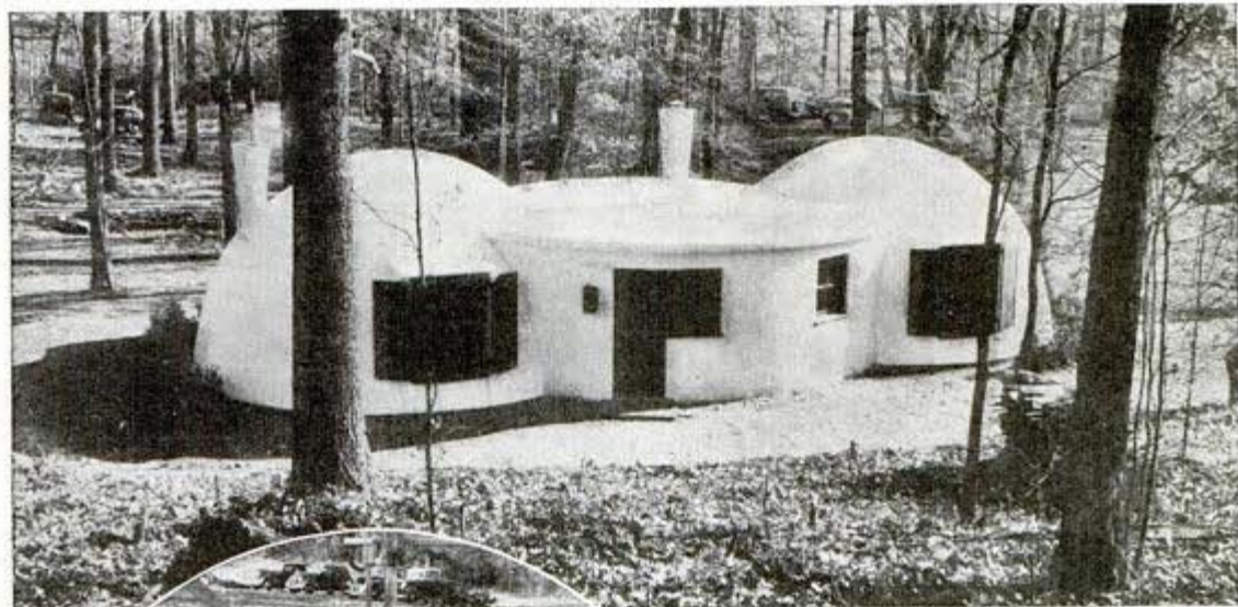
At Falls Church, Va., a colony of unique concrete igloos offers economical housing for war-industry workers. One hemisphere contains two bedrooms, the other a living room; between is an entrance hall, bath and kitchen
