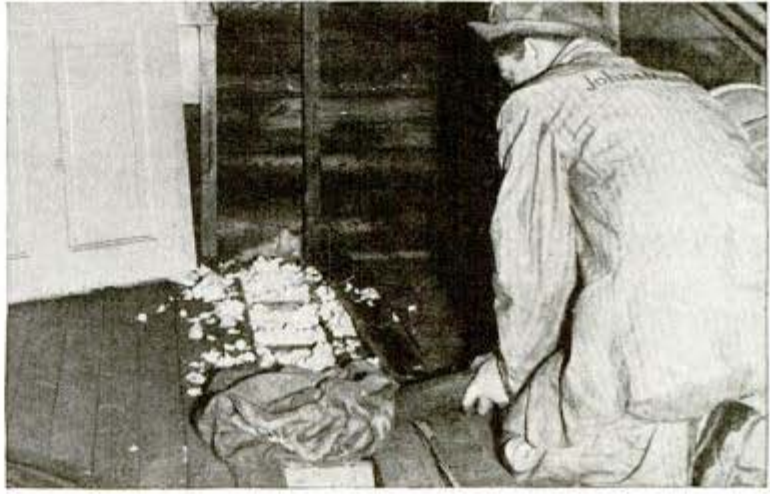
Proper insulation of attic will save the average dweller as much as 71.4 percent of all the heat escaping through roof of house
