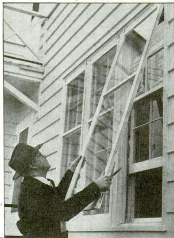
Putting storm windows on your house will save as much as 63.8 percent of the heat escaping through windows. Below, taking temperatures at floor and at the ceiling. Differences exceeding four degrees indicate inefficient heating
