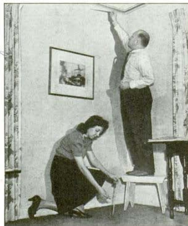
Putting storm windows on your house will save as much as 63.8 percent of the heat escaping through windows. Below, taking temperatures at floor and at the ceiling. Differences exceeding four degrees indicate inefficient heating
