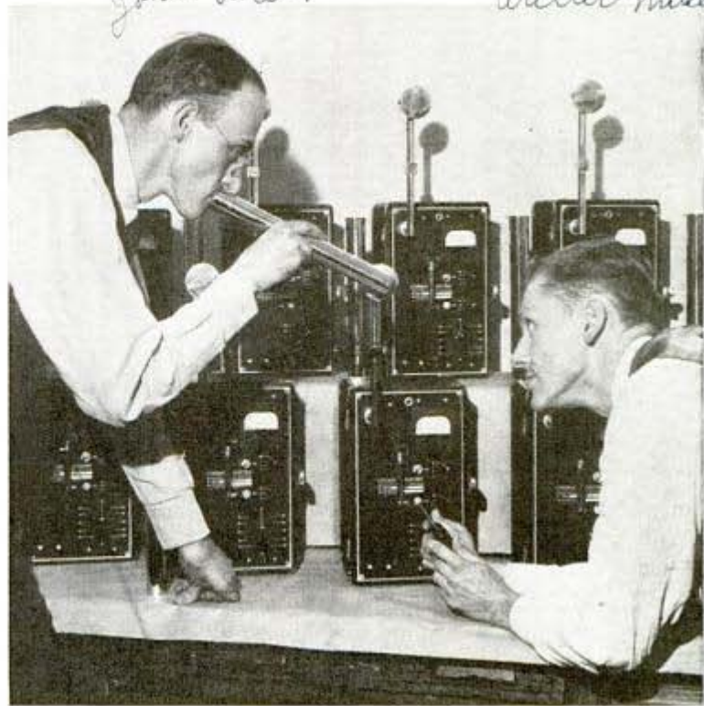
One blows the whistle while another adjusts sensitivity of "noise" meter
