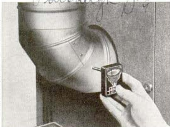
Gauge checking amount of draft in furnace elbow
