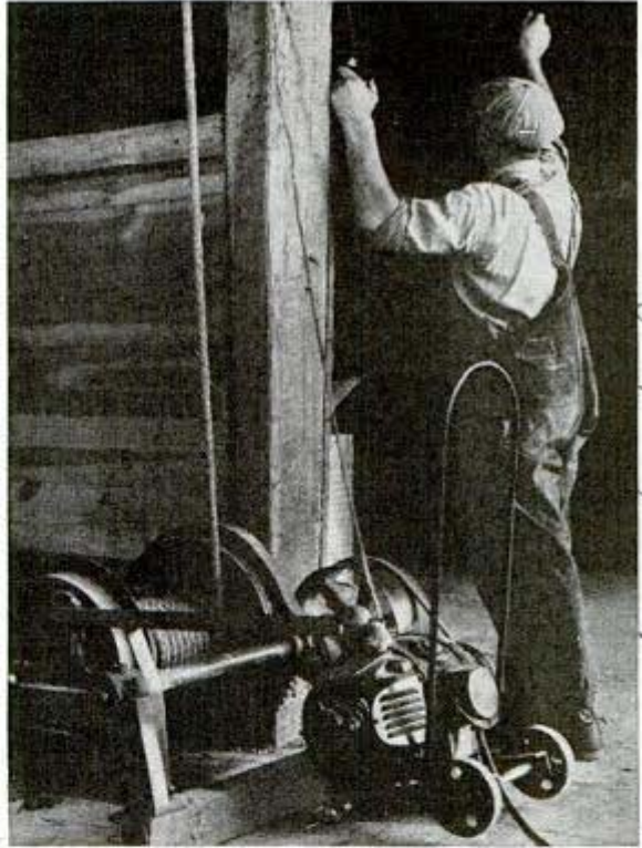
Here the portable motor does the lifting, enabling one man to handle the hay (Westinghouse photo)
