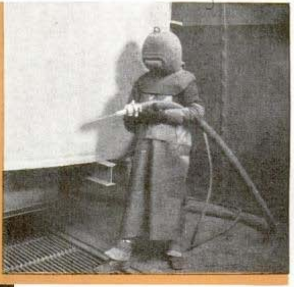
Helmet, apron, shin guards, gloves and steel-capped shoes protect a sand blaster
