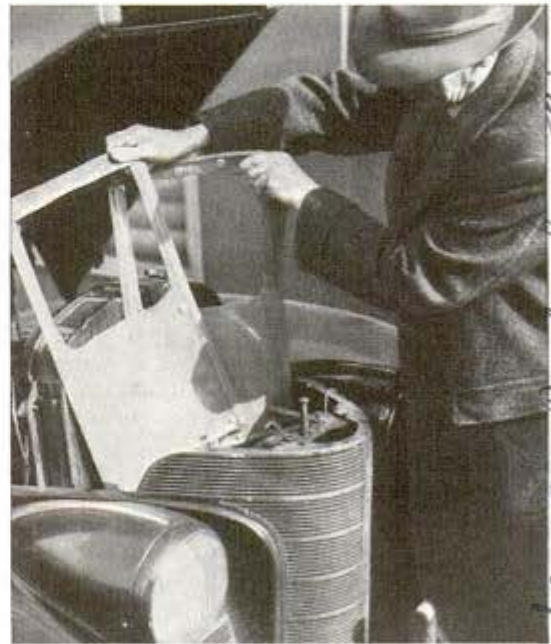
Two-piece winter front adjusts to fit car radiator
