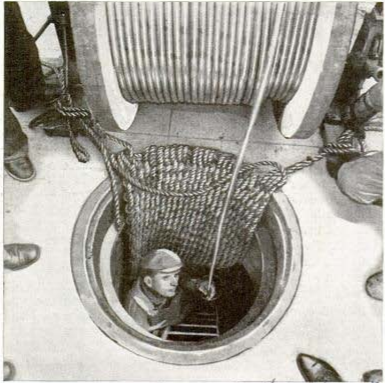
Unwinding from its spool, a new coaxial cable starts underground
