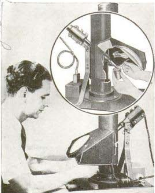
Soldering jobs handled under magnifier as in circle
