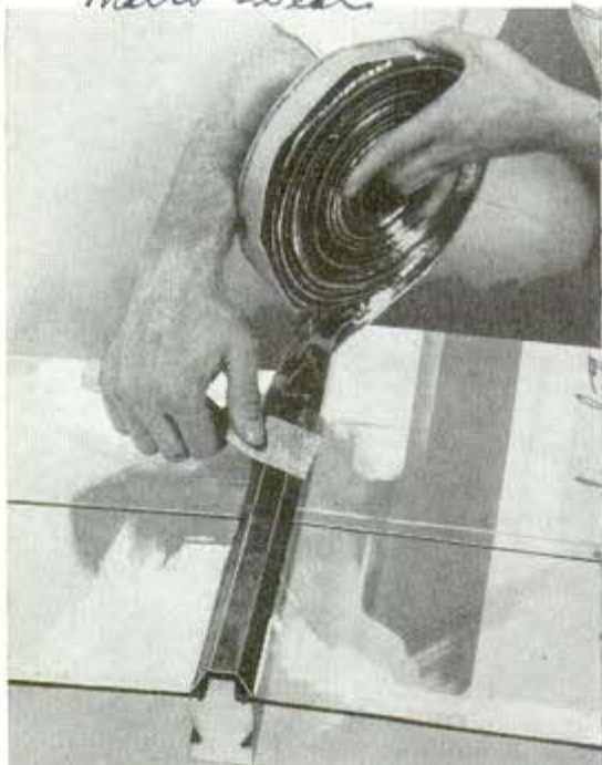
Glazing tape unrolls as it is applied to window
