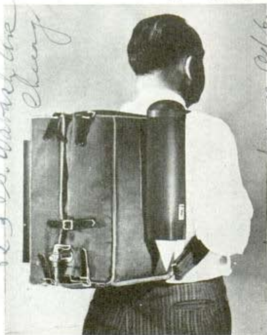
Jacket insulates water tank as it makes the rounds
