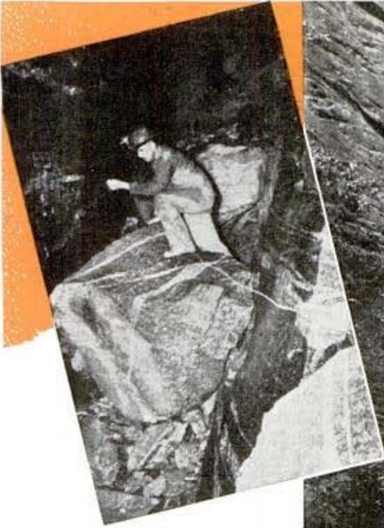
↑ Stringing telephone cable in a cave in Bald Mountain, N. C.
