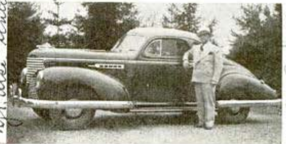
Side bumpers guard fenders and wheels from scrapes
