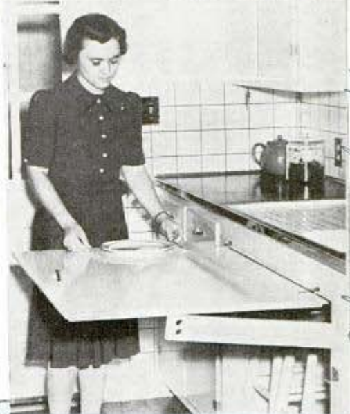
→ Drainboard has a portion of the side on hinges so it can be pulled out and rested on wooden arms
