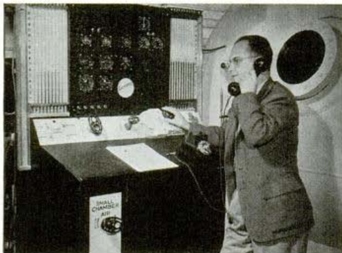
Outside control panel for altitude chambers with operator talking to pilot inside. One chamber also is connected to the cold room
