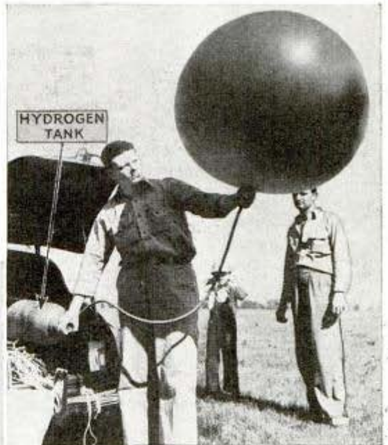
Two methods used by amateur radio operators for erecting emergency antennas. Above, inflating balloon with hydrogen, and, left, sending up kite attached to spool mounted on auto wheel
