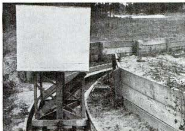
Above, the target carriage rounds a bend in the track, which is three feet wide and a foot deep. The wooden parapet, rising 40 inches above bottom of track, hides carriage from view of gunner
