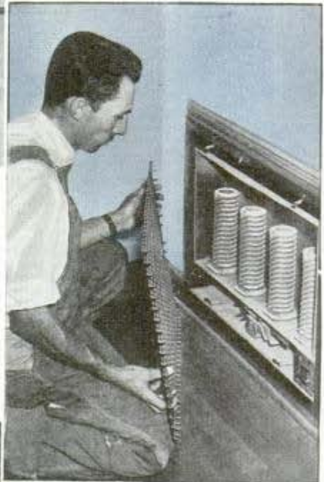
Nailing asbestos siding over plywood on home in "smokeless community" Meadow Hills Automatic electric heating unit being installed in a Fonde-built home ↓
