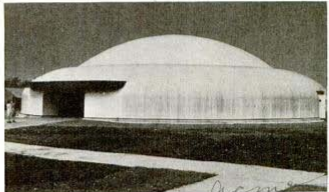
No beams or supports are needed in this shell-like structure
