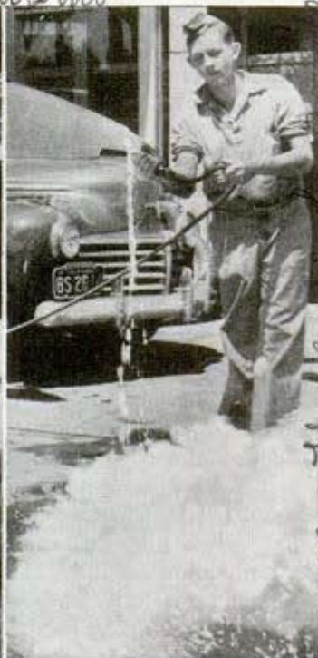
Powder (left) quells magnesium fire but water spreads flames
