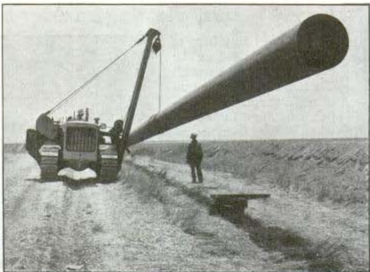
A Caterpillar tractor gently drops the huge pipe into trench
