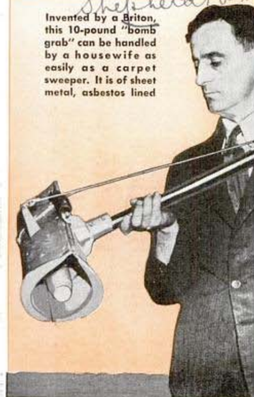
Thousands of these long-handled snuffers are spotted around English cities to fight incendiary bombs, which burn out under the asbestos dome. Below, control room of London's civil defense organization from which fire fighting and rescue work are directed
