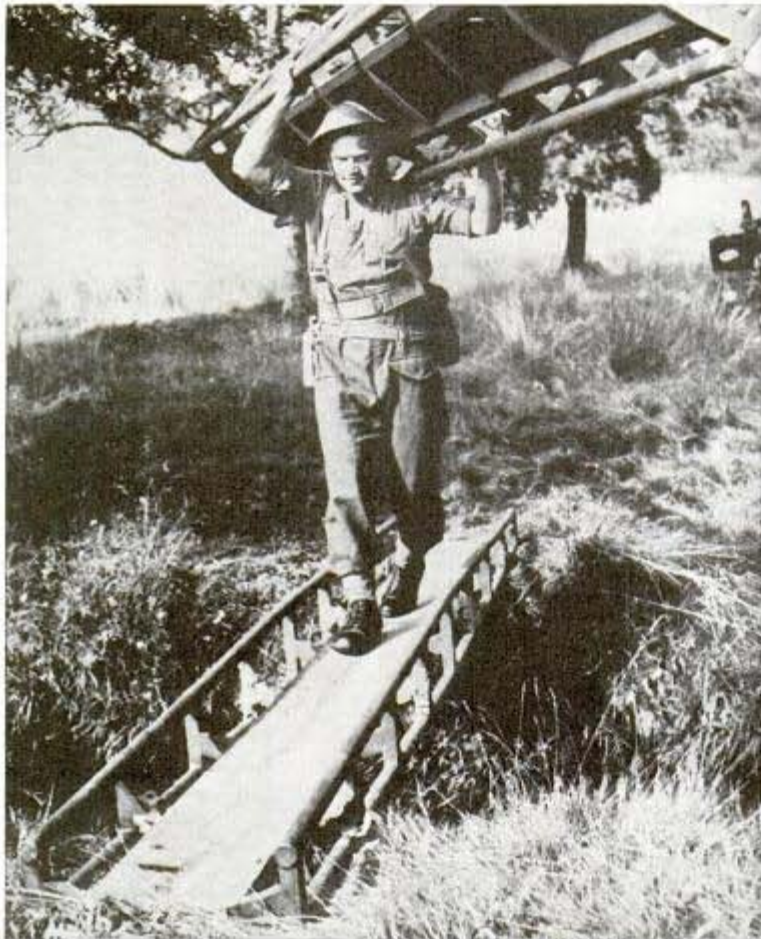
Soldier carries bridge section overhead as he crosses ditch on another
