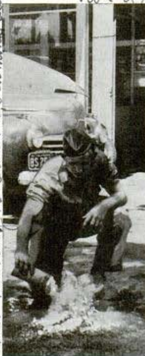
Powder (left) quells magnesium fire but water spreads flames
