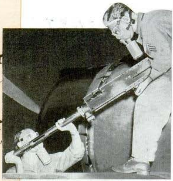
Mechanics wearing gas masks as they install .50-caliber machine gun on pursuit plane
