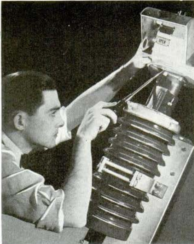
Circuit breaker recloses circuit five seconds after shut-off
