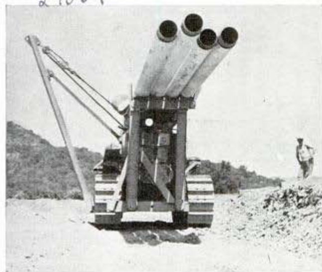
Tractor carries five tons of pipe on top of special rigging.
