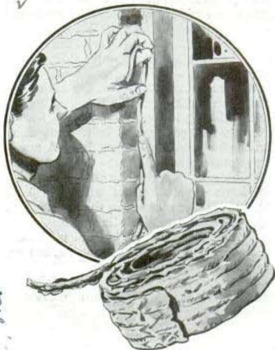
The calking cord is pressed in place with a finger
