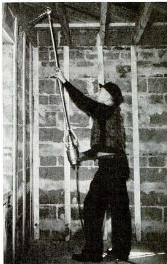
Extension drills at angle in places hard to reach
