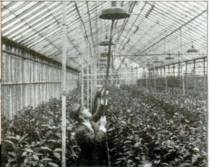
Attendant replaces light bulb in a greenhouse fully equipped with rows of growth-promoting lights
