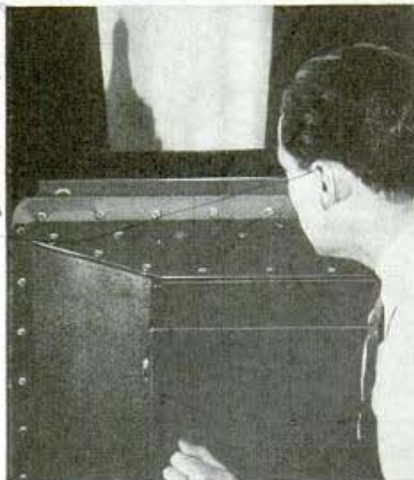
← View finder on giant camera pointed at Empire State Building lightning rod is a rectangle cut in wooden mask which replaces top panel of office building window
