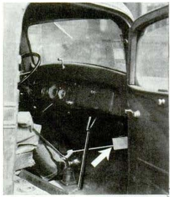
Extension on gear lever stops idling in neutral
