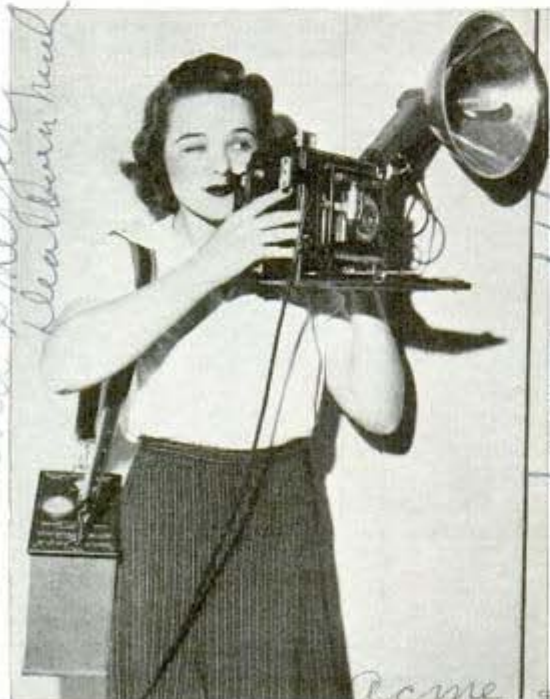
Super-speed lamp "freezes" action at 1/20,000 second
