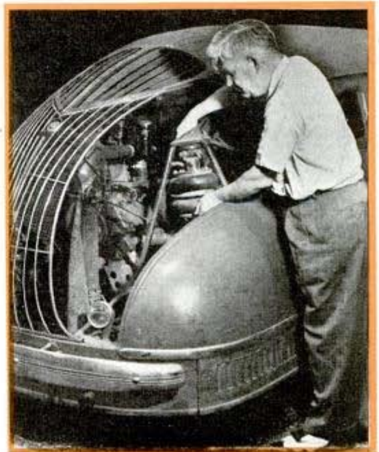
Adjusting rubber springs which also serve as shock absorbers on the Stout car
