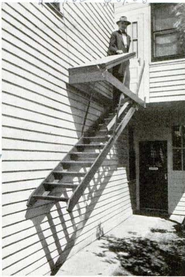
Stairway is counterbalanced by sliding weight in hinged cover
