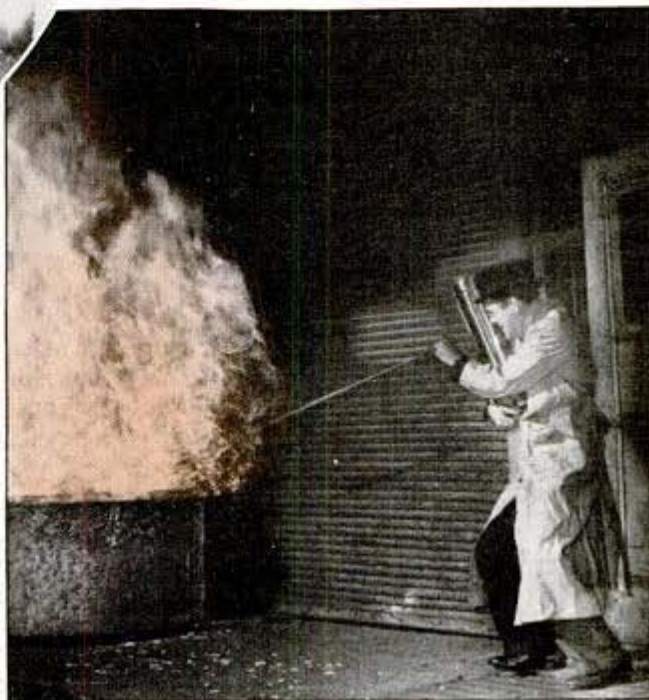
Two and one-half gallon foam extinguisher putting out a gasoline fire in Underwriters Laboratories
