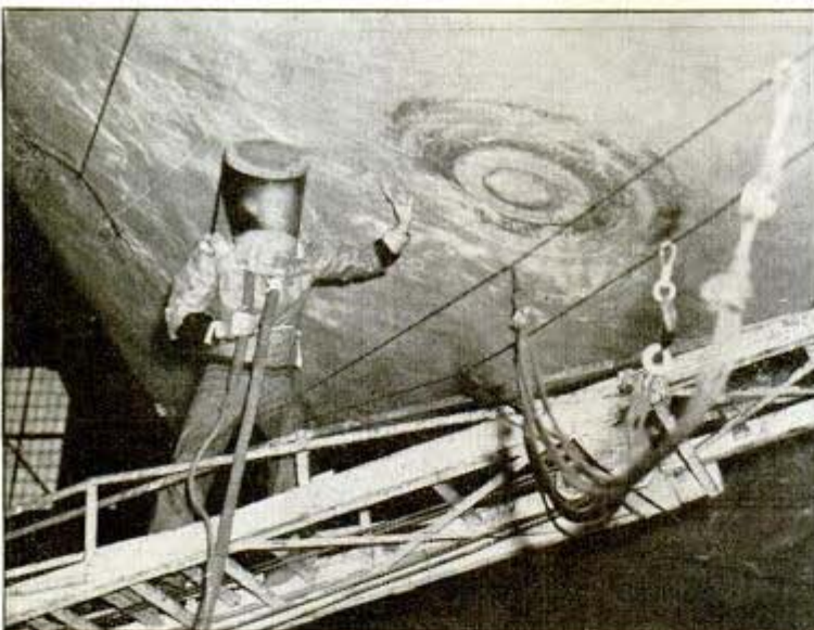
↑ Inspecting blimp calls for man in gas mask to enter the big envelope in search of leaks and weak places in the bag
