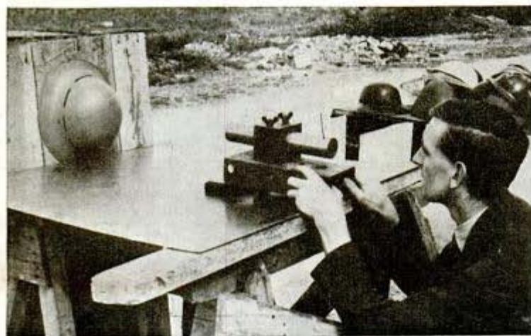
Gunner firing steel balls at helmet tests its ability to shed shrapnel fragments with safety
