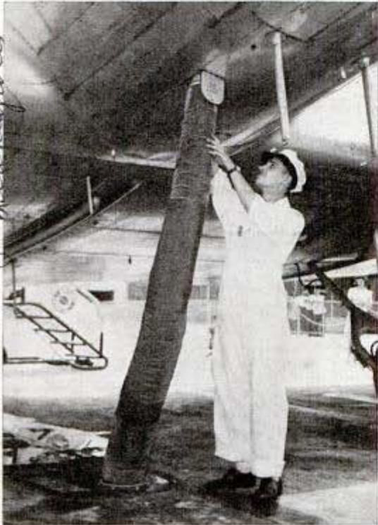
Tube from underground duct blows air into plane
