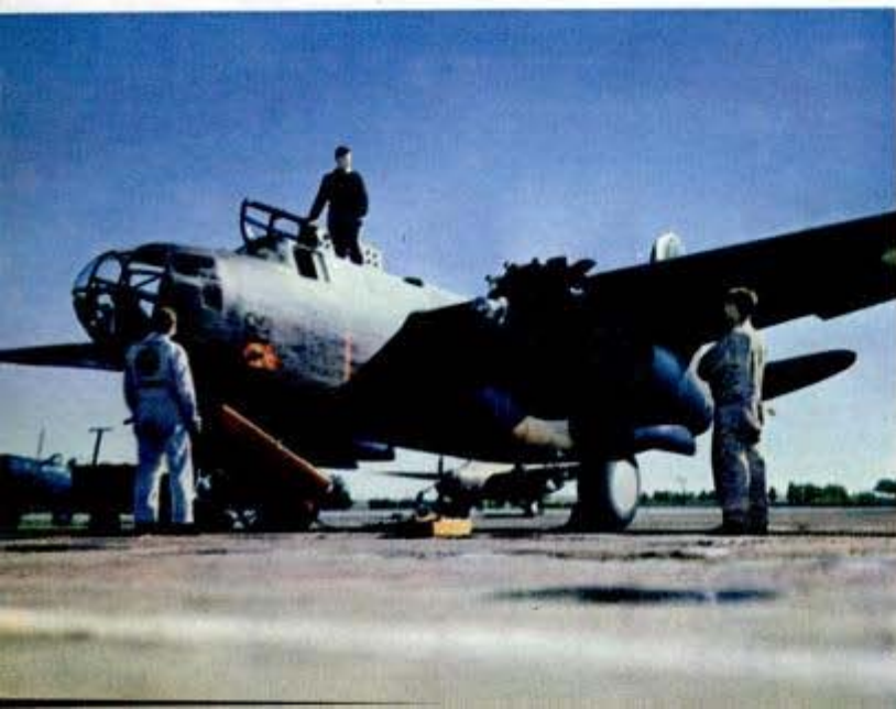
Below, natural color photograph of a Douglas DB-7B undergoing a test run of the engines near plant
