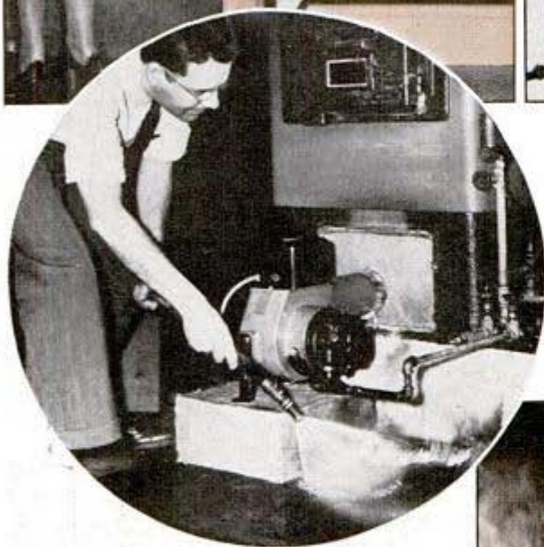
← Fine spray from hose cools and quickly kills oil fire around furnace; heavy stream would spread flames
