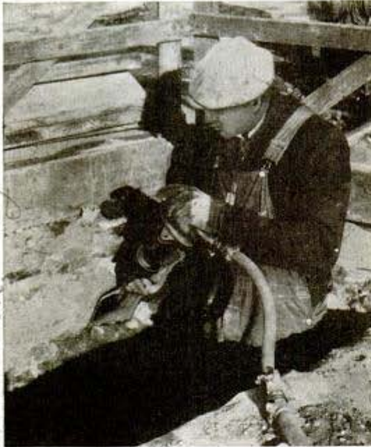
Air pressure drives the small spade into hard clay
