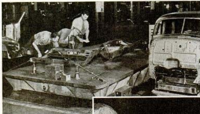
← Checking the frame of an automobile on the 8 by 18-foot steel platform, where the slightest inaccuracy can be detected
