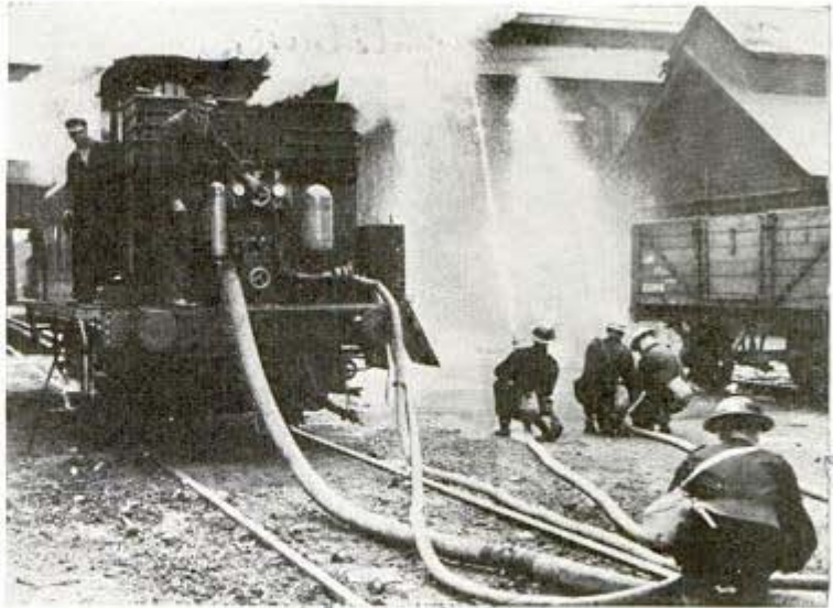
Pumps on fire-fighting locomotive deliver a ton of water per minute
