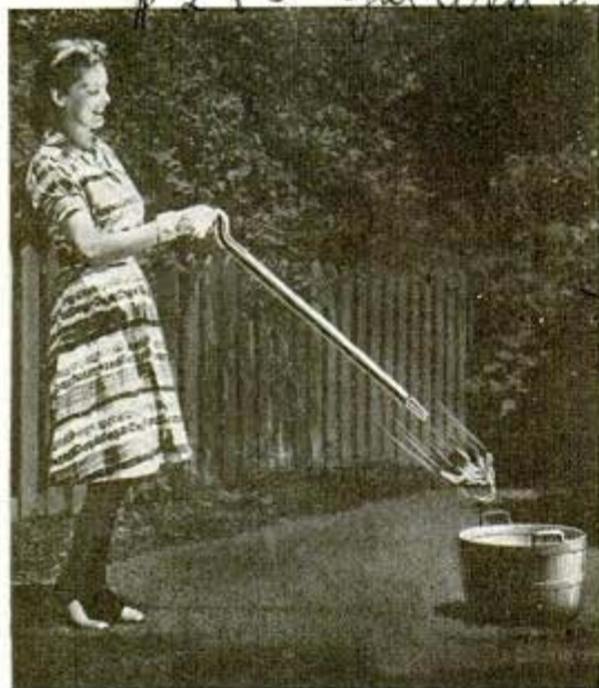
Uprooted weed is shot into gardener's basket when trigger in handle is pressed to release the spring
