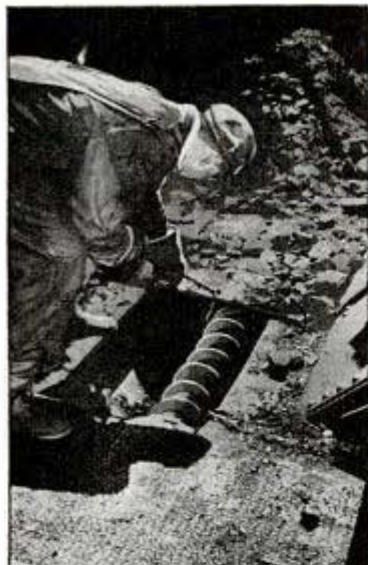
This powerful stoker screw delivers coal to firebox
