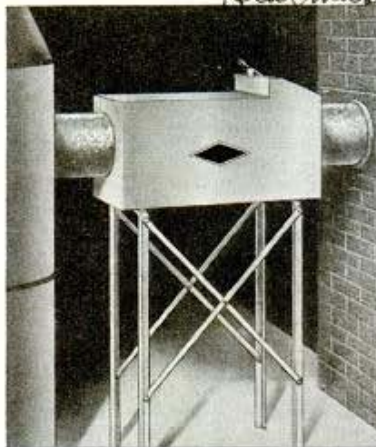
The photo at left shows a fuel saver installed between the furnace and chimney, while the diagram at right indicates the flow of air and gases
