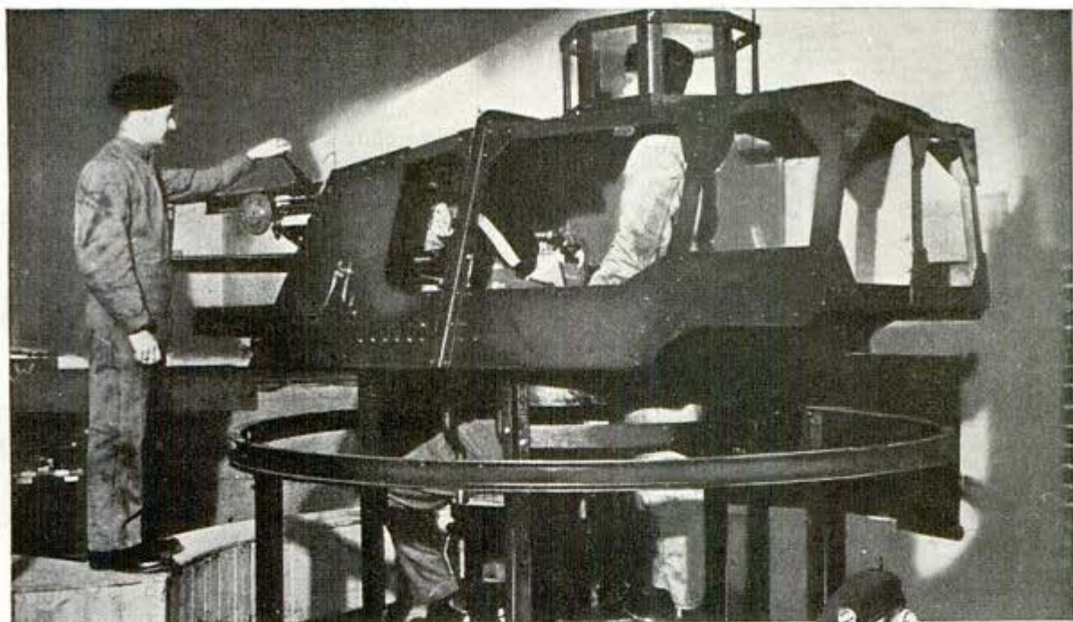
Above, pupil in fastest Rypa machine that pitches and lurches like a real tank while he tries to keep on the target
