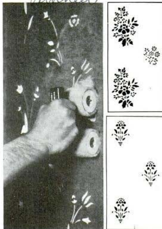
Left, using roller to paint designs on wall through stencil. Right, prints of two available patterns
