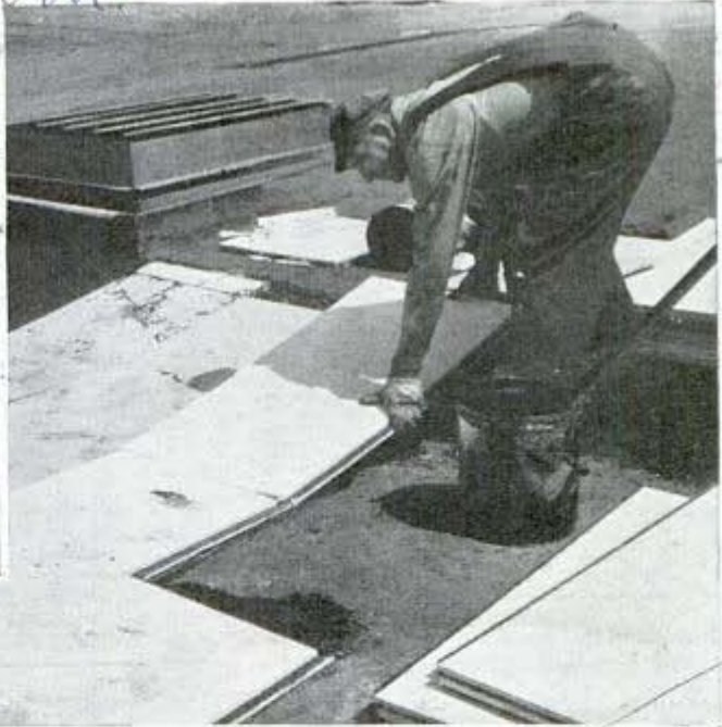
How shiplapped roof insulating board may be applied to a flat roof deck to seal out heat in summer and seal it in during winter. Below, sectional view of building showing typical uses of structural insulating board. Some applications are practical only for new houses
