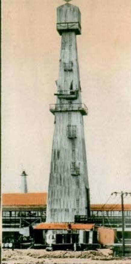
Left, well illuminated for drilling after dark. Right, Ford Motor Company well in California is distinguished by sheet metal covering on framework of the derrick
