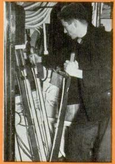
Loading a shell into deck gun of the navy's largest submarine, Kingston . Levers at right control valves for submerging or surfacing
