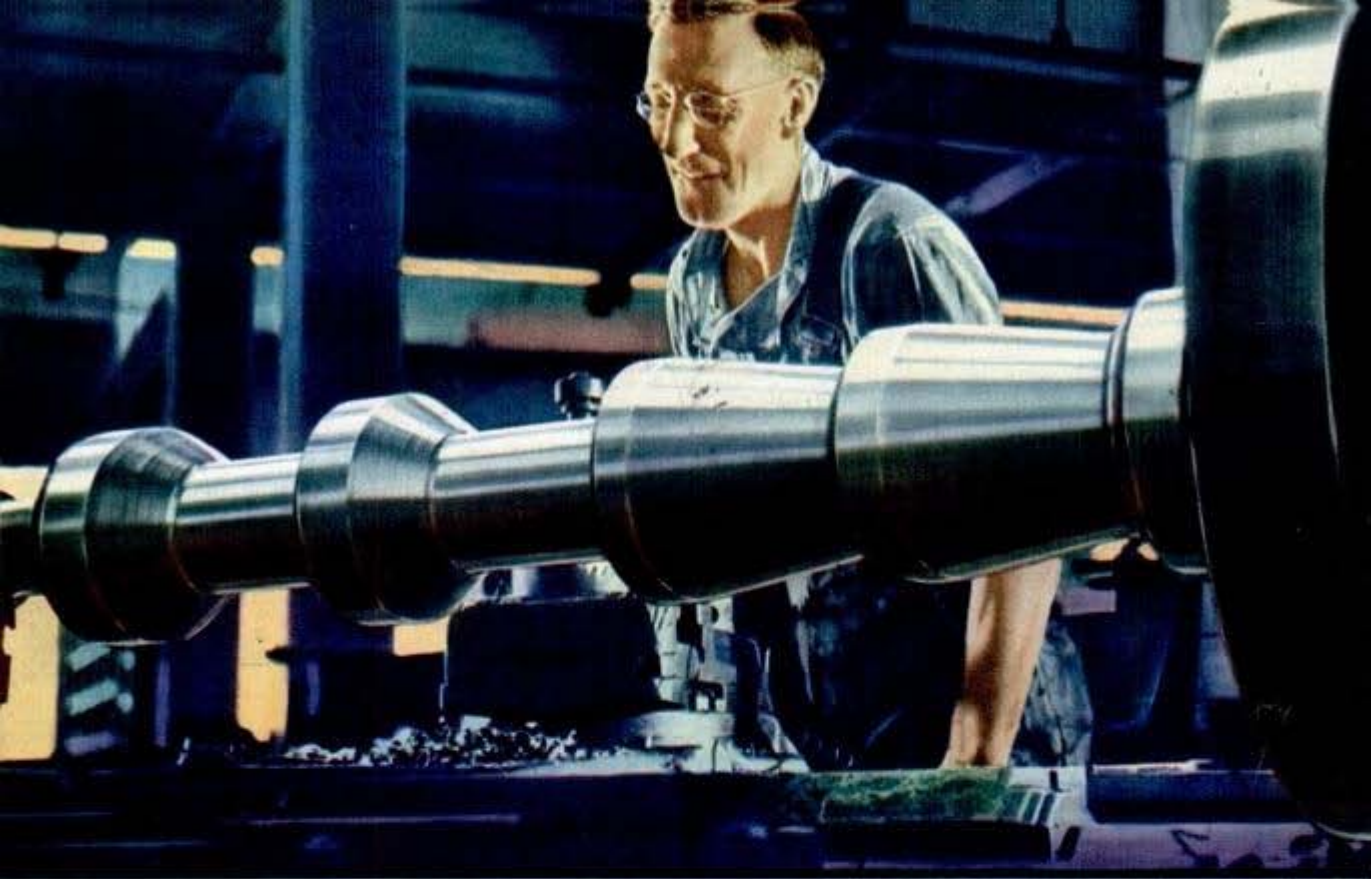
24 8106 Above, cutting valves for packer assembly used in testing or acidizing oil wells. Acidizing is one of the means employed to extract more oil from existing fields, the sand being treated to increase its porosity
