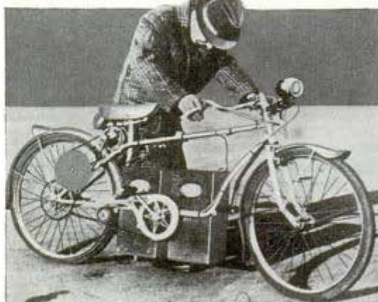
Two dry-cell batteries run this bike about 63 miles
