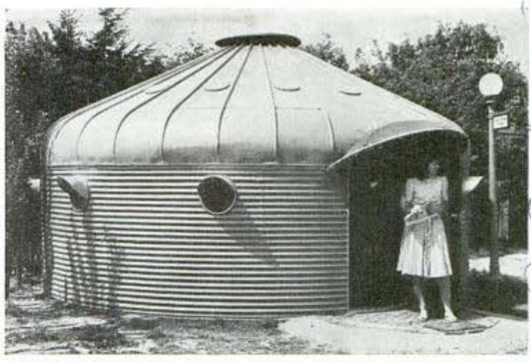
Steel house with "umbrella" roof is built of prefabricated steel panels, has ceiling skylights and porthole windows on sides
