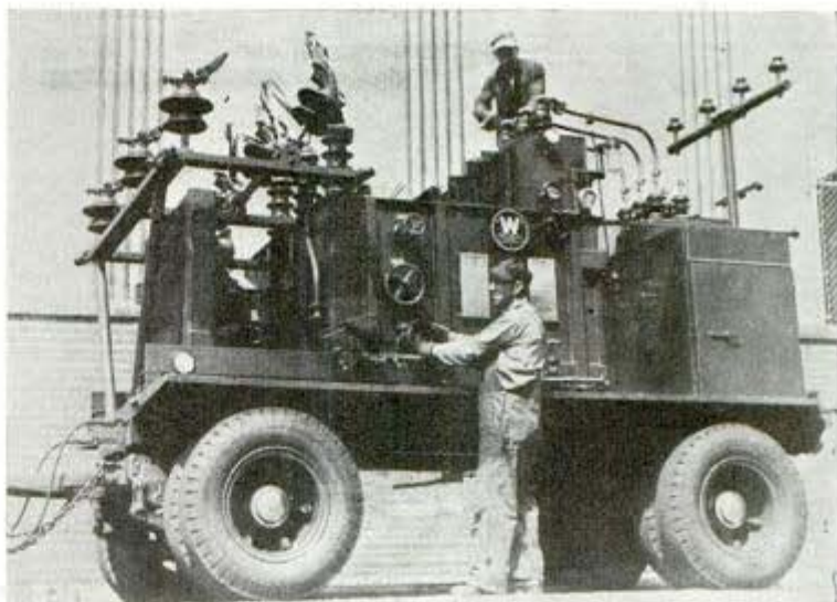
Portable substation, built by Westinghouse, helps keep power flowing
