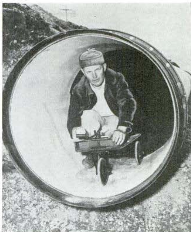
Pipe inspector eases his work with scooter pushed by foot
