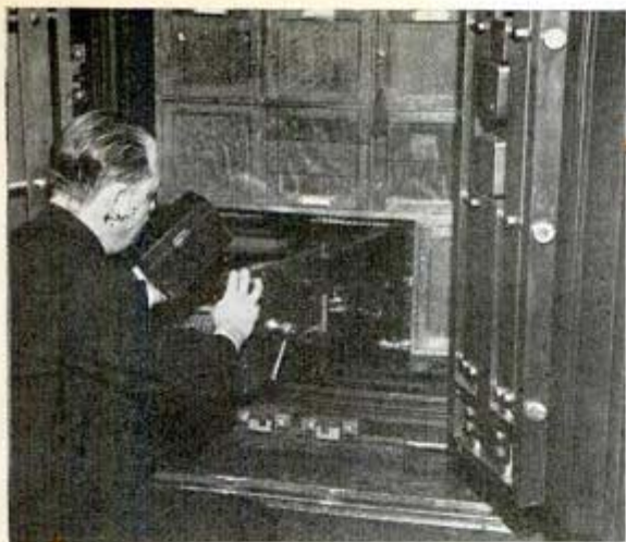
Left, vault in which the Vargas is kept has solid steel doors, each 16 inches thick and arranged in layers. It is protected by an electric alarm
