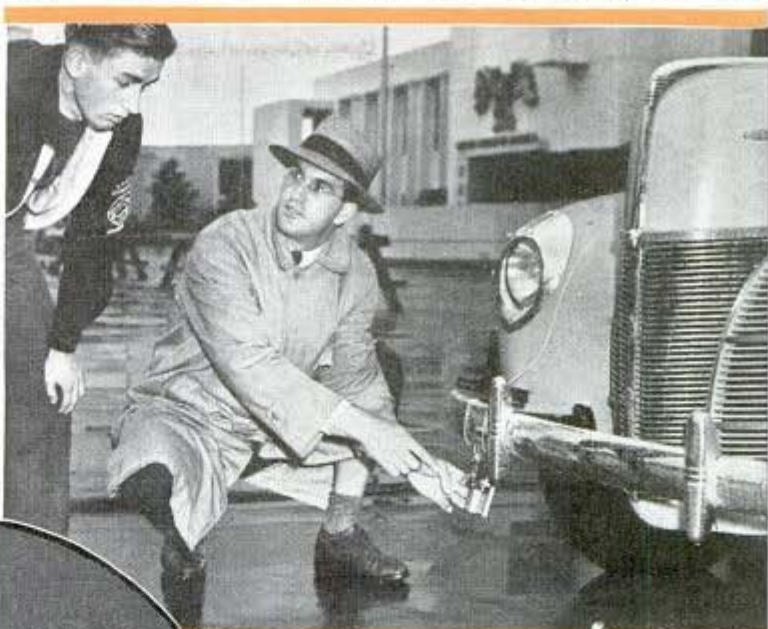
Observer points to detonator which he fires as car moves, signaling driver to stop. As brakes are applied, detonator fires again, then time for driver to react is measured
