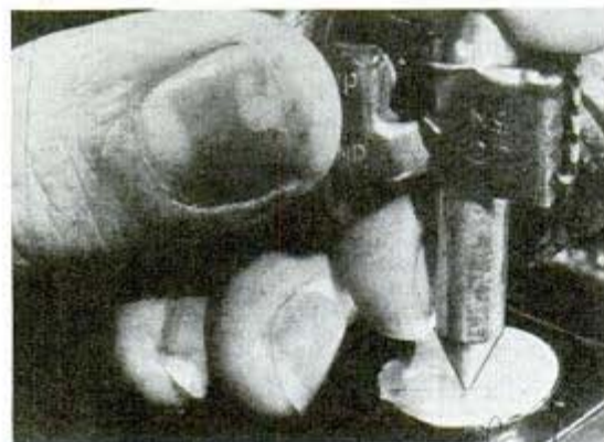
Spot-welding a filament 1/2,000 inch in diameter is so delicate a job it is done under magnifying glass
