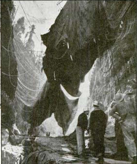
Above, 35,000 pounds of canvas and ropes, ready to be raised. Right, rigging is started on its way up. Bottom, tent nears first level. Note gutters on wall
