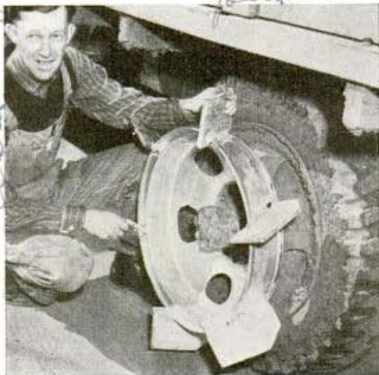
Rim equipped with paddles fits outside truck wheel
