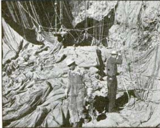
Above, 35,000 pounds of canvas and ropes, ready to be raised. Right, rigging is started on its way up. Bottom, tent nears first level. Note gutters on wall
