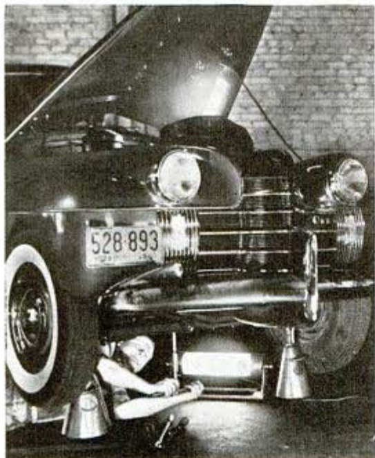
Tool tray carries fluorescent lamp under automobile
