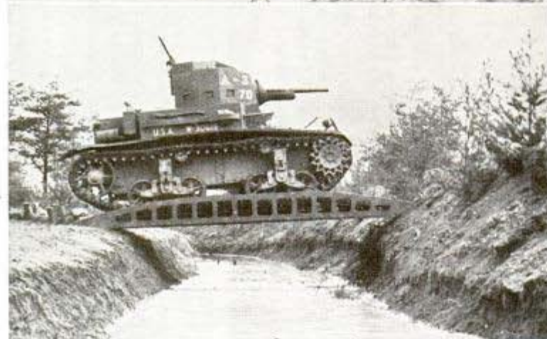
Knee-deep in water, army engineers at Fort Belvoir, Va., are shown at top erecting a new-type sheet-steel ramp which enables a tank to cross small streams. Bottom, the fabricated steel "bridge" is given a test
