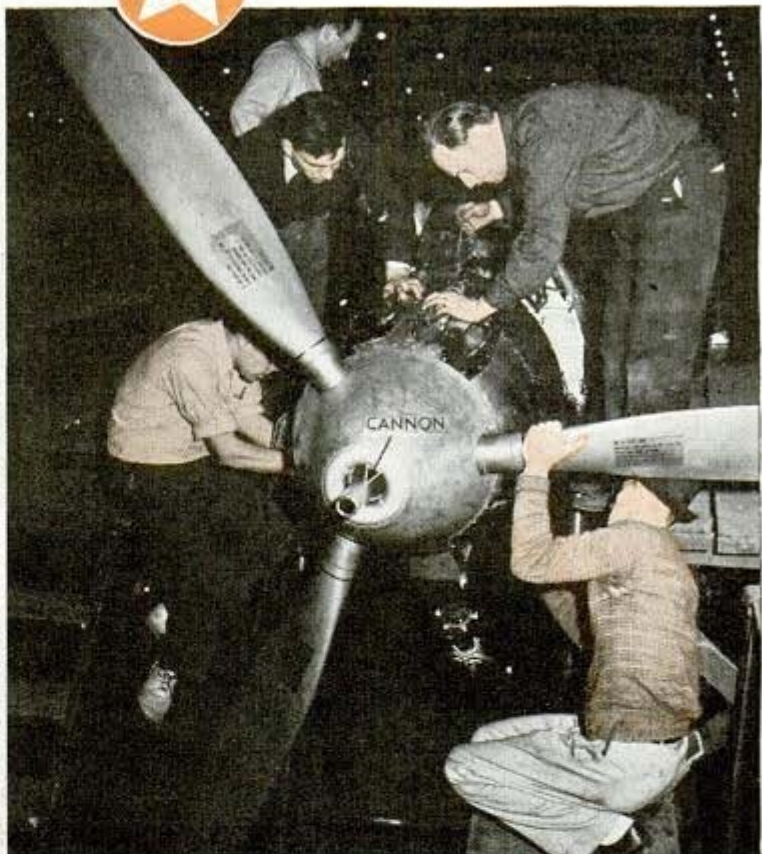
Servicing the Airacobra's armament, which includes a 37 mm. cannon that fires through the hollow hub of the propeller (see arrow) Below, comparing Airacobra's diving speed with speed of a bullet
