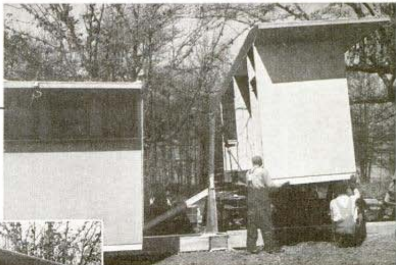
Prebuilt section being lowered from trailer, above, will be bolted to other sections already in place
