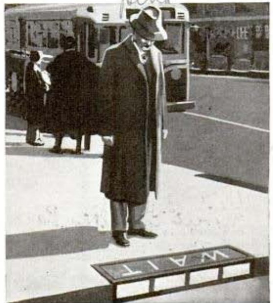
Here pedestrian halts at "wait" sign. When the word changes to "walk," he can cross intersection safely
