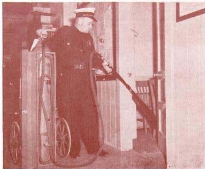
Below, demonstrating how to fight fire in office with carbon dioxide
