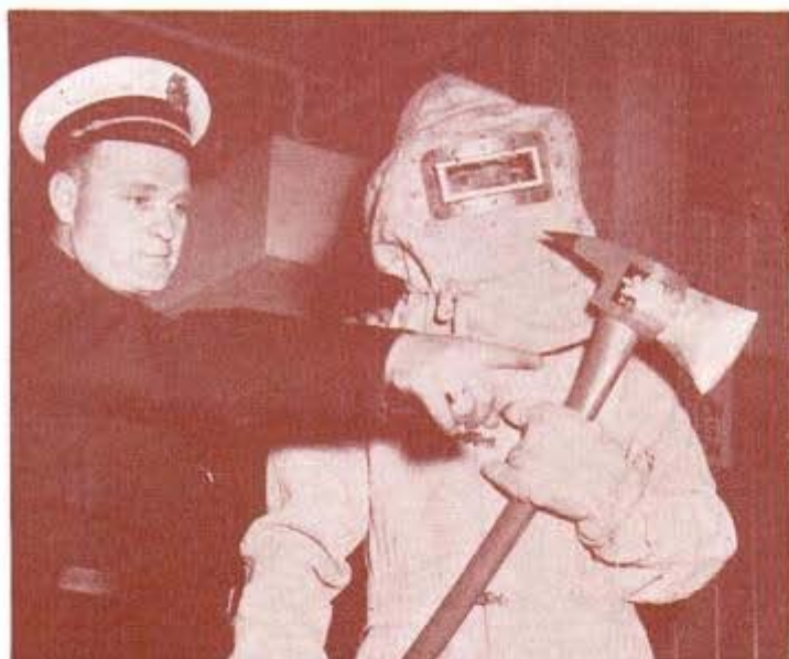
Above, fire chief instructing employe dressed in asbestos clothing
