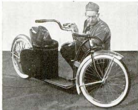
Motor-driven bicycle has auto seat and combination clutch and brake pedal in the floor
