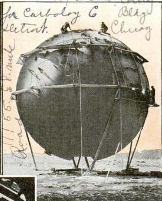
Above, sphere for storing hydrogen gas, fuel used in tool making
