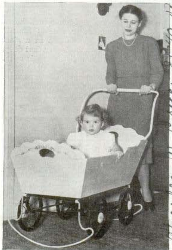
Rockers are lowered to use baby carriage as cradle
