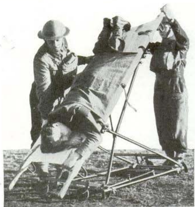
Stretcher on tilting cart rocks patient to restore breathing
