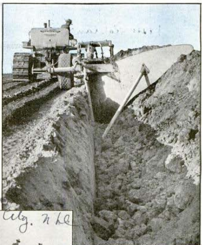
The big Diesel-drawn plow, above, digs down three feet to turn up better soil
