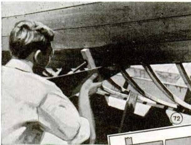
Perfect joints in divided planks are easy to make by running a saw repeatedly through the joint
