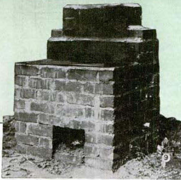
Figs. 6, 7 and 8 show an unusually attractive fireplace of brick that is a real asset to the garden landscape. It is built on two grade levels and has a high chimney for a good draft. Construction requires about 500 bricks and less than a sack of cement
