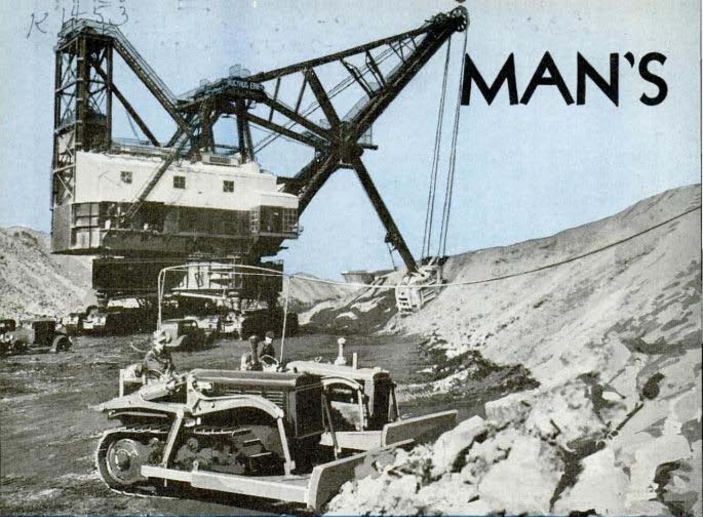
R 1453 South Melbourne, Wis Above, thirty-three cubic-yard Bucyrus-Erie stripper operating in an Indiana surface coal mine. Below, 52 men standing in heavy duty stripping dipper demonstrate size of the huge machine
