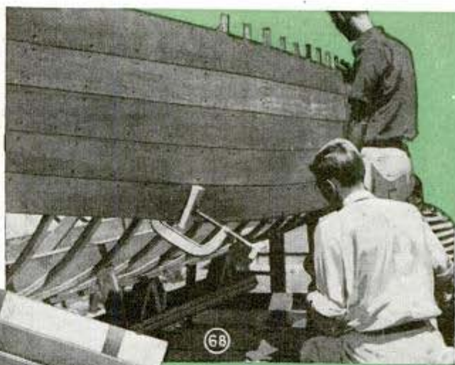
Blocks conforming to curve of ribs are used in drawing planks up with clamps
