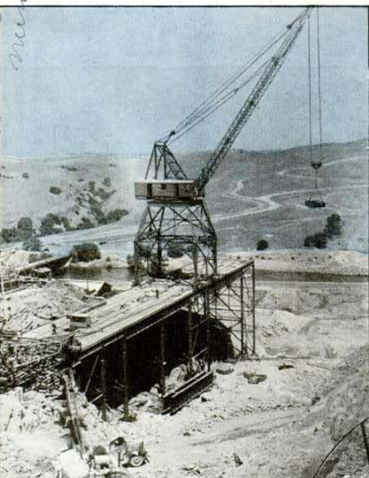
Above, American revolver type derrick hoisting material from which its own roadbed is manufactured, a construction trestle over a stream
