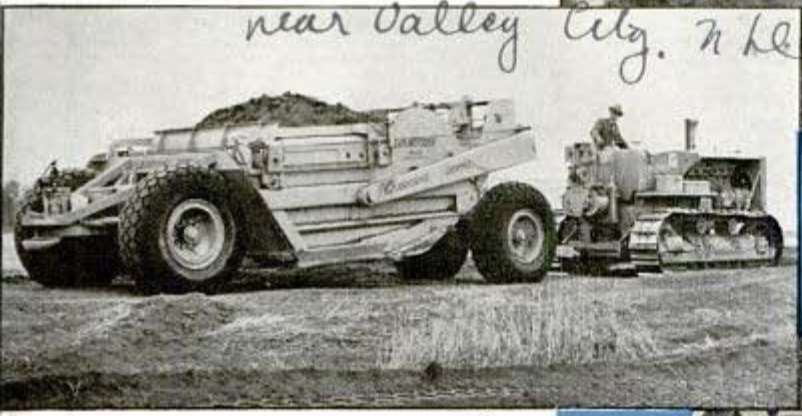
"Caterpillar" Diesel tractor and scraper making fill on county road construction
