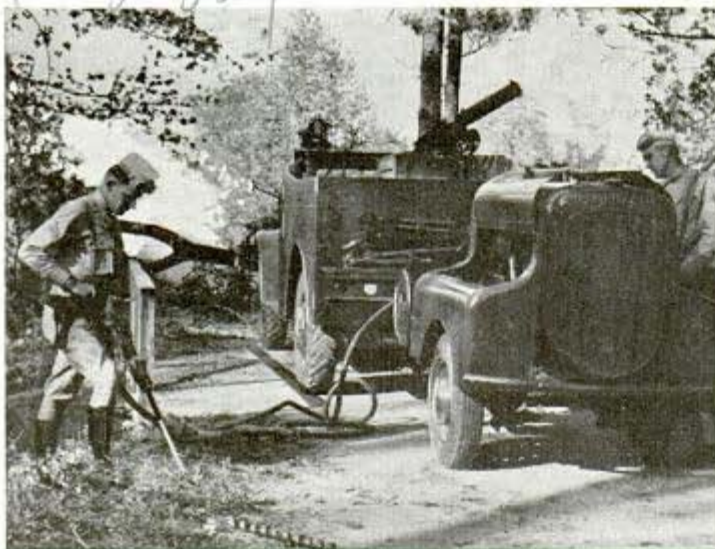
Above, the air drill starts a crater in road to slow the enemy advance. Below, a battery of gas cylinders; placing these screens is an important duty of the "explosion squad"
