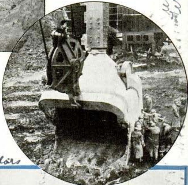
Below, huge electric shovel makes workmen look like pygmies
