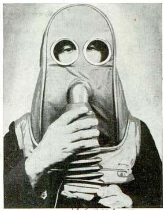
Instead of the regulation gas mask, persons hard to fit wear this helmet draped over the shoulders
