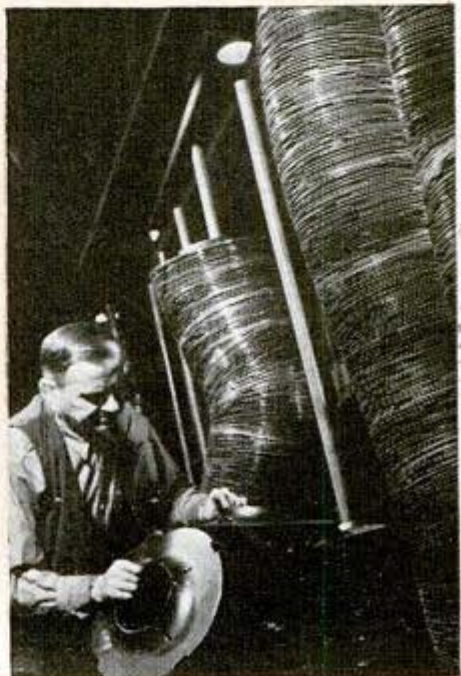
Left, Westinghouse pneumatic tube system, in which messages speed through tubes that, in this photo, resemble pipes of an organ
