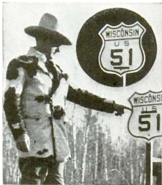
Bar over numeral tells motorist he is driving north or west; beneath, (see inset) it means south or east
