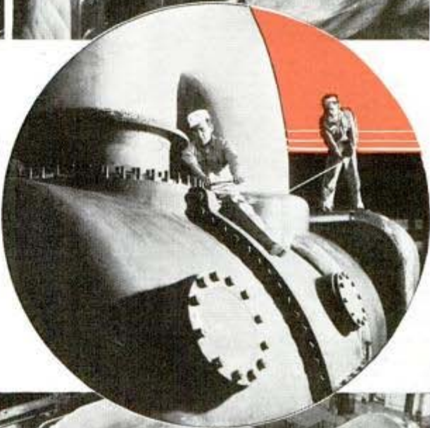
Above, left, speed-reducing gears essential for harnessing steam power in ships. Right, installing stainless steel reaction blades which will be placed in high-pressure rotor of huge steam turbine. Circle, workman using large wrench on low-pressure section of turbine. Bot. om, gigantic single-shaft turbine which delivers 220,000 horsepower to generator
