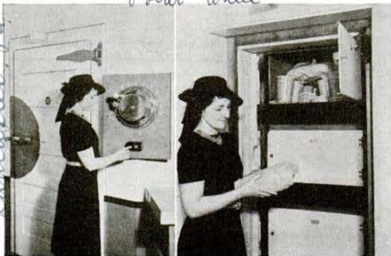
Left, a patron dials her locker number and presses button; right, swung into position, the locker is opened and frozen food is withdrawn
