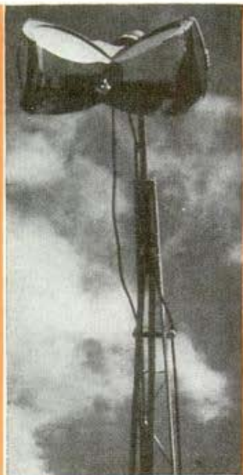
Left, leaving tunnel on Pennsylvania turnpike. Lighting is blue-green from mercury lights designed by Westinghouse. Right, light used at interchanges and tunnel approaches. Bottom, location of tunnels
