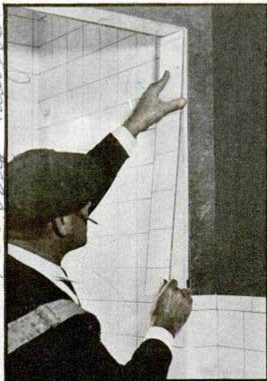
At left, nailing on strips of "tiles" which resemble ceramic tiles and help fireproof the home. Right, curtain of water flowing down roof furnishes cool shade. Below, pumping dry mineral wool into attic for insulation—result, a cooler house in summer, warmer in winter
