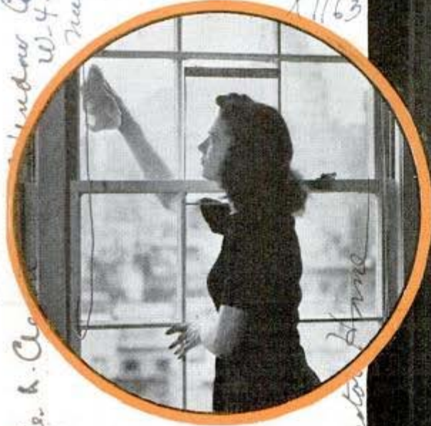
Sliding panel in lower sash (above) permits washing entire window from inside. Right, glass walls brighten the hall; below, circular parchment disk reflects light from bulbs in base of lamp
