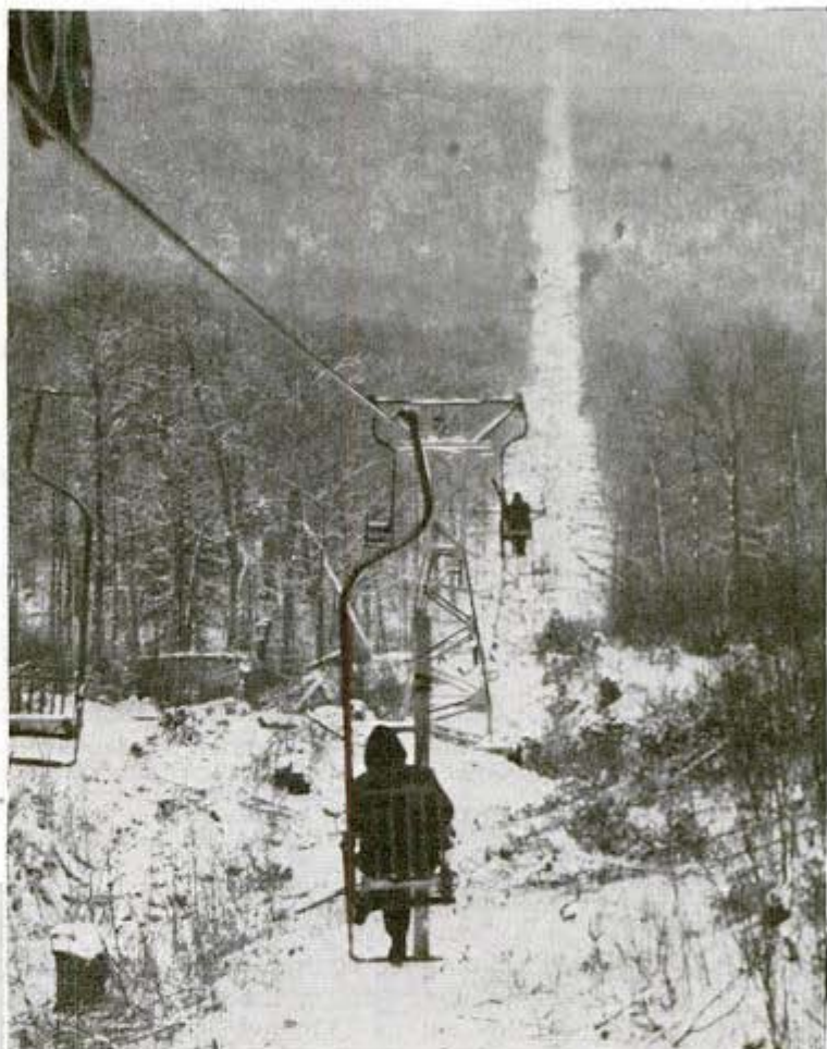
At left a skier boards a cable-hung chair for the long ride up the slopes of Mount Mansfield, Vermont. Part of this 6,330-foot chair tramway is seen above
