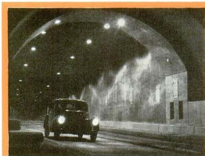
Left, leaving tunnel on Pennsylvania turnpike. Lighting is blue-green from mercury lights designed by Westinghouse. Right, light used at interchanges and tunnel approaches. Bottom, location of tunnels
