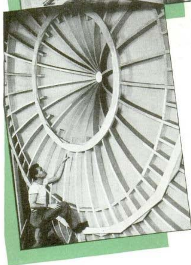
Top, left, part of air intake of Stanford wind tunnel. Inset, another flying wing model. Right, note "cuffs" at propeller blade roots that provide extra thrust. Bottom, exterior of wind-tunnel chamber
