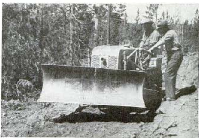
Trailmaker, above, breaks path for baby trailmobile shown at top, left. Bottom, latter machine carries gasoline to run vehicles and fire-fighting apparatus
