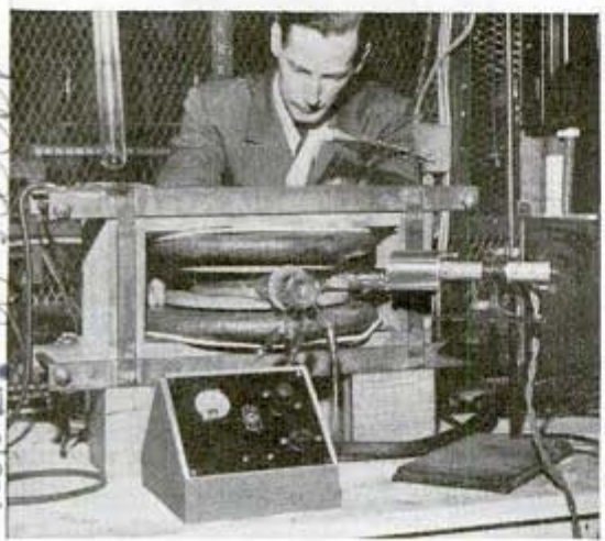
Doughnut-shaped miniature atom-smasher is shown here in special framework
