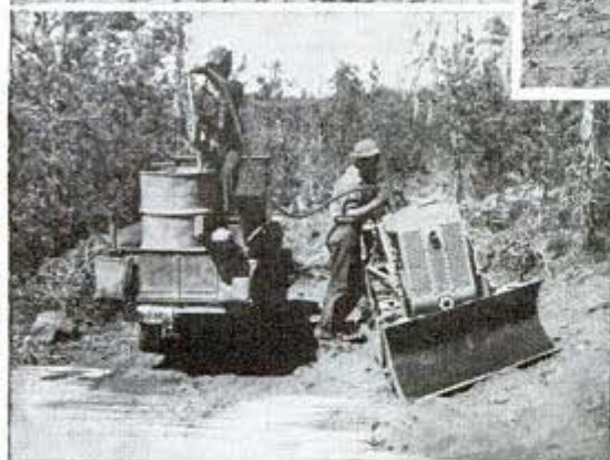
Trailmaker, above, breaks path for baby trailmobile shown at top, left. Bottom, latter machine carries gasoline to run vehicles and fire-fighting apparatus
