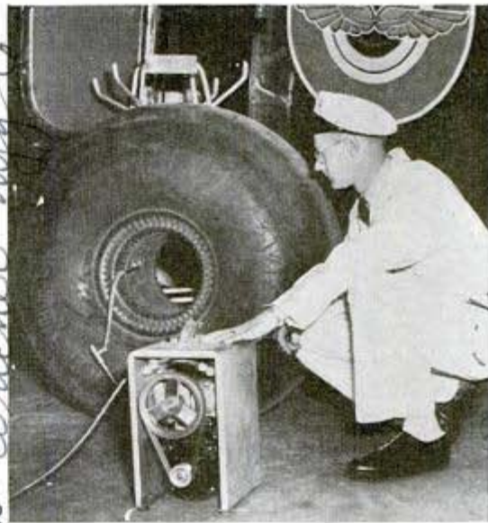
Portable vacuum pump driven by one-quarter horsepower motor speeds deflation of big airplane tires
