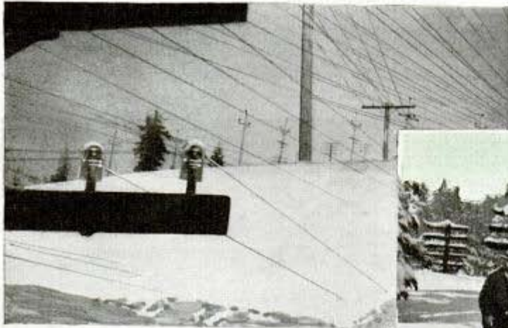
Two telephone line crossarms and lower wires are buried by snow after a storm in the California sierras, above. Right, snow is piled nineteen feet deep and wires have broken from lower crossarm
