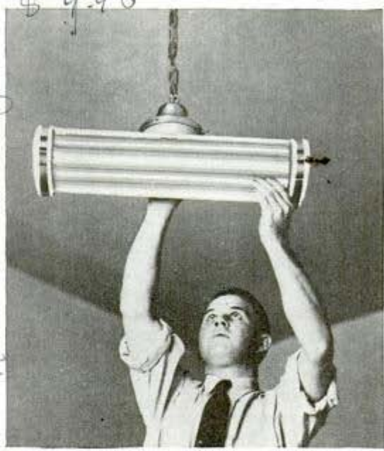
This fluorescent ceiling light is easily substituted for ordinary globe by plugging into the old socket
