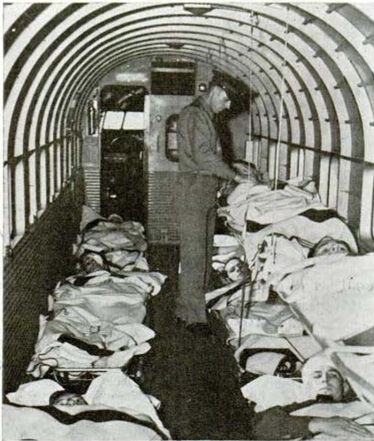
With enough space for twelve cots, this airplane which usually hauls freight can be converted into flying ambulance within twenty minutes
