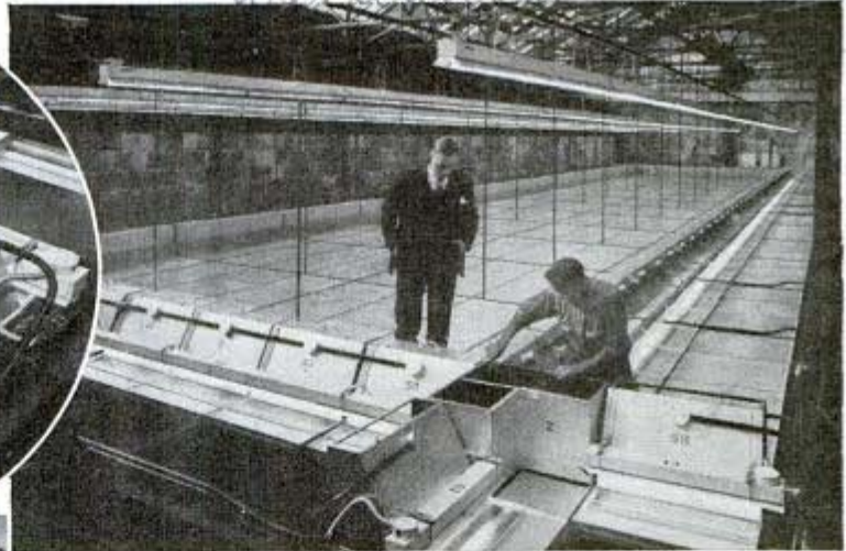
Miss Nancy Weston Above, installing "sunlight" battery over art gallery; in circle is one of the lamp units, and beneath it, through ceiling window, can be seen paintings on wall. Below, visitor sees painting in natural light.
