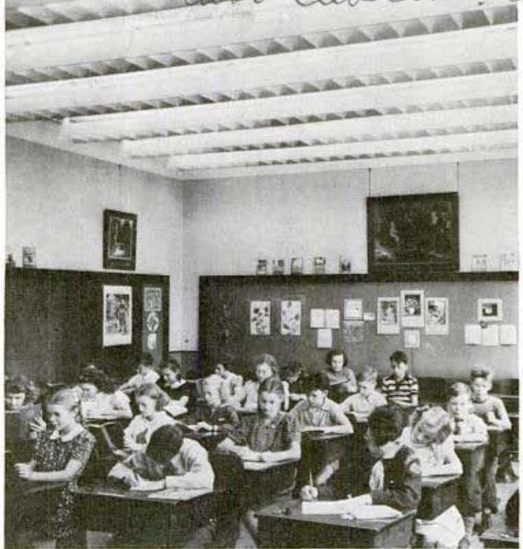
Fluorescent lamps in specially designed system of reflectors illuminate each pupil's desk in this classroom with wealth of daylight. On bright days system helps make light uniform for all
