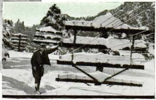
Two telephone line crossarms and lower wires are buried by snow after a storm in the California sierras, above. Right, snow is piled nineteen feet deep and wires have broken from lower crossarm
