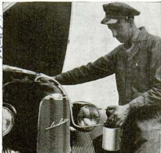
Filling station attendant removing water from radiator with siphon before adding anti-freeze solution
