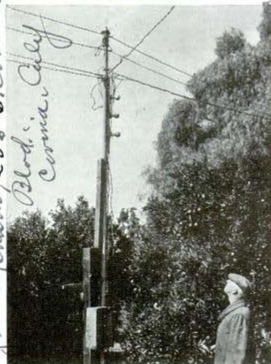
Electric lights on pole, hooked up with thermostats in citrus grove, indicate where frost is prevalent
