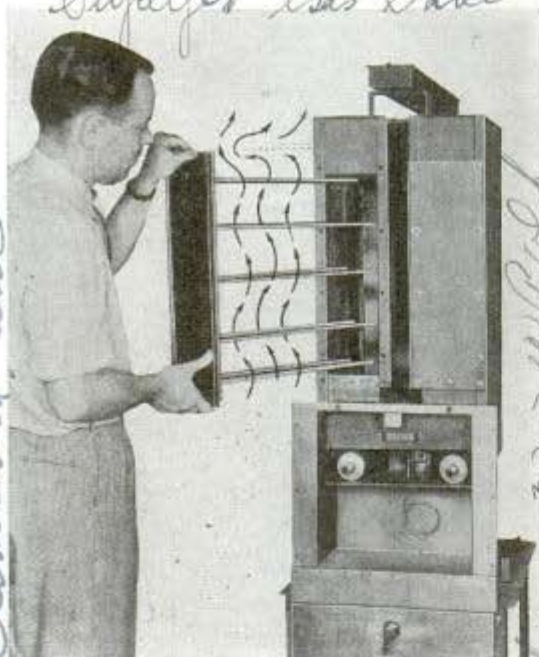
Arrows indicate hot gases zigzagging among baffles to aid transfer of heat through walls of chamber
