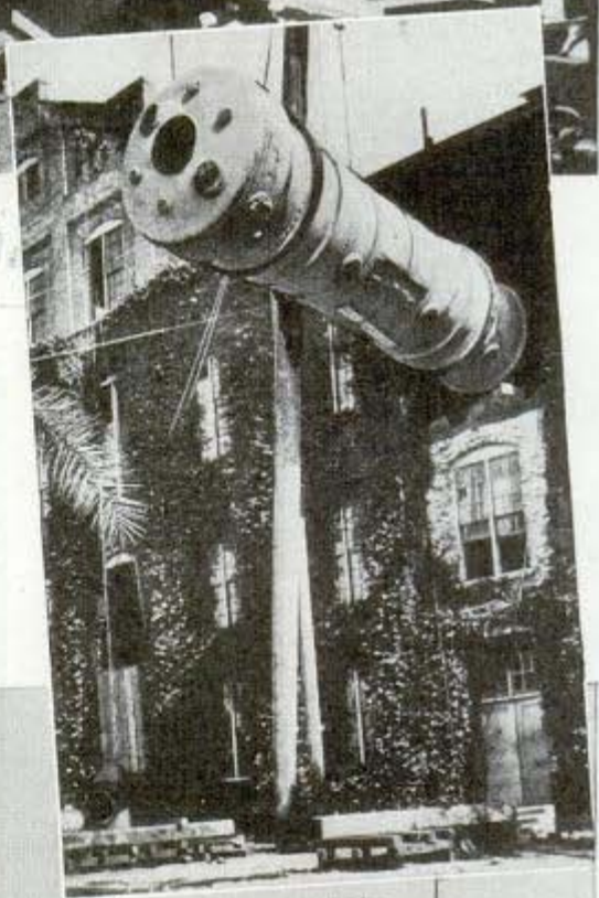
Easing 150-ton load from flatcars to barge (above) without a splash was a ticklish job. Right, hoisting forty-ton sugar dryer into third floor. Below, the seventy-nine foot "Jeep" rig with forty-two wheels hauls a big transformer
