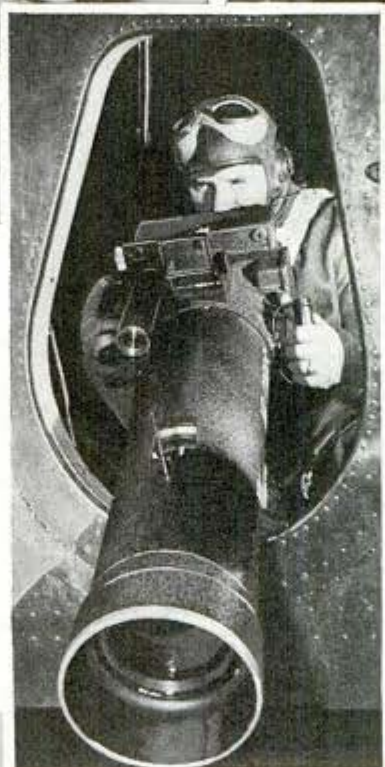
Army photographers capture thirty-six square miles of terrain with a single snap of their latest aerial mapping cameras from their photographic plane at four miles altitude. Right, "Big Bertha" camera—a forty-inch focal length camera being directed from pear-shaped opening in door of plane. Above, cameraman inhaling oxygen as he operates wide-angle aerial camera in plane high above ground
