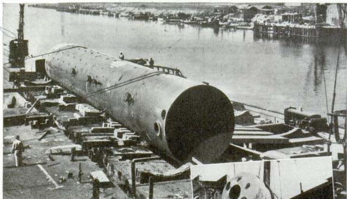
Easing 150-ton load from flatcars to barge (above) without a splash was a ticklish job. Right, hoisting forty-ton sugar dryer into third floor. Below, the seventy-nine foot "Jeep" rig with forty-two wheels hauls a big transformer
