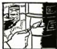
Sealing Crack in Boiler
