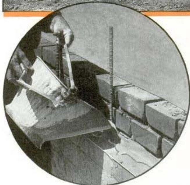
Top, putting section of partition in place. Center, one of the completed apartments. Bottom, space between inner and outer walls of brick is filled with moist concrete which flows into joints
