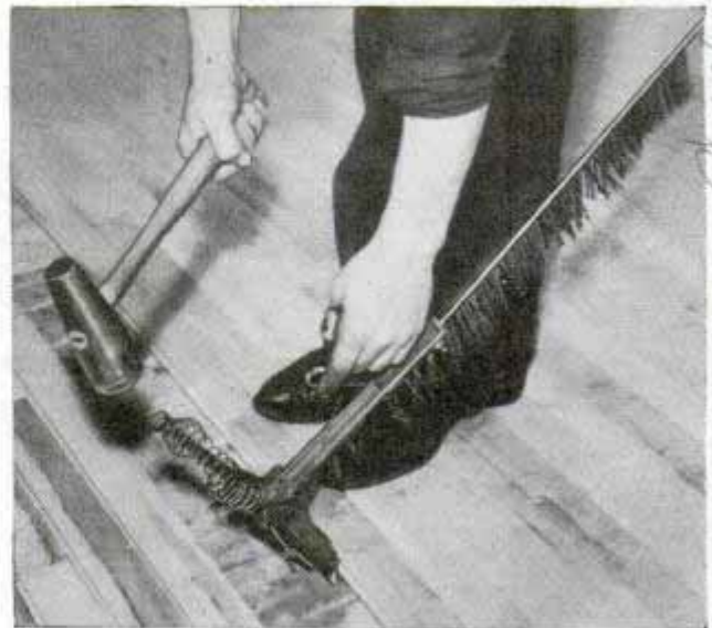
Floor nailer drives and sets nail with plunger; trigger operated with left hand feeds a nail at a time
