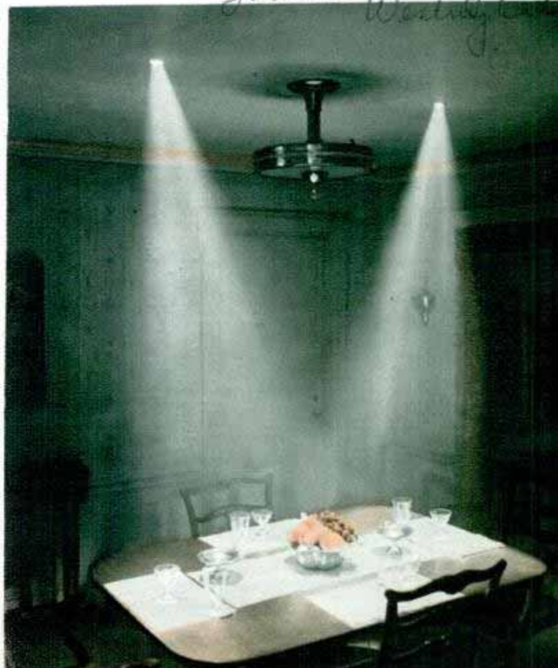
Marion Hughes. Left, illuminating dressing table with fluorescent lamps. Right, demonstrating fluorescent installation in floor lamp. Bottom, pinhole lighting of dining table with spotlights mounted above the false ceiling.
