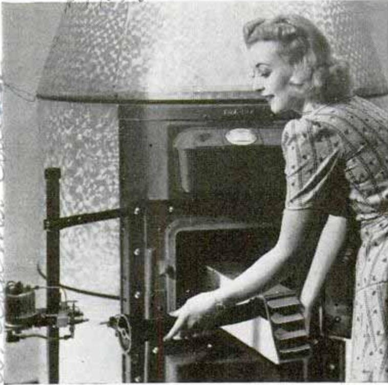
When steady heat is not needed the housewife simply plugs the automatic gas-burning unit into the door of the furnace
