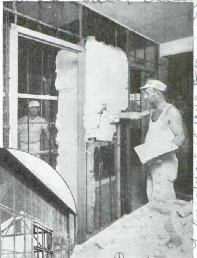
Curie Above, applying plaster to metal lath forming partition. Left, metal lath of outer wall, supported by light steel channels, ready to receive cement mortar
