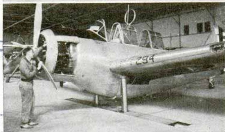
To service the plane it is hoisted by twin posts, wheels are retracted, then it is lowered within easy reach of mechanic
