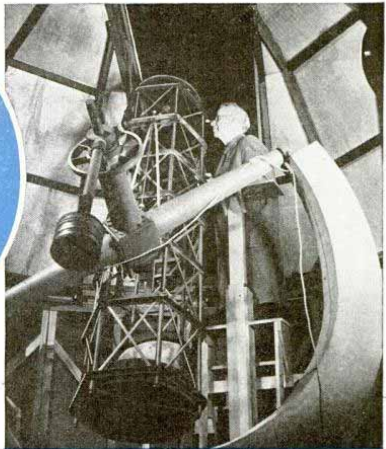
Above, Halley's Comet in 1910. Right, light from stars reflects from mirror at bottom of tube to eyepiece at top. Center, photo shows comet clearly as telescope follows it, stars appear as streaks. Bottom, two back-yard comet chasers
