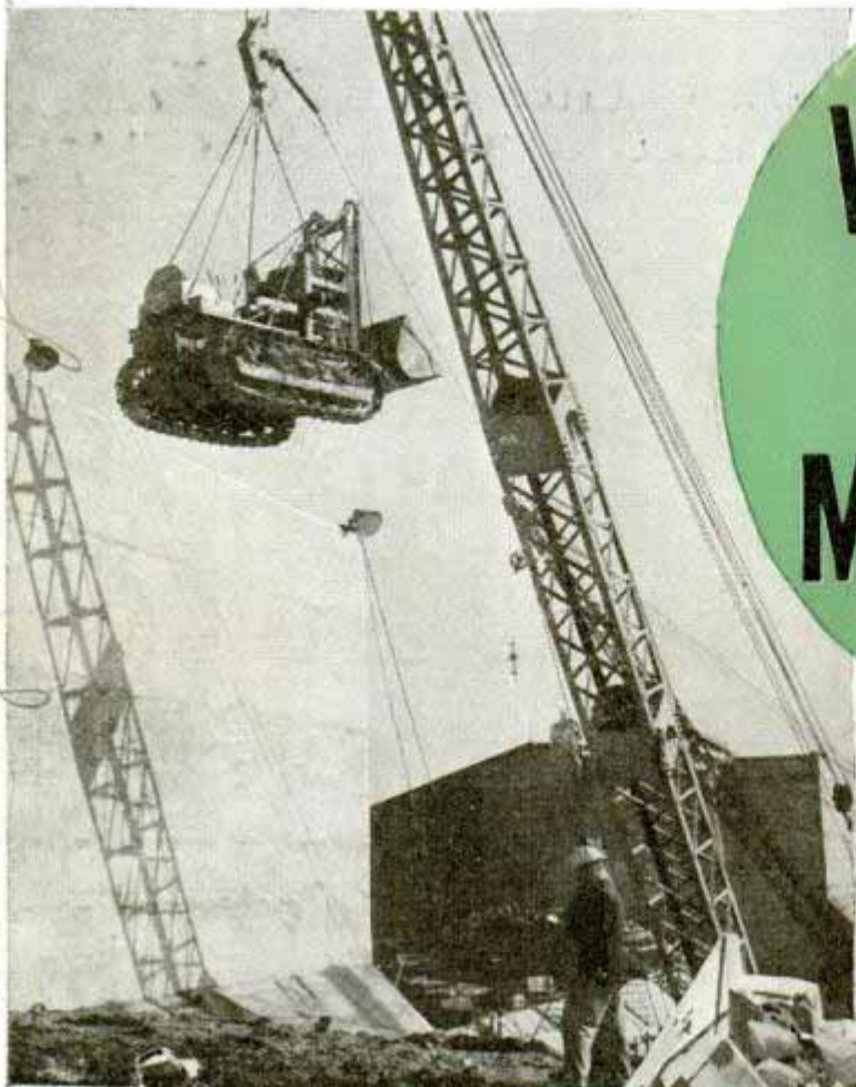
Dumpler Kocher Co 1940's With mighty machines of his own making, man is building mountains to control flood waters in southern California, where the adobe soil fails to sustain usual type dams. Of a dozen to be built, Hansen dam is the greatest to date, requiring 14,000,000 cubic yards of earth, divided by a concrete spillway. Top photo, derrick lifting tractor over fill; center, "scuttle" dump truck. Note arrangement of tires for extra power on hills. Bottom, left, placing concrete from huge bucket amid forest of reinforcing steel; right, this apparatus scoops up and dumps six cubic yards at a time into giant truck
