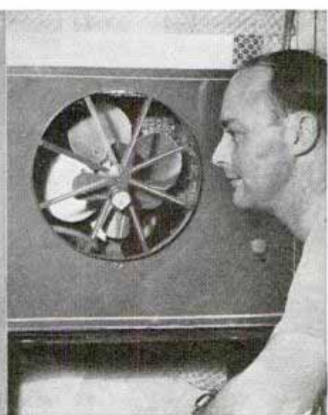
The view at left shows the wall of excelsior which is kept moist to cool the air passing through it, evaporating three gallons a day
