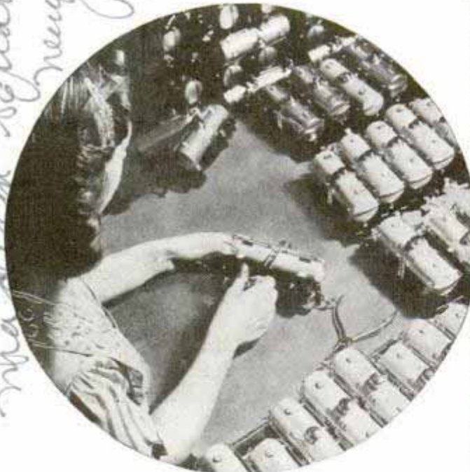
Geared at high speed to meet demands of model railroaders and purchasers of toy trains, production lines in miniature railroad factories, as complete and efficient as those of large automobile plants, now turn out in one year 550,000 tiny locomotives, 1,650,000 cars and more than 5,000,000 feet of track. About ninety per cent of this is sold in the month preceding Christmas
