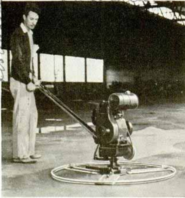
Gyrating paddles of electric "trowel" impart finish like marble to surface of newly laid concrete floor
