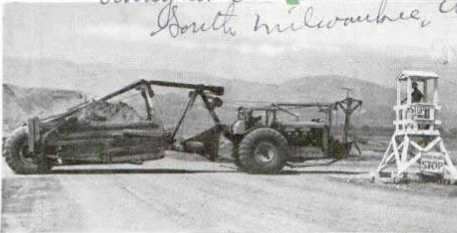
Top, called a "dragveyor," this monster pours a steady stream of earth into truck by means of a conveyor belt, a power shovel and drag line keeping supply going. Circle, gigantic scraper, coupled to a 160-horsepower Diesel engine on two wheels, picks up twenty-five cubic yards with ease. This revolutionary earth mover, known as a Tournapull, can do the work of 300 horse-drawn wagons like the one shown at right in the picture
