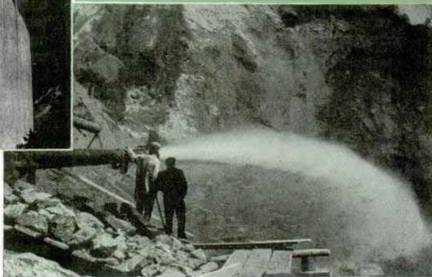
Top, snowplow cleaning up drift. Center, drawing of double-deck railroad and highway bridge which will span river 500 feet above river bed. Bottom, making highway cut with hydraulic equipment
