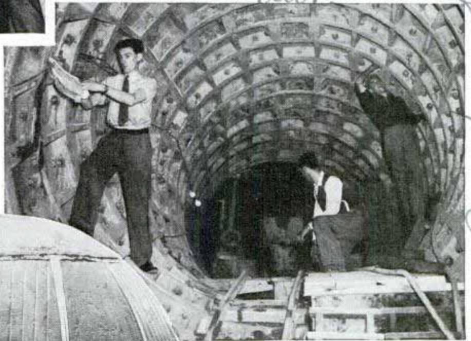
In America as overseas, preparations against possible air raids are being hastened. One manufacturer in the United States developed the steel "tent" at top, in which a family of six could take refuge. Built on a concrete base six feet square, it would resist anything but a direct bomb hit. In the center, workmen are finishing the steel-and-concrete walls of a tunnel leading to one of England's largest underground shelters, adapted from a subway. It accommodates thousands and is easily accessible. Left, a concrete "igloo" built in five hours for test purposes on the Potomac
