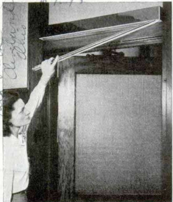
Three-foot glass tube being inserted over doorway emits invisible curtain of germ-killing ultraviolet
