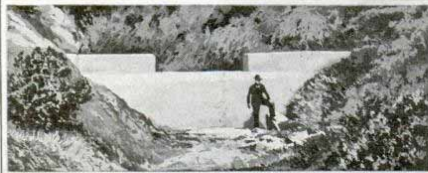
27 DAM PROPER COMPLETED WITHOUT RETAINING WALLS
