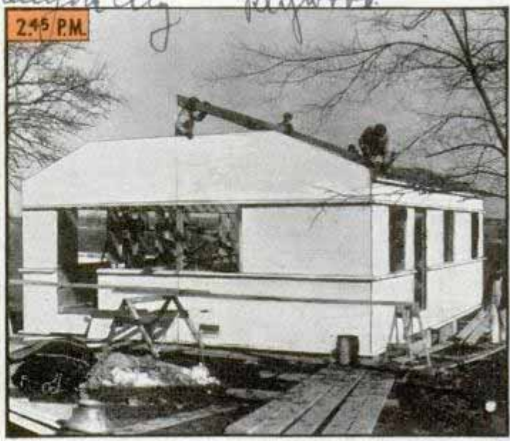
Bottom, this page, additional stages in construction: 1:20 p.m., ceiling rafters dropped in place, and, 2:45 p.m., third side-wall tier is in and one-piece gable is being dropped into place
