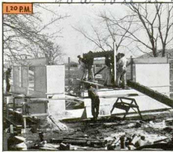
Bottom, this page, additional stages in construction: 1:20 p.m., ceiling rafters dropped in place, and, 2:45 p.m., third side-wall tier is in and one-piece gable is being dropped into place
