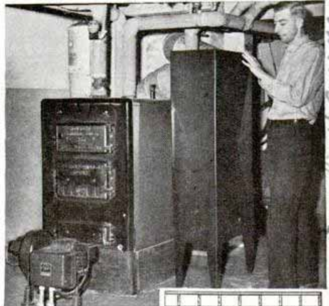
Above, the fuel saver is installed next to furnace to warm basement air, which passes upward through it. Diagram at right illustrates how it can be used as an auxiliary to hot-water heater
