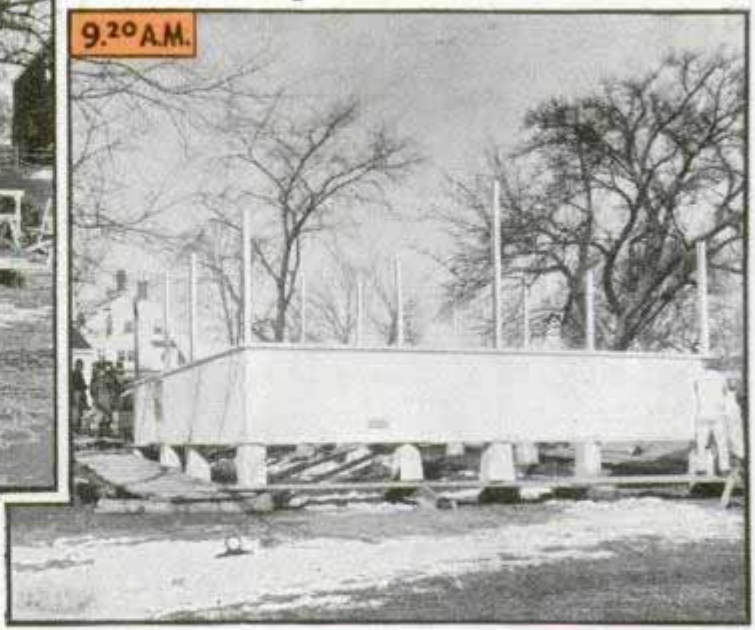
Tops of this and page opposite: 8:10 a.m. side wall supports and floor joists being attached to concrete piers; 9:20 a.m., first row of prefabricated exterior side walls set up; 10:30 a.m., second tier of side walls almost attached and windows taking shape, and at 11:50 a.m., workman gluing top of side-wall tier so third tier may be fitted above it and nailed
