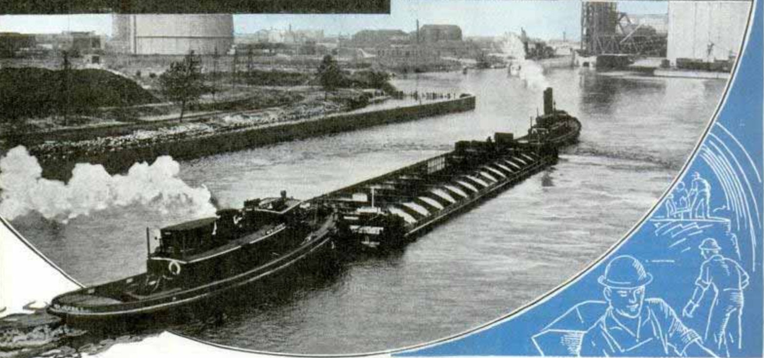
Handhogs at upper left bore tunnel by hand, peeling off clay with wire knives. Right, hauling out trainloads of muck. The tugs are escorting prefabricated section of tunnel to be sunk into river bed
