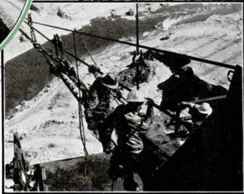
Like a giant roller coaster, a ten-mile belt hauls 22,000 tons of sand and gravel daily from Redding, Calif., to site of Shasta dam, crossing the Sacramento river twice. This conveyor system, longest in the world, consists of twenty-six relays of endless belt, each driven by 200-horsepower motor except the last three; these (circle, left) go down-grade and generate power used on other sections. Upper left, some of the 16,000 rollers on which belt travels. Upper right, gravel piling up at end of belt line. Lower right, connecting three-inch cable to bearing at top of 460-foot cableway head tower at dam site
