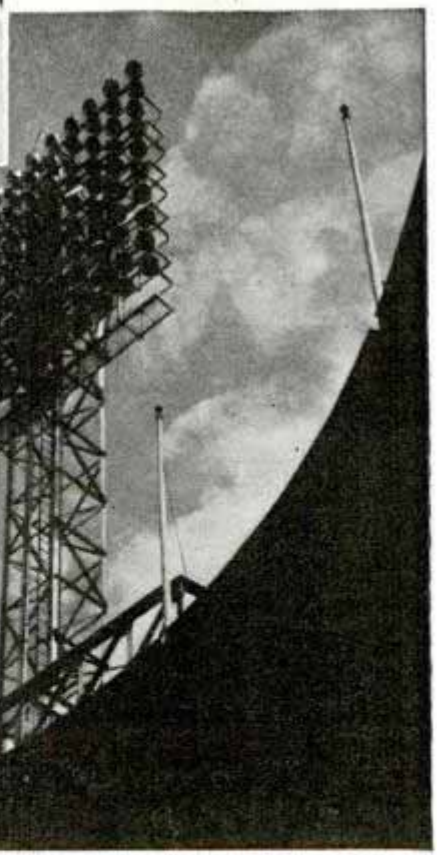
Baseball field marked with 836 boxes, at top, which were used by engineers as targets for aiming the lights in making final adjustments of New York Giants' 200,000,000-candlepower lighting system. Bottom, one of the biggest of the eight steel towers, containing 120 lights, located on grandstand roof in outfield
