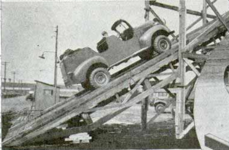
Above, one and one-half ton army truck bouncing up steep six-foot incline in test; below, light trucks must be able to ascend grades like this in low gear, carting a thousand-pound load. At the front ends (right) truck radiators and headlights are guarded by heavy metal grill
