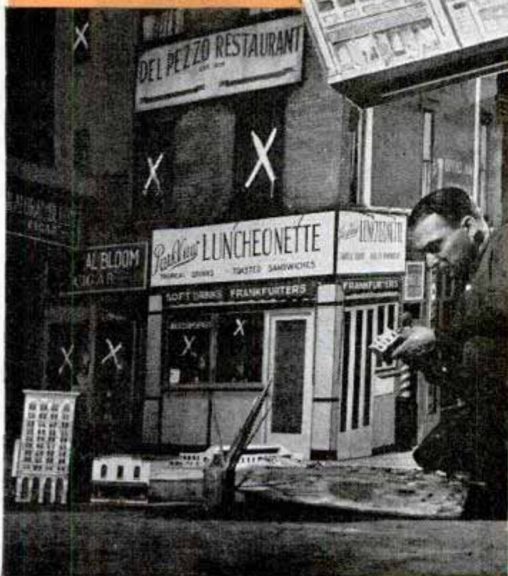
Composition walls are glued to building frames made of wood, above; ordinary clothespins holding them together until glue sets. Below, a study in proportions; model builder, squatting near tiny street being built for another diorama, paints dwarf buildings that form part of city built to order. X-marks on windows protect glass from breakage
