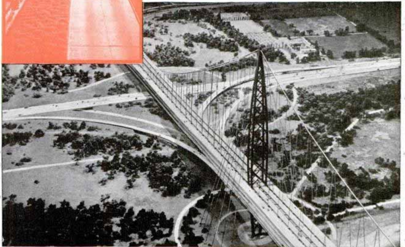
Top, junction of two major arteries in the future. At left, modern divided highway in New York is jammed because of cars turning left in front of heavy traffic at grade intersection. Below, each traffic lane, divided according to speed, has a separate approach and deck on suspension bridge of the future
