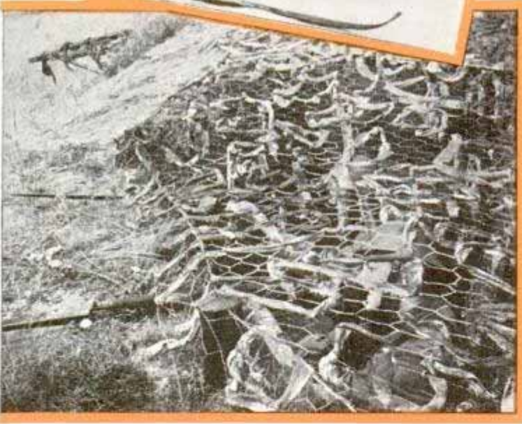
Warplanes approaching camouflaged anti-aircraft battery in maneuvers (top). Mechanized cavalry vehicle, painted white, blends with snow in Fort Knox maneuvers (inset). Machine-gun crew (center) in white costume for maneuvers over snow-covered terrain at Fort Brady, Mich. Bottom, Dutch coastal defense infantrymen in trenches camouflaged with wire netting covered with pieces of jute, similar in color to surrounding fields and meadows
