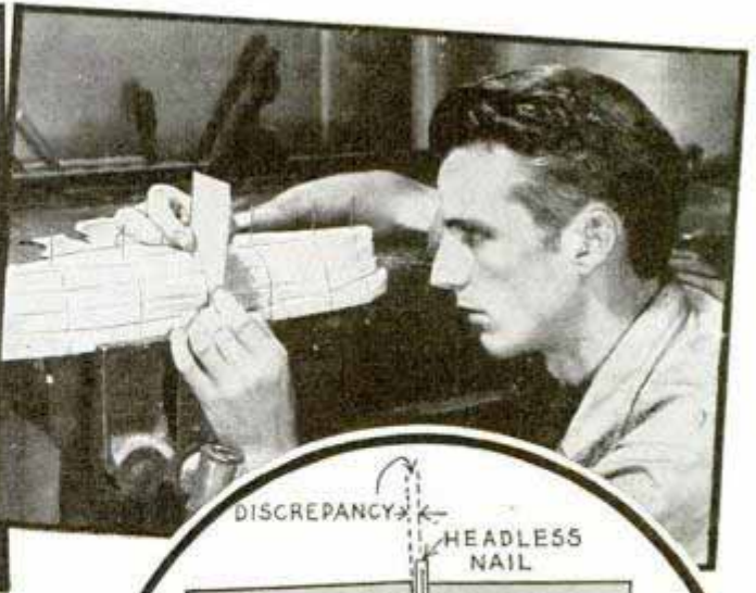
NAILS ARE DRIVEN VERTICALLY WITH AID OF SQUARE
