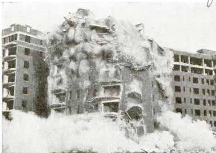
Apartment building going down in a puff of smoke and dust as wreckers set off charges of dynamite to blast away pillars
