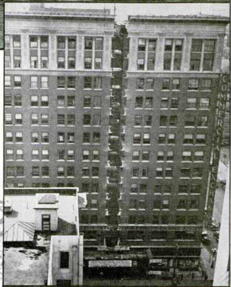
Moving a house across Puget Sound by barge, top. Below, five-foot section of skyscraper is cut out and building rejoined
