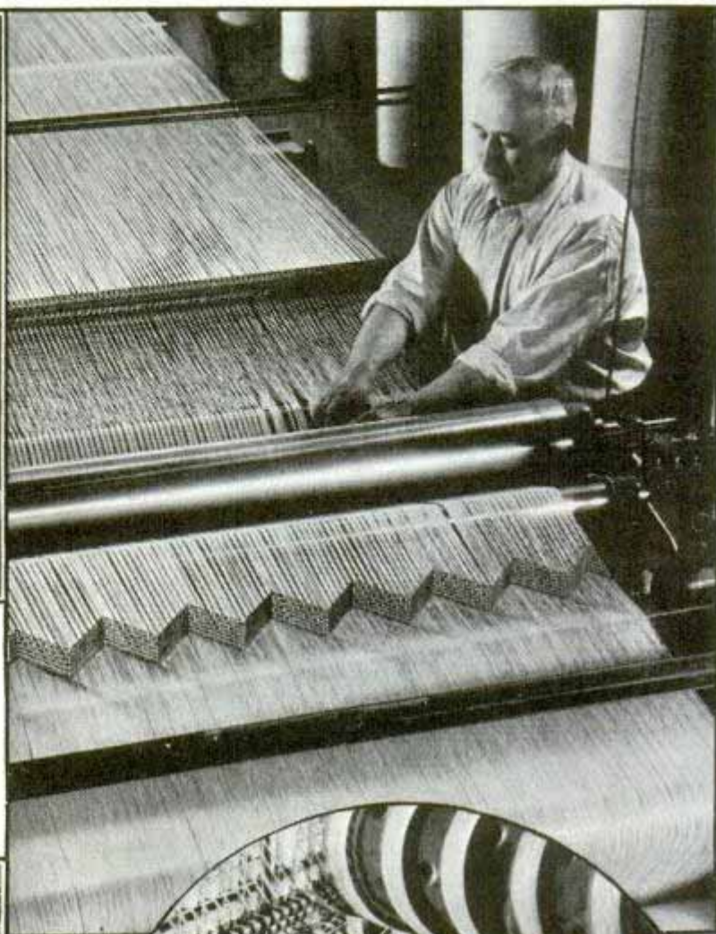
In ancient times a lifetime frequently was spent weaving one rug. Today American manufacturers produce a million pounds of rugs each working day. Above, a card puncher "piano playing" a pattern, translating a paper design into the cards on the loom by pressing keys on the cutter
