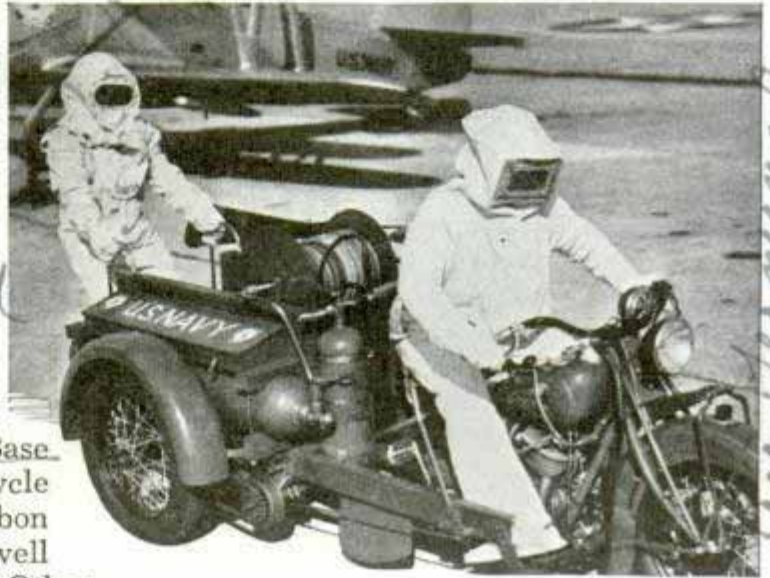
Top, left, holding bolt cutters used in rescue work, and, right, unreeing carbon-dioxide fire hose. Bottom, asbestos-clad firemen on motorcycle "fire truck"
