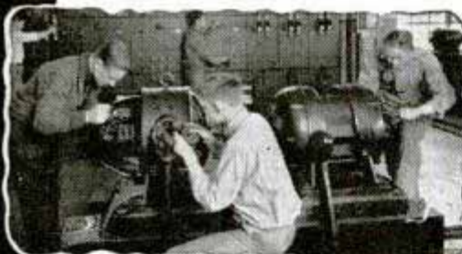
Students repairing motor generator set, and operating one of our power switchboards.
