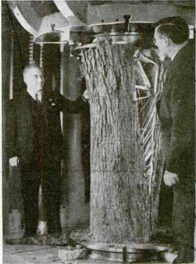
clerk At left is the research machine that can exert a 3,000,000-pound push; it was built to test fabricated aluminum products. At right, it uses a third of its muscle power to split a sturdy oak *
