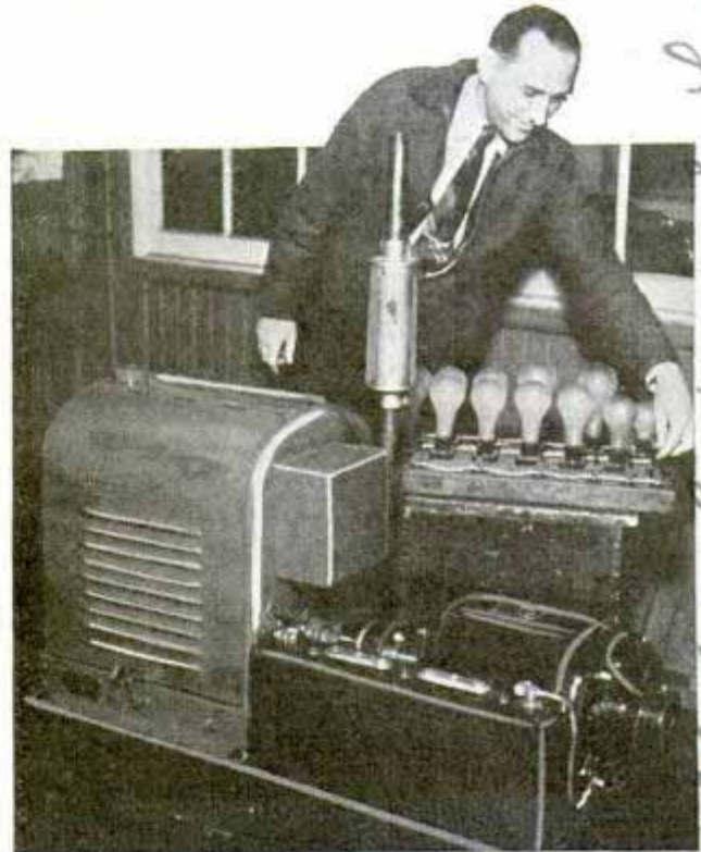
Turning on any lamp in house operates relay for gasoline engine starter and sets generator in motion
