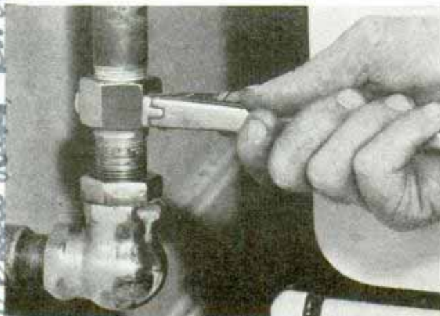
Pipe joint with built-in shut-off valve closes line against leakage if pipes are to be disconnected
