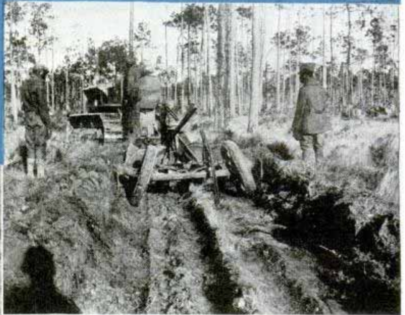
Brush is burned when heavy snow makes it safe, top. Below, at left, CCC boy planting seedlings; right, constructing fire-control line in southern pines with double moldboard plow
