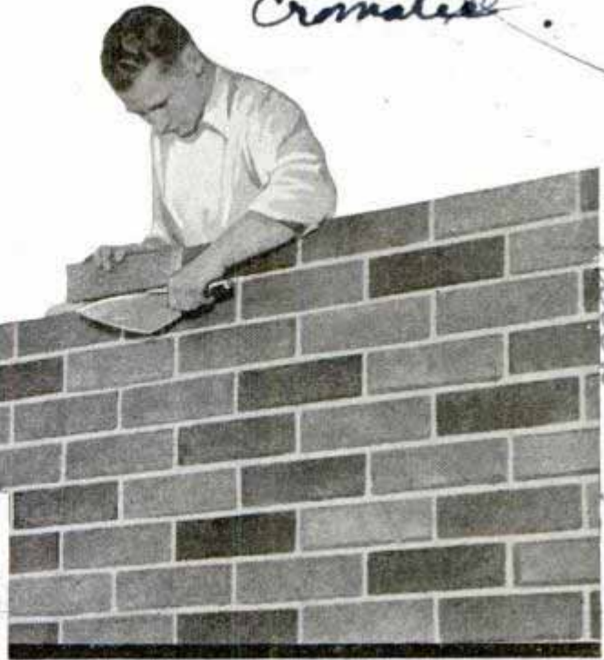
Tile is as easy to lay as brick and it covers twice the area. Note cellular design of samples at left
