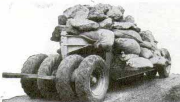
Nine tires under heavy ballast pack the earth smooth
