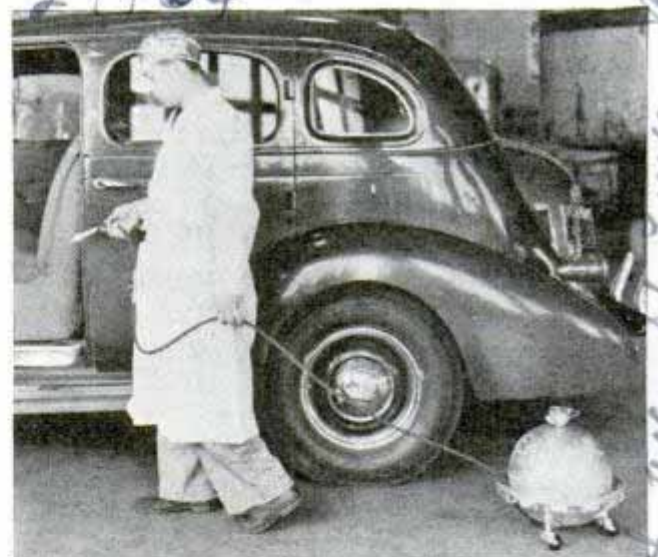
Hydraulic brake systems are serviced quickly by portable pressure tank that resembles a torpedo
