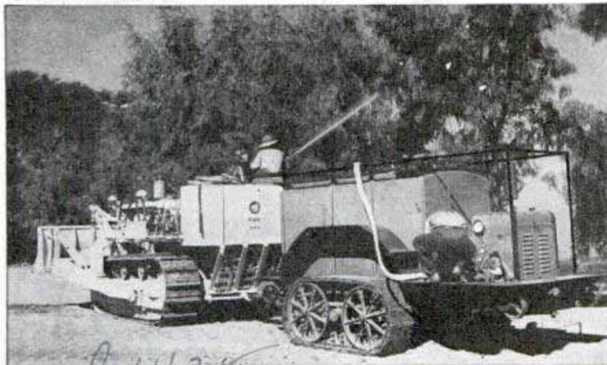
Fire engine carrying own water tanks can quit road and travel over rough country on its treads
