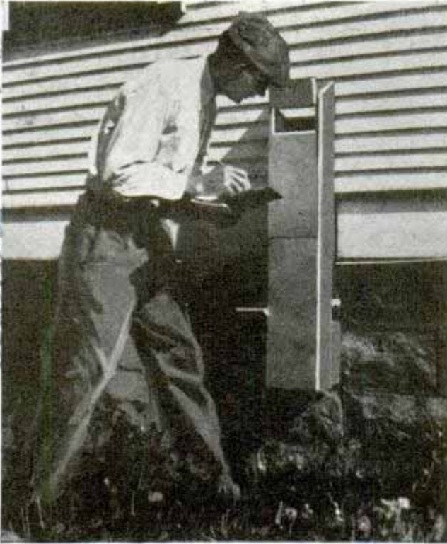
Gas meter dials can be seen through periscope in house wall so reader needs not enter the building
