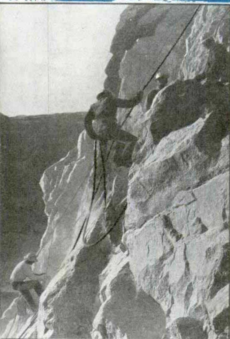
Top, hopper with tubular spout for pouring concrete into wall forms. Center, draftsman's conception of completed dam. Bottom, jackhammer operators working on steep abutment walls
