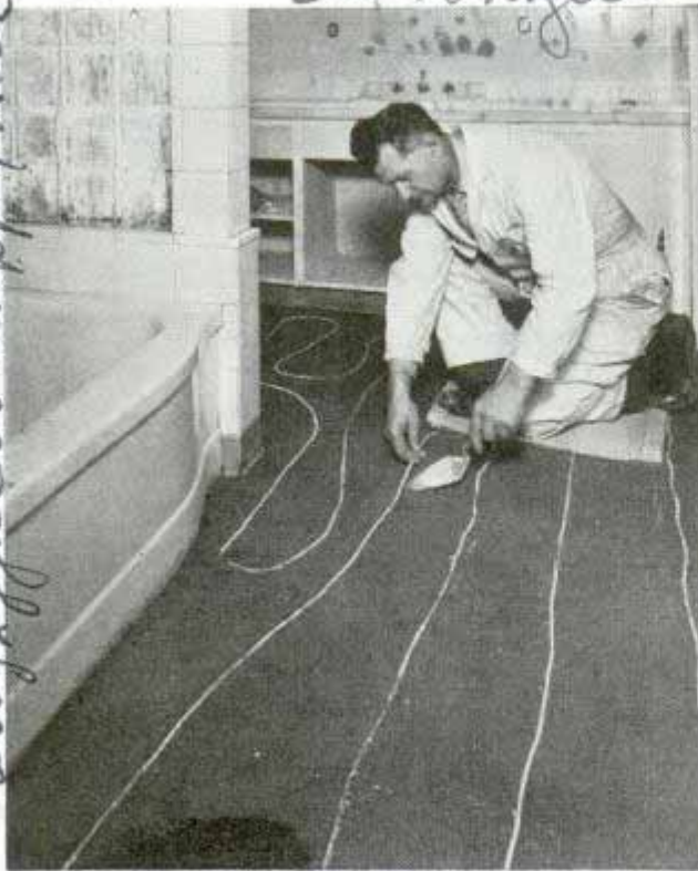
General Electric Cable any office or supply house Laying electric cables beneath tile floor of bathroom to warm floor at turn of a switch in bedroom
