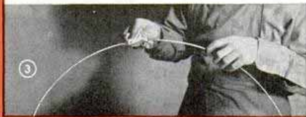
Polishing is done with silicon-carbide abrasive. For the last stage use red rouge (above), which is then washed off with muriatic acid (below)
