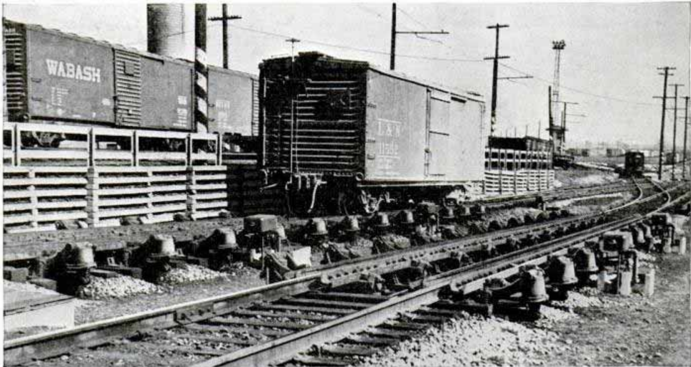
Humpmaster, top, watches operations from post directly above hump and has telephone and loud-speaker connections to every tower and shanty office. Below, a heavily loaded boxcar slows down on a retarder
