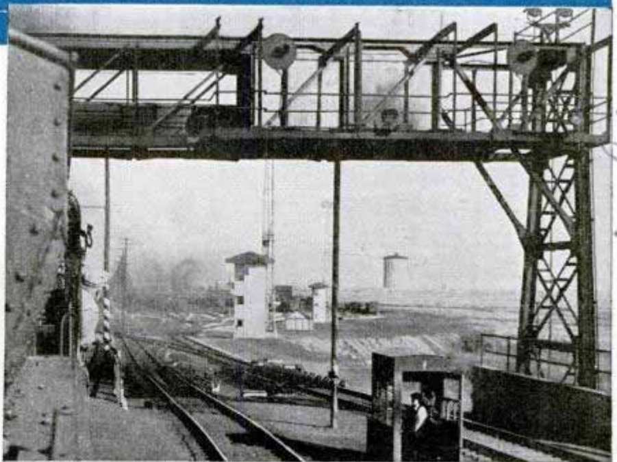
Towerman at top operates switches sending boxcar to proper track, and, judging speed and weight of car, turns controls applying retarders. Bottom, view at hump as powerful engine pushes last car down grade. Foreman in shanty supervises uncoupling cars according to "train consist" list
