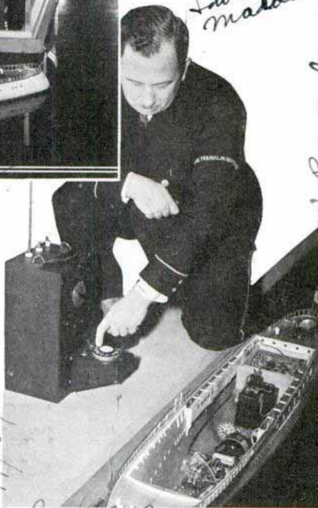
Left, radio-controlled boat responds to orders transmitted by short-wave impulses. Below, operating new telephone dial that is used for selecting the proper impulses to send in executing any given maneuver
