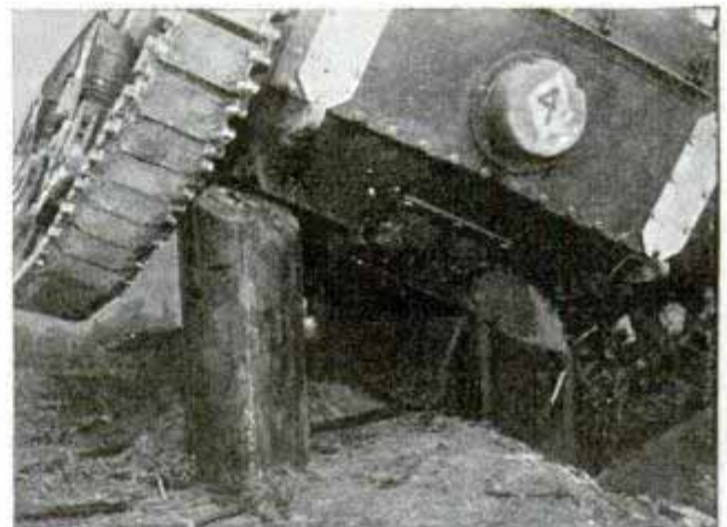
Barrier of the type which has been found successful in stopping advance of tanks
