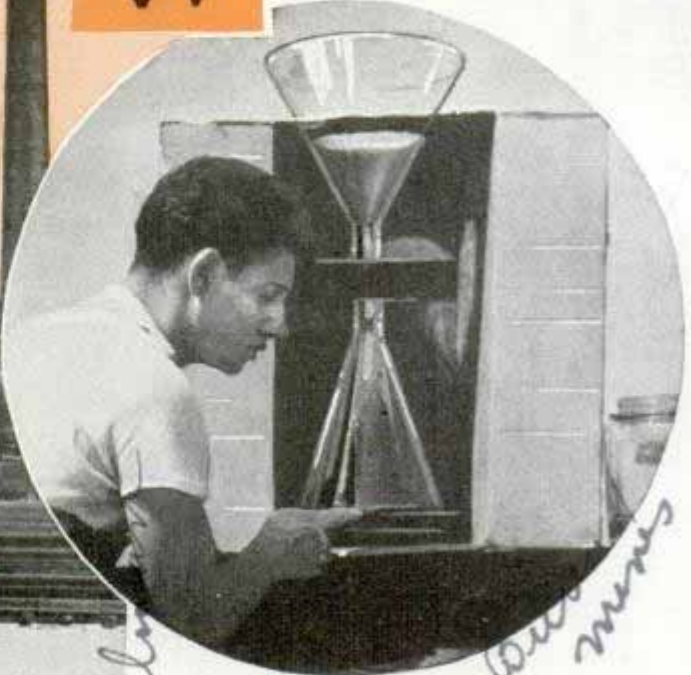
Smoke density chart, below, is held fifteen or twenty feet from eye until lines converge, then compared with smoke under observation; 40-per-cent density is allowed
