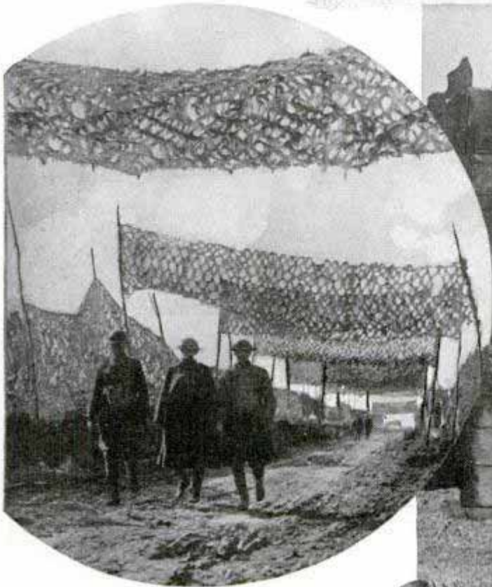
Above is an example of the method of camouflaging roads in war zone. Flimsy cloth or fish netting is strung across and alongside road to make it invisible to aerial observers. The weird masquerade shown at top, right, was designed for scouting from treetops, where the broken stripes in black and white blend with sky and branches
