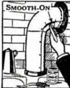
Stopping smoke leaks
