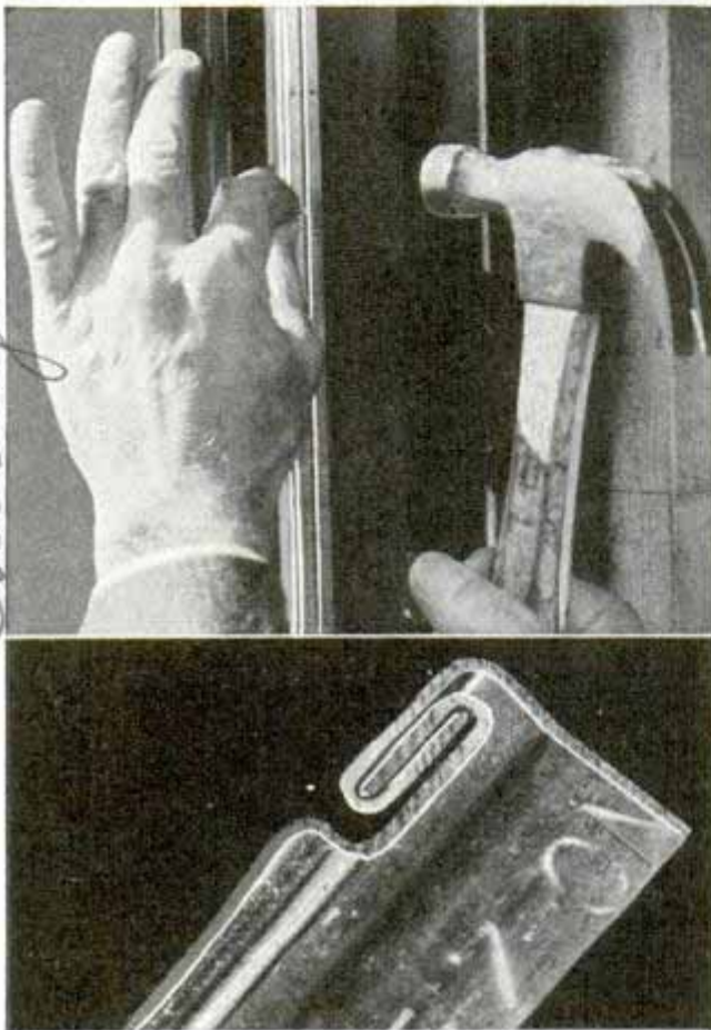
It is easy to nail weatherstrip on window frame and sash. Below, interlocking sections keep out wind
