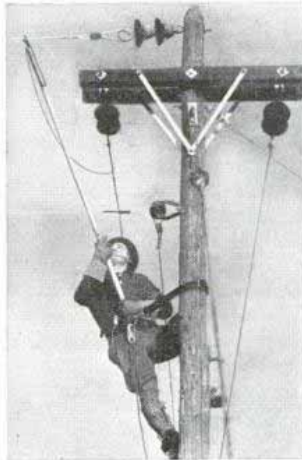
Left, "hot sticks" hold high-tension wires at safe distance while men work on pole. Right, lineman handling "hot" wire with extension tool
