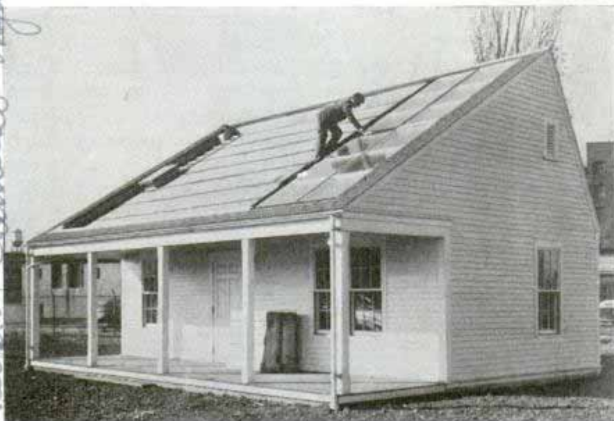
Heat trap under glass roof causes sun's rays to heat water which is then stored in basement tank for use in warming home during cold weather
