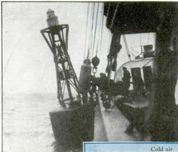
Top, placing acetylene gas tank in lighted whistle buoy; as buoy rises on wave, air is drawn in at whistle; as it sinks, rising water compresses air and forces it out through whistle. Diagram shows how air currents affect foghorns. Below, Coast Guard lifeboat in surf, and Ambrose lightship at New York harbor entrance
