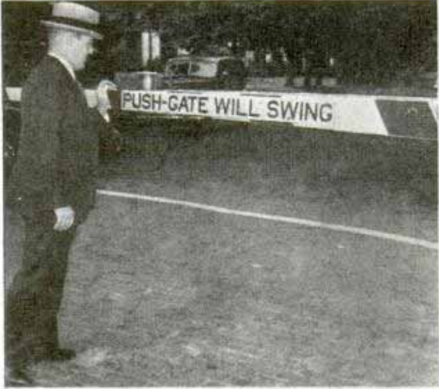
Pushing railroad gate to prove it really will swing to release trapped motorists as sign indicates
