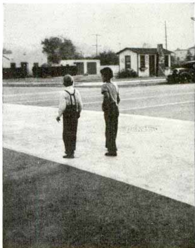
Wide strip of white to mark crosswalk over highway silhouettes pedestrians so motorist can see them
