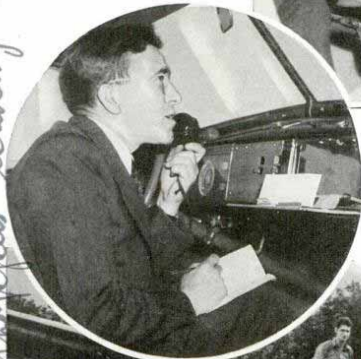
Two-way radio enables a ground crew to track down the metal two-seater sailplane owned by one gliding club. The sailplane, on endurance flights, may travel several hundred miles from starting point and a special lightweight radio working on five-meter wave length guides the crew following in an auto also equipped with the two-way radio. Above, sailplane in the air and pilot giving instructions on radio to crew on ground
