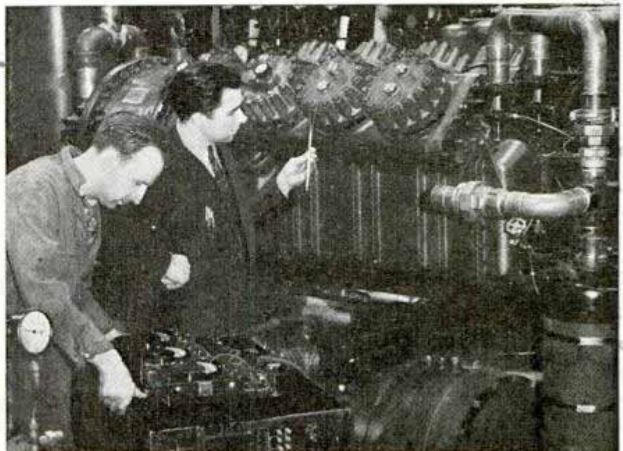
Compressor of air-conditioning unit is cooled by its own refrigerant gas
