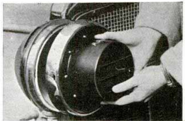
Fitting three-slot hood over automobile headlight
