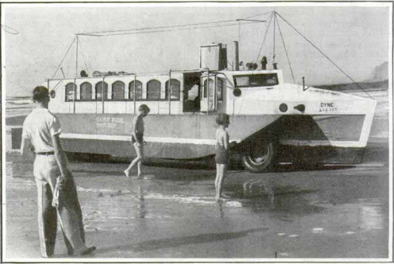
Boat equipped with wheels can go ashore where there is a sloping beach to pick up load of passengers and then launch itself again into deep water for a round-trip pleasure ride
