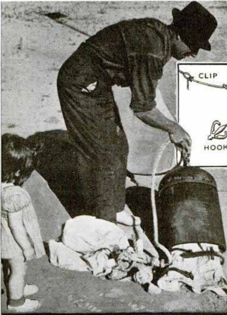
Communities inaccessible by rail or located in rugged country are being served by nonstop planes that pick up and deliver mail. At each point on the modern "rural" route, the plane drops a pouch and picks up another suspended on a line between two tall poles. A grappling iron let down by the pilot engages the line so the mail bag may be hauled into the plane. Top, left, dropping pouch and picking up another. Right, the grappling iron. Center, sketch of pickup system. Bottom, left, mail clerk emptying pouch to take letters by auto to the post office
