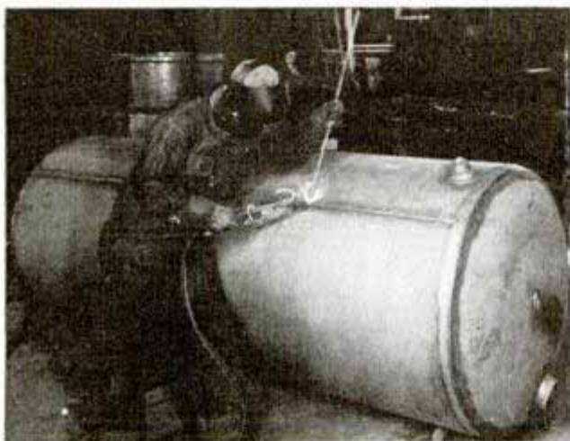
Monel-metal gasoline storage tank being fabricated by the atomic-hydrogen welding process
