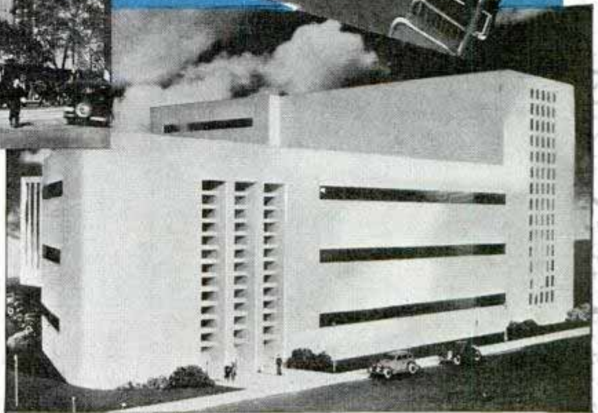
Windows are abolished in the modern store and factory. Scientific lighting, often with the new fluorescent tubes and with daylight coming through glass-block walls, saves maximum space for sales display and machinery. Environment is under complete control, air-conditioning systems providing optimum "weather" for work. Above, windowless Sears, Roebuck & Co. store in Baltimore. Right, model of factory just completed for Church & Dwight, soda manufacturers
