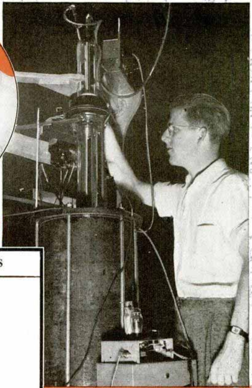
Upper left, experimenting with hearing aid; right, measuring sound transmission in gas. Various gases humidity and temperature all affect the distance sound travels. Below, decibel scale of common sounds
