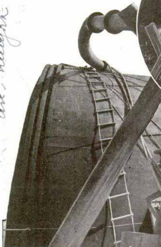
Right, wheat dumped into compressor pipes is forced into tank shown below. Sketch, at bottom, right, illustrates the tank submerged in lake.
