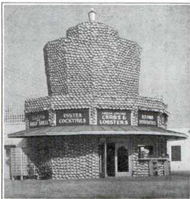
Appropriate exterior for this sea-food cafe in Los Angeles consists of 10,000 abalone shells
