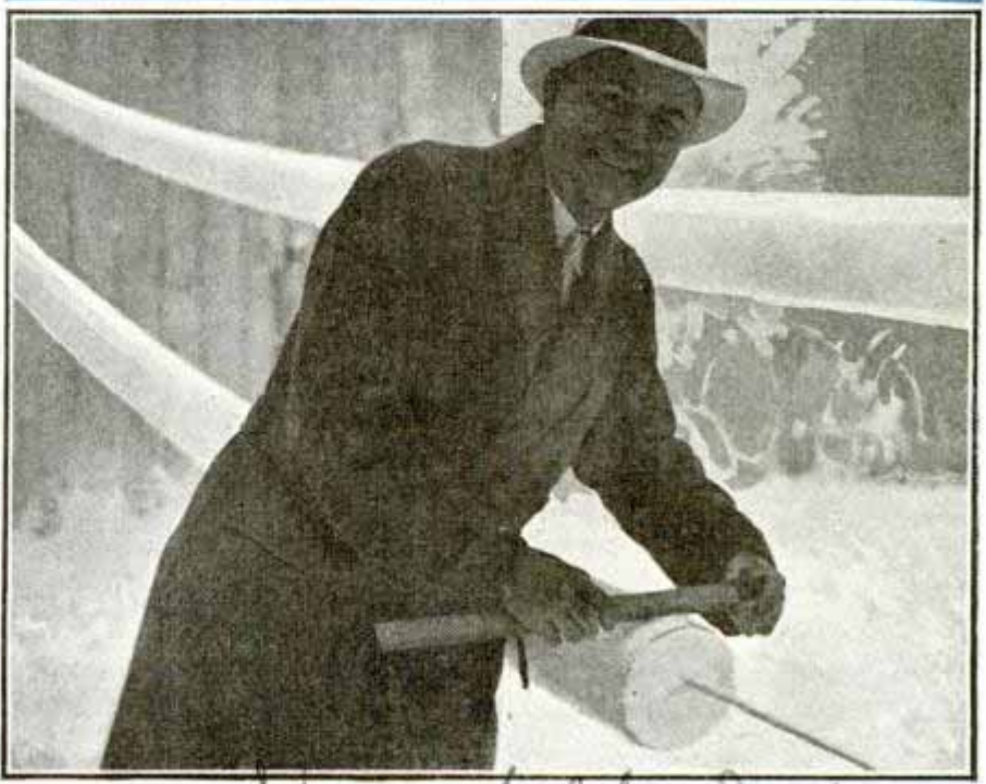
How snow fence controls formation of drifts (upper left); snow-plow clearing road in Sierras (right), and seven-inch deposit of wet snow on three-sixteenths inch electric-light wire (below). The snow weighs approximately fourteen ounces to the foot
