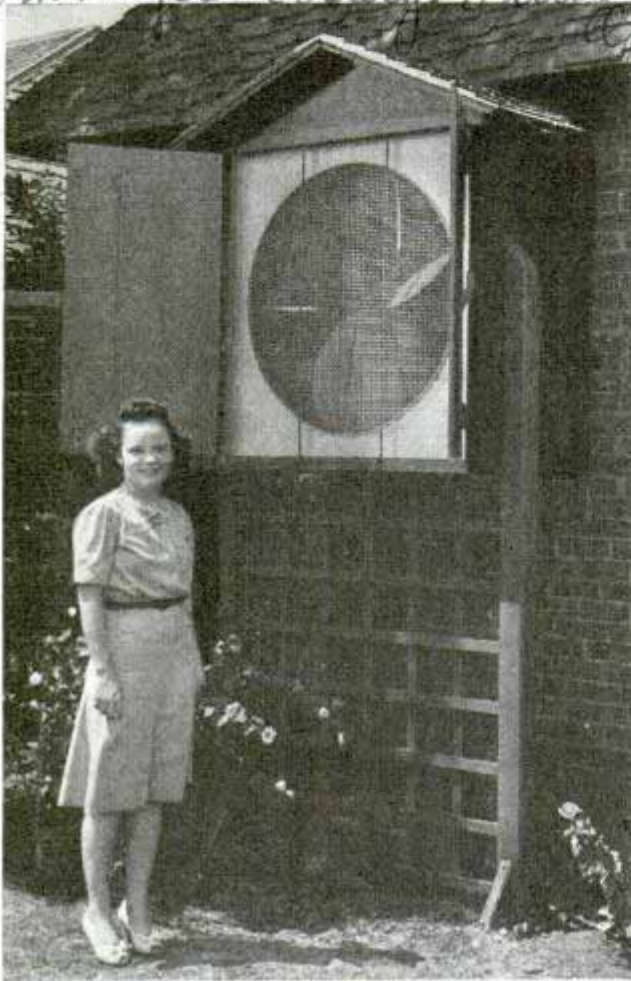
Fan mounted outside of window draws air from house fast enough to make complete change once a minute
