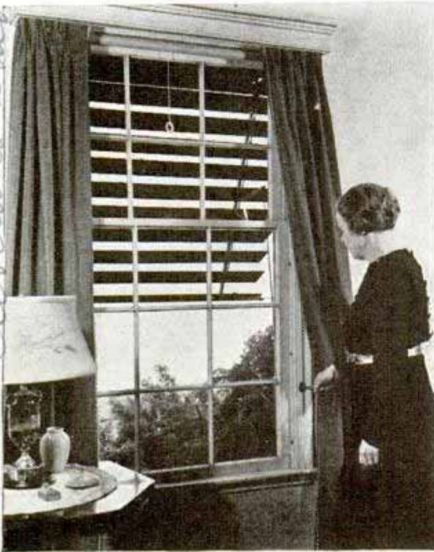
Adjusting the vanes of the outdoor Venetian-type awning by a chain inside the window
