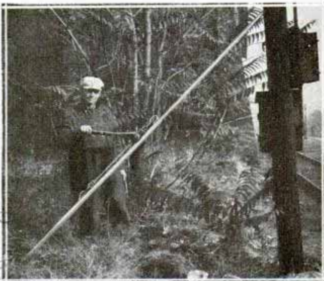
One man can straighten leaning post with telescoping pike pole that is worked similar to auto jack
