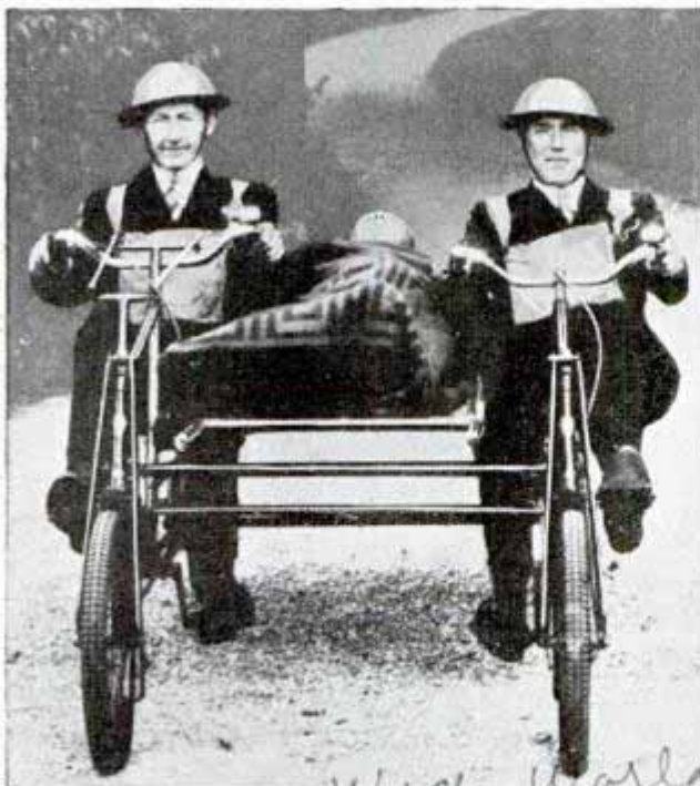
Test run with the bicycle ambulance. Rider on right-hand bike is in control
