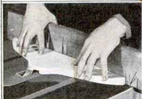
Cutting half-lap joint (coat hanger)
