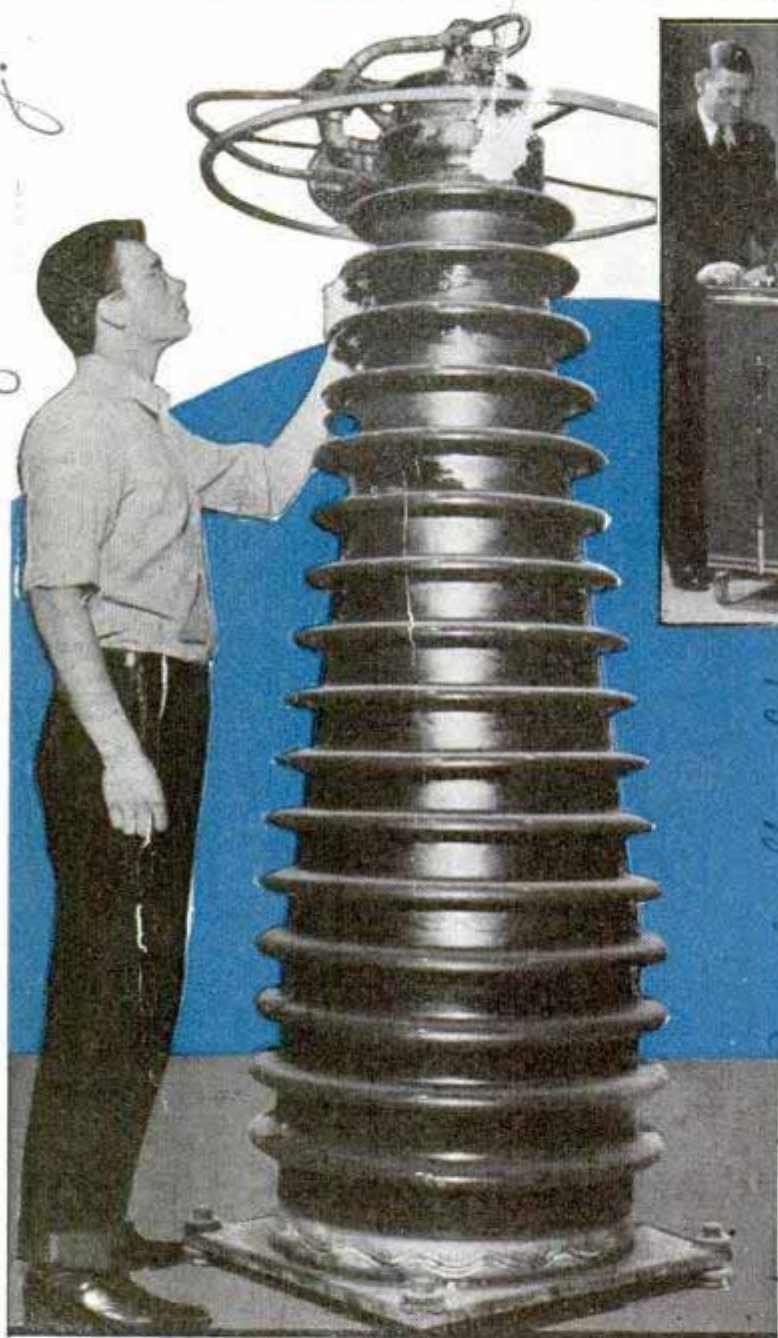
Left, upper electrode of million-volt X-ray tube at California Institute of Technology. Right, new X-ray photography apparatus avoids slow time exposures and gives clearer pictures
