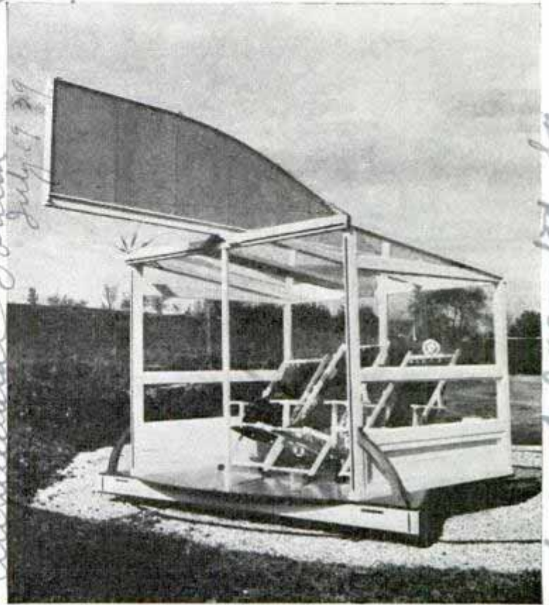
Canvas weather vane keeps glass sundeck facing away from wind, turning it on a circular track. Only the front is open.
