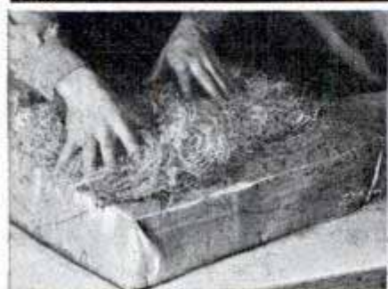
15 FILLING PLACED OVER TOP
