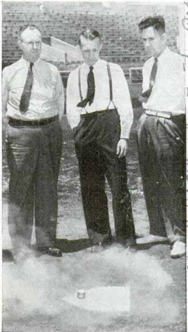
Compressed-air cylinder installed in home plate blows dust away and then sinks out of sight in the base
