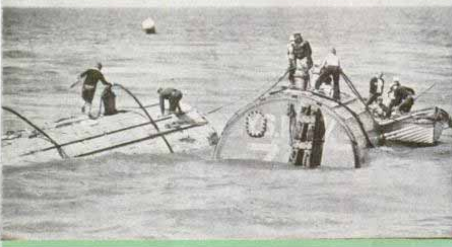
Top, swirling water marks spot where pontoons lifting submarine are nearing surface. Center, the "Squalus" on test run off Portsmouth. Below, navy men inspect pontoons after failure of first effort to raise wreck
