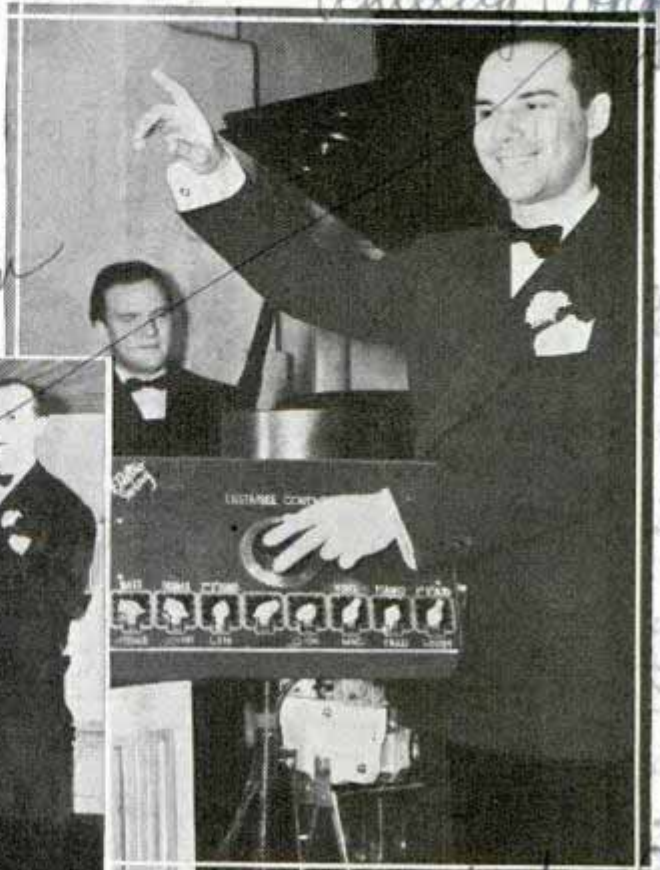
Left, saxophone players with their instruments hooked up to amplifiers are under direct control of orchestra leader who regulates tone volume by turning dial as above
