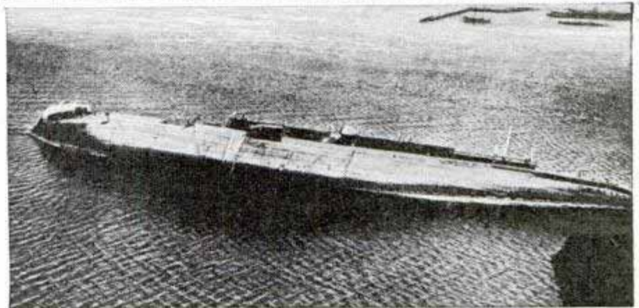
Top, mailboat covered with cement serves as pier for big ship. Bottom, same craft before conversion
