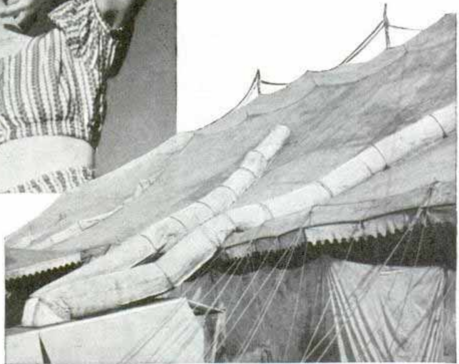
"Big top" performer, above, cools off under breeze from vent of air-conditioning system. Right, two of the ducts delivering "perfect weather" from portable units to points of distribution on the roof of the circus tent.
