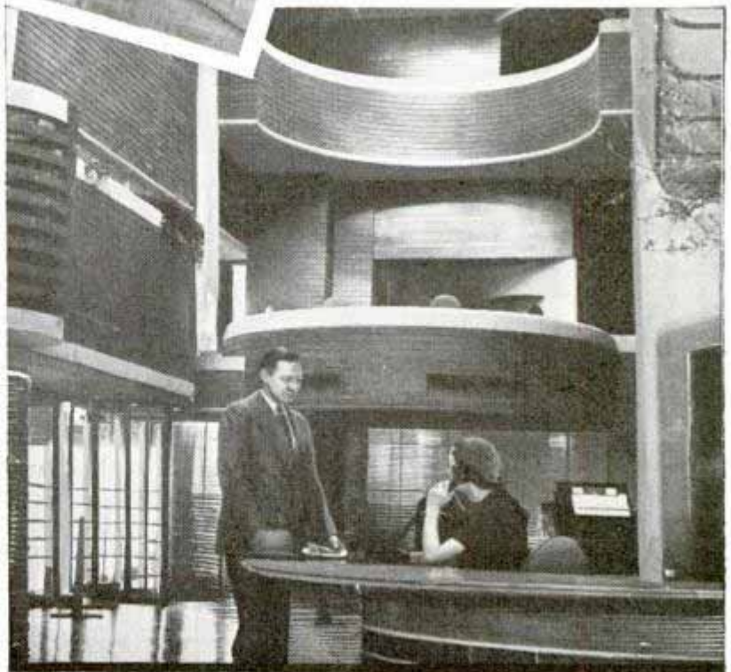
Center, glass-enclosed bridge linking two buildings. Above, glimpse of tapering "golf tee" columns which support roof. Circular stairways between floors save space. Reception hall is seen below
