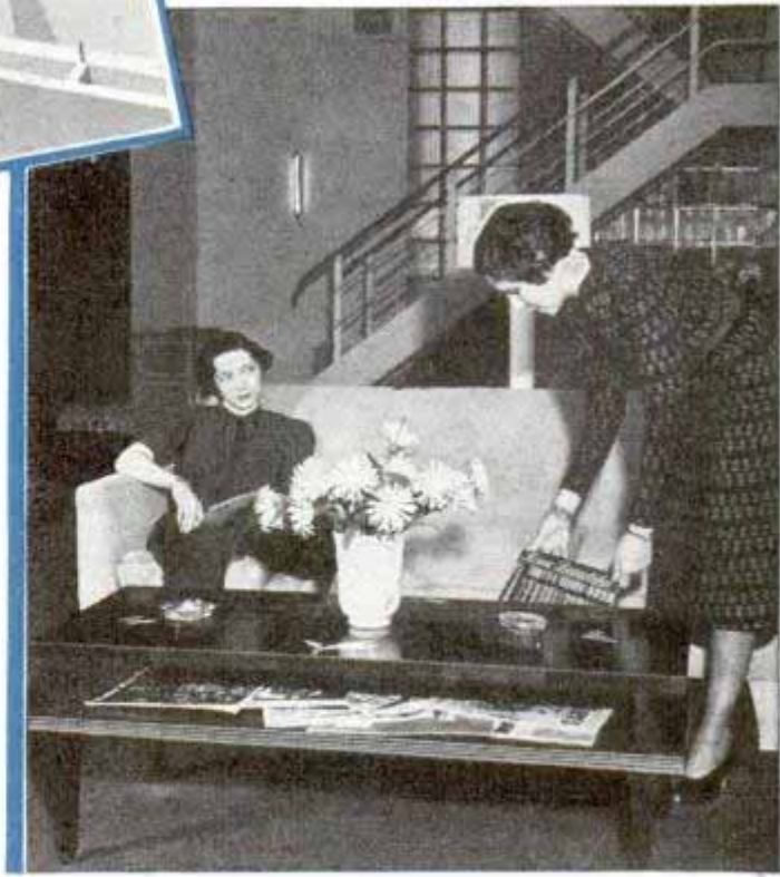
Fireplace heater (top); low-cost concrete house under construction (center) and living room of modern two-story house (bottom). Note free-hanging staircase in background
