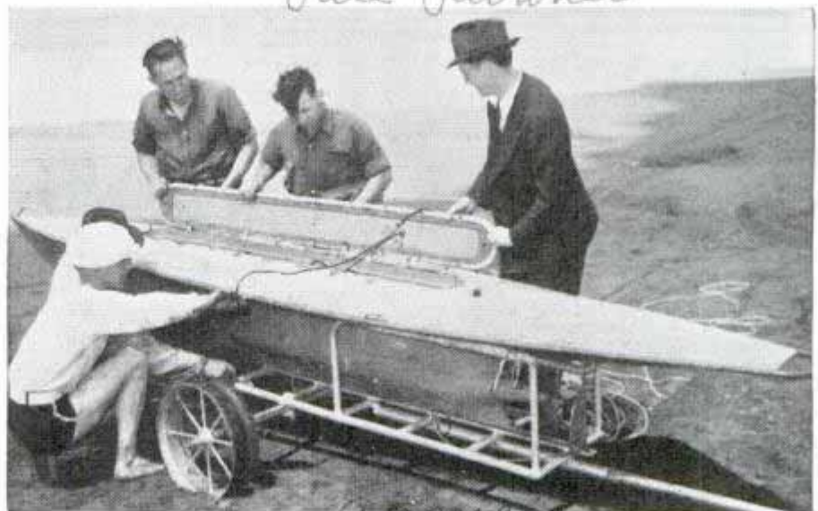
Preparing to launch electric lifesaving boat which is navigated by remote control by coast guardsmen on shore through impulses sent by cable
