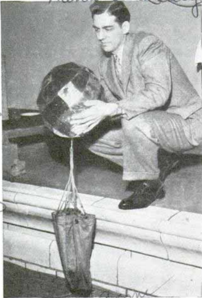
Floating near an airplane down at sea this ball marker would be visible to rescuers ten miles away
