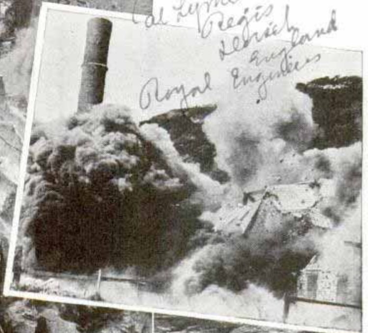
Left, setting blast charges at site of new dam. Below, blowing up a condemned factory building. Circle, view of Wyoming dam site just as blast was set off. Bottom, preparing charges for breaking lump coal off face of mine Photo courtesy du Pont company
