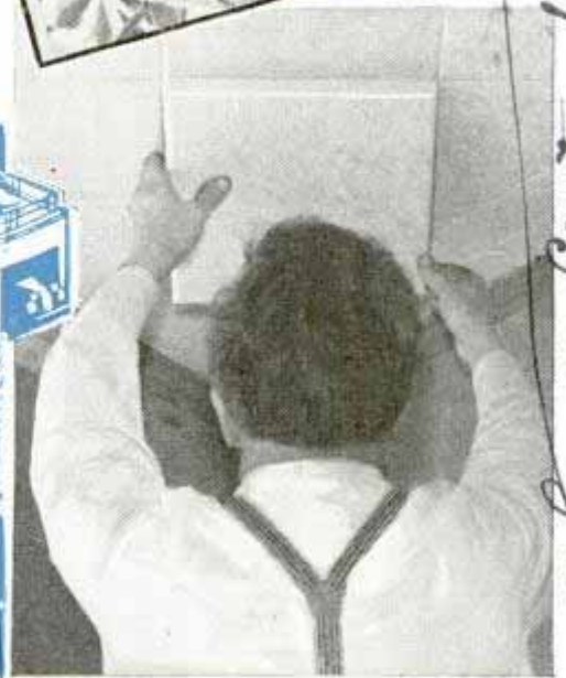
Attaching sound-absorbent material to studs (top, right); bird's-eye view of concrete forms for low-cost house (center); box-room form suspended in air (bottom, left) and sheathing ceiling with sound-absorbent material
