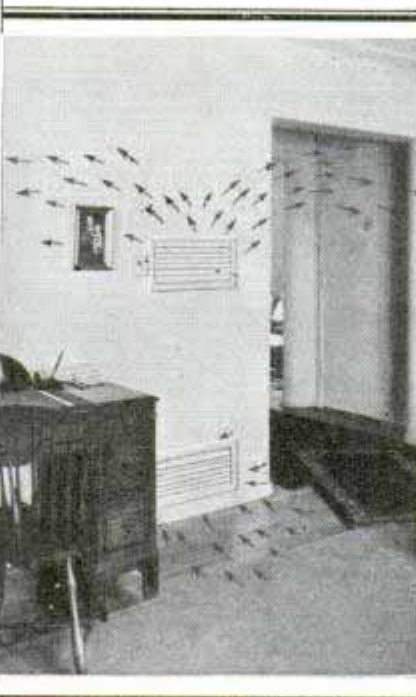
Diagrammatic drawing of gas heater built into wall, and photograph of finished wall showing grilles for air circulation
