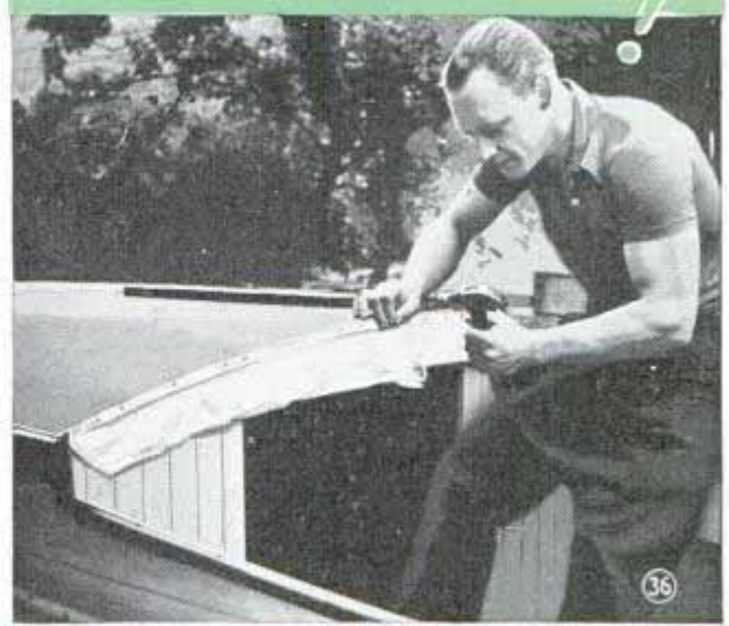
INTERMEDIATE BEAMS SUPPORTED ON CLEATS
