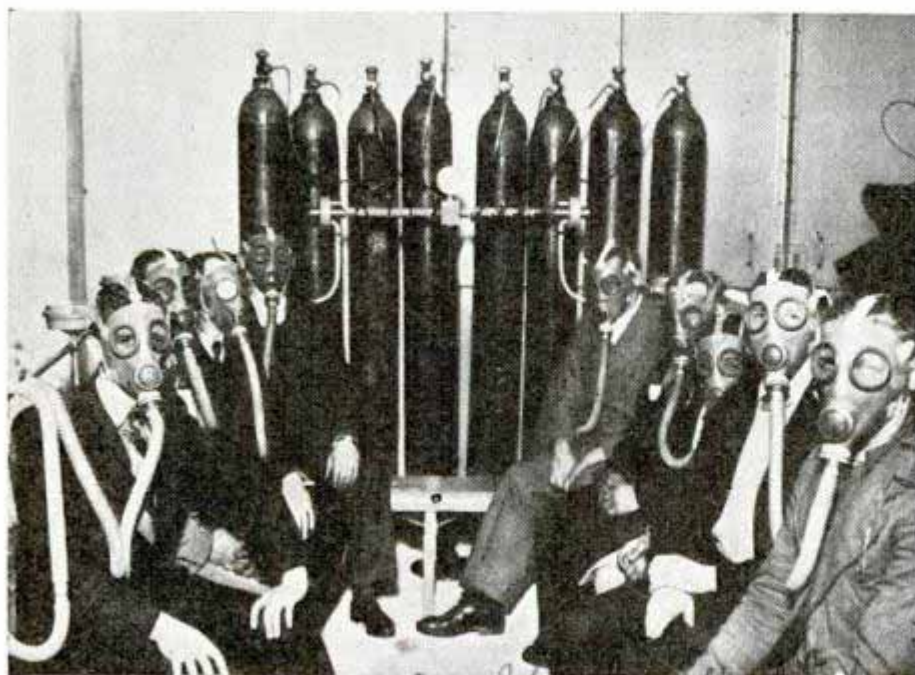
Instead of using individual oxygen "bottles," the gas masks all tap a common pipe line fed by large oxygen tanks in air-raid refuge
