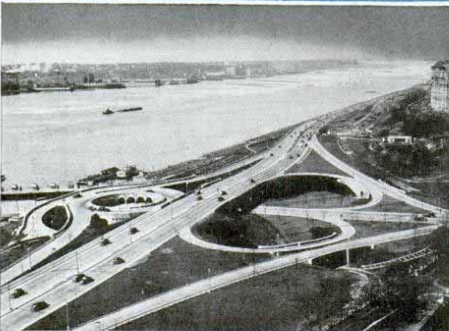
Left, Riverside Drive in New York demonstrates highway grade separation of cloverleaf type used at heavily traveled intersections. Above, same spot illuminated at night
