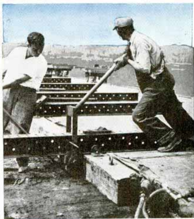
Top, testing qualities of low-type road surface in U. S. Bureau of Public Roads laboratory. Center, dividing concrete highway by moving slabs laterally with aid of compressed air in fire hose. Bottom, automatic traffic counter aids in highway planning
