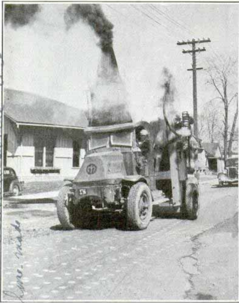
Dots on pavement are marks left by the hammer as it moves along, the distance apart being regulated by speed of the truck
