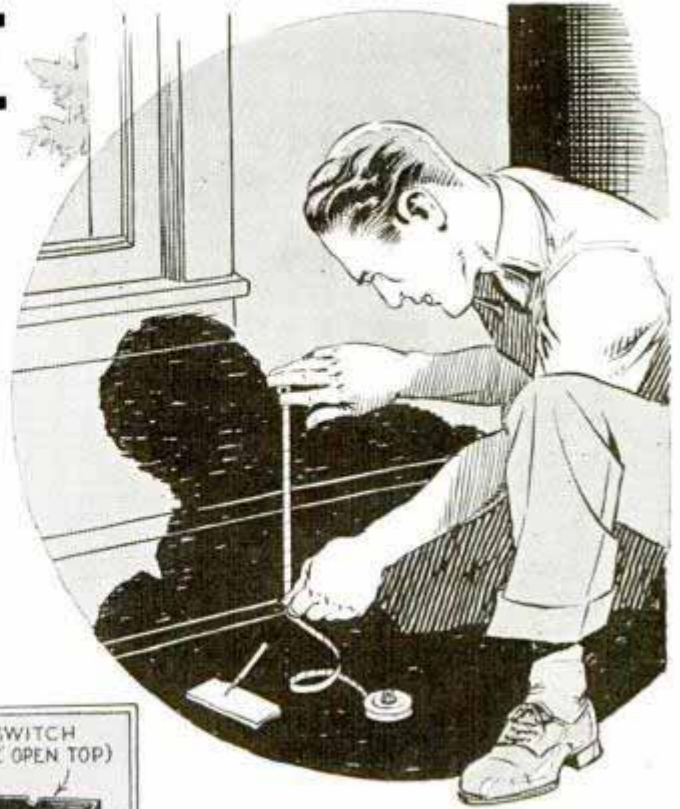
All convenience outlets should be spaced the same distance from the floor for uniformity of appearance
