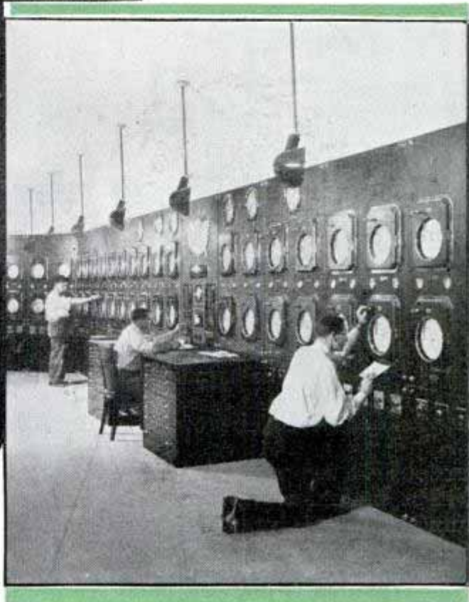
Left, pump and tank for washing air supplied to NBC studios in Radio City. Below, right, control panel for regulation of temperatures in twenty-seven radio studios
