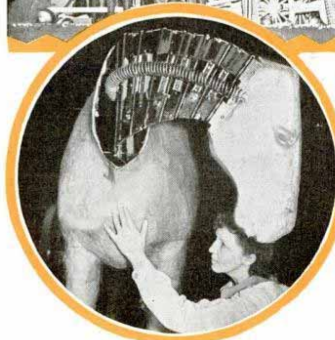
Above, core of horse's neck is made so that the head can be moved. Motor is mounted in the body, which is made of laminated paper. Group sets are generally operated by control boxes, each with six to fourteen cams. Interior motors in figures are controlled by mercury switches. Rockers, pitmans, working pieces of rack against tooth gear, and weight lines all help to give grace and smoothness to the dummies' actions
