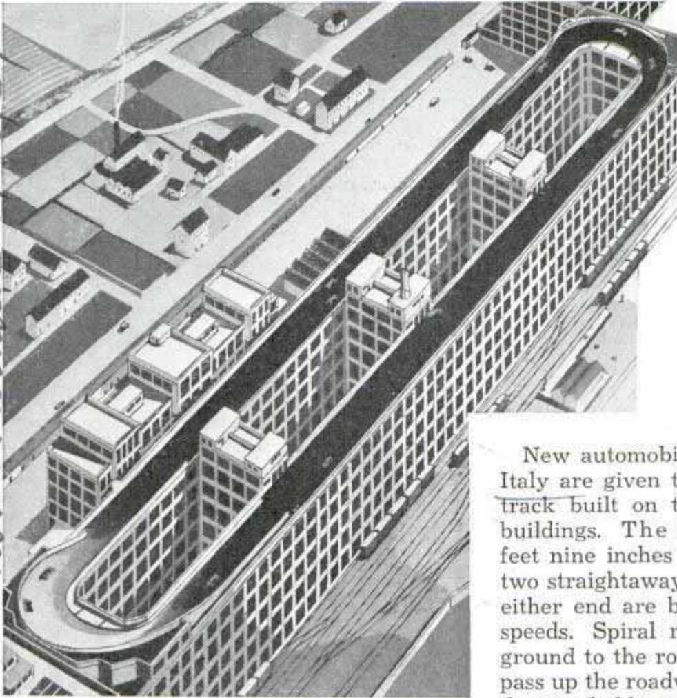
Left, race track on roof of factory buildings where cars are given their first test. Right, spiral roadway for reaching the roof
