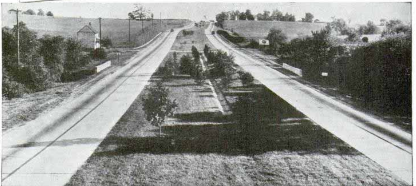
Top, portable device used to weigh trucks. Center, elevated routes with opposing streams of traffic minimize chances of accidents. Bottom, divided roadway helps reduce accidents
