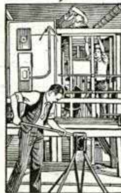
HOUSE WIRING only one of the many branches you "Learn By Doing."
