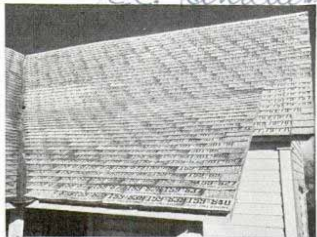
Oklahoma residence shingled with leftover license plates obtained from the state factory
