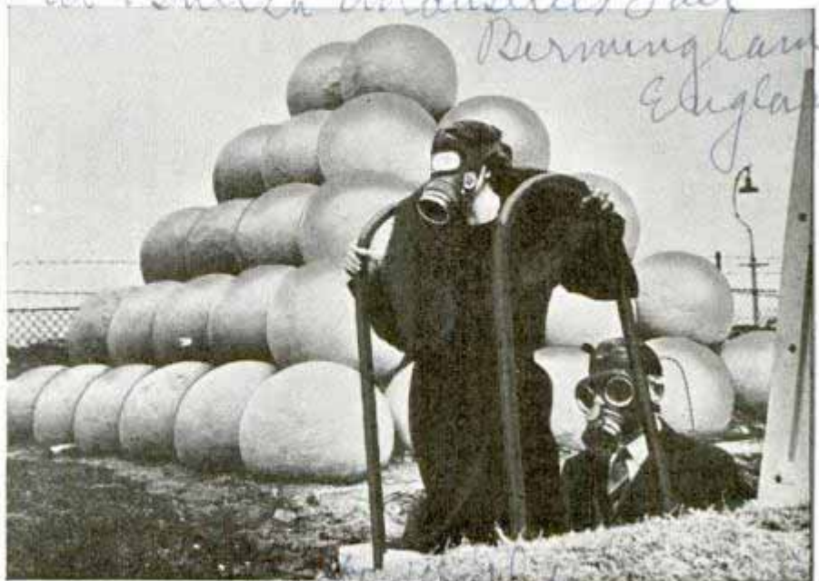
Concrete balls piled in pyramid at surface of a bombproof refuge deflect the shock of explosives falling near the shelter
