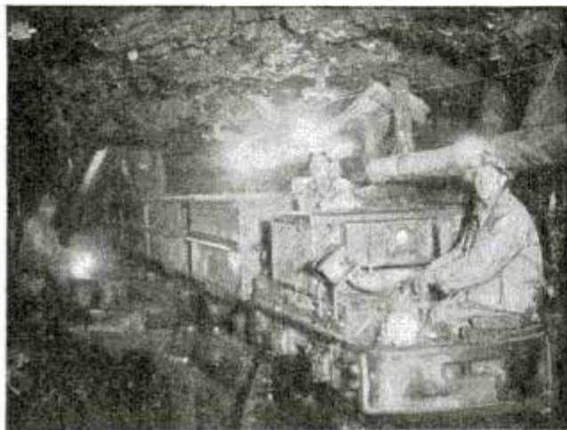
Electric locomotive hauling ore cars in a deep mine. Notice the ventilation pipe at right
