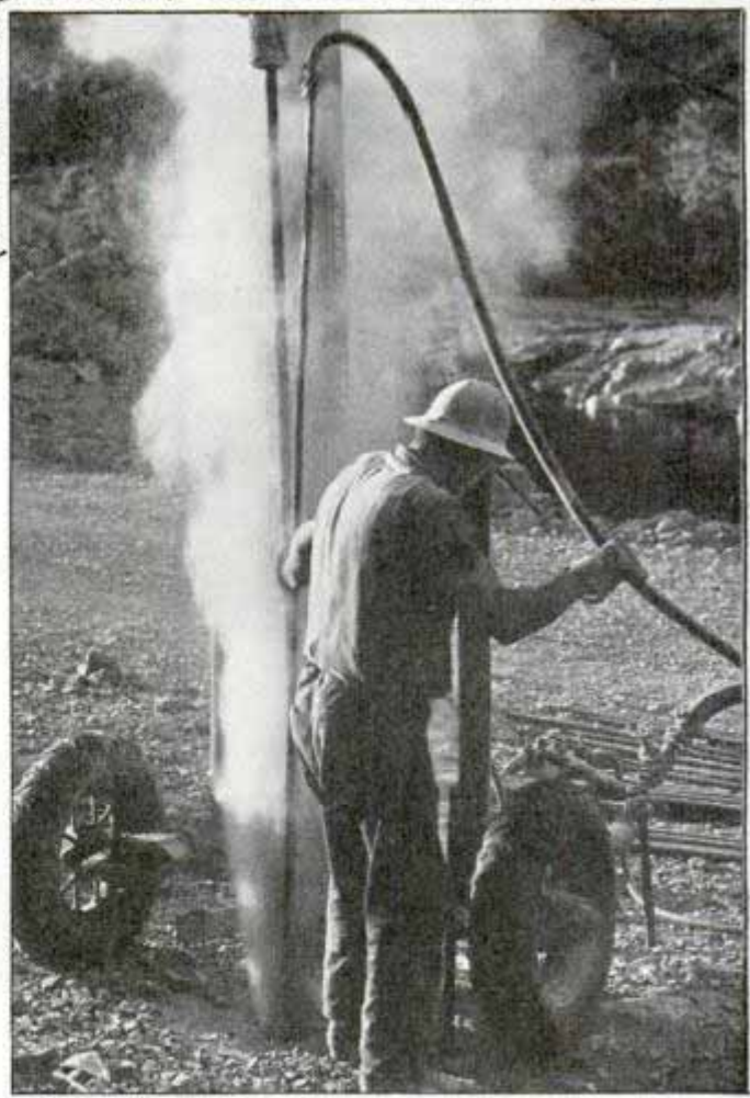
Top, drawing of Shasta Dam and power plant. Bottom, workman blowing rock dust from hole being drilled at Shasta Dam site
