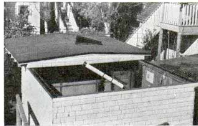
Roof of home observatory rolls out of way so amateur astronomer can point telescope into night sky
