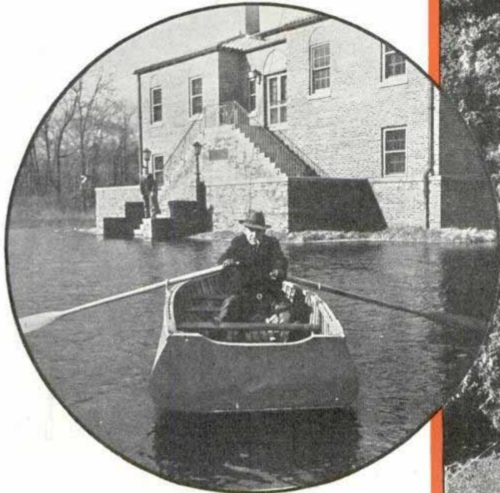
Circle, rowing to work is a regular occurrence in transmitter technician's life. In background is the Wayne plant. Right, bird's-eye view of Columbia's transmitting plant. The steel tower, which radiates the radio impulses, is 550 feet high
