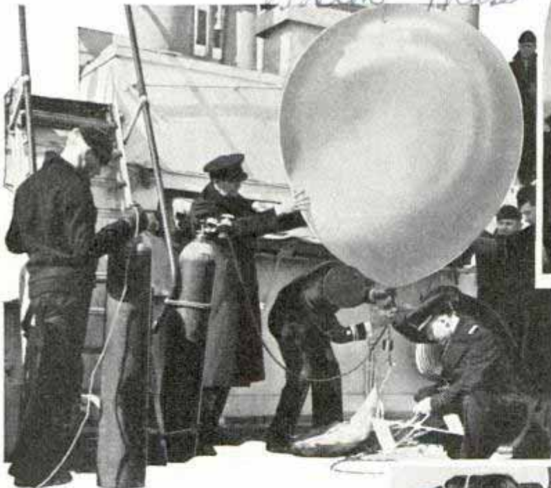
U. S. Coast Guard Top, left, Lieutenant Commander Edward H. Smith, commanding the cutter "Chelan," and Lieutenant Ned Sprow preparing radio meteorograph for trip aloft; right, sighting departing balloon with theodolite, to compute wind velocity and direction
