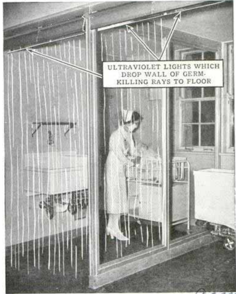
Science White lines sketched into the picture represent the invisible screen of ultraviolet light that purifies air in nursery
