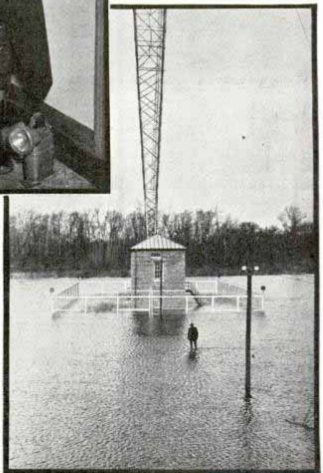
Top to bottom, photos showing how useful hip boots are to the radio "hermits" when flood waters rise around the Wayne plant
