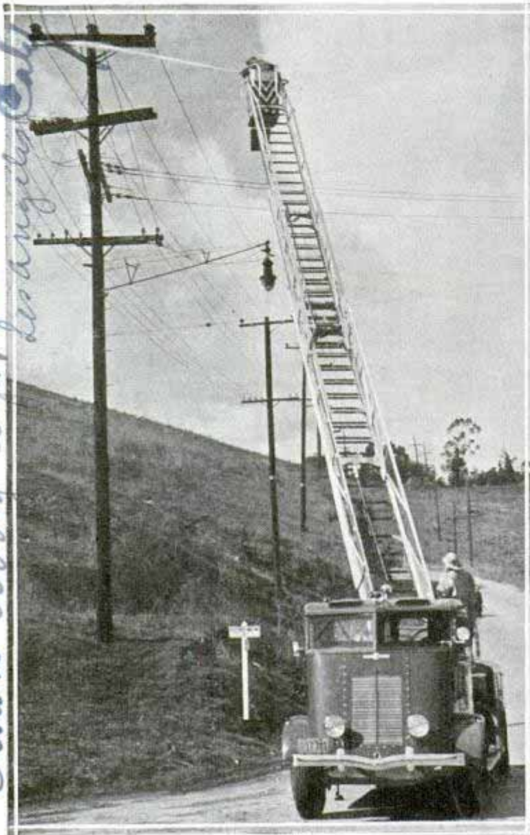
Above, spraying corrosion and dust from power-line insulators with high-pressure stream of cleaning fluid. Right, with seventy-five-foot turret ladder retracted, the "wash truck" moves on to a new location
