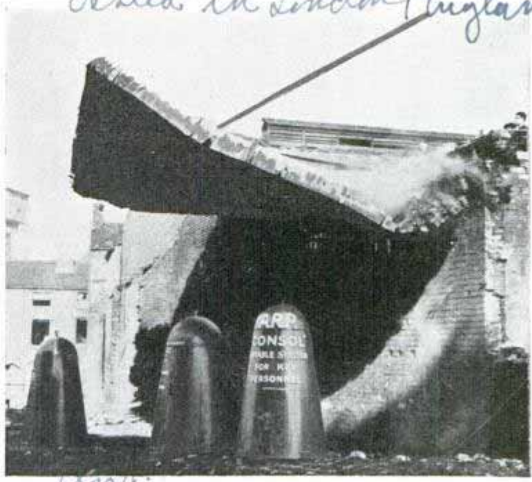
Air-raid shelter standing under collapsing wall in severe test simulating war conditions remained undamaged from shock
