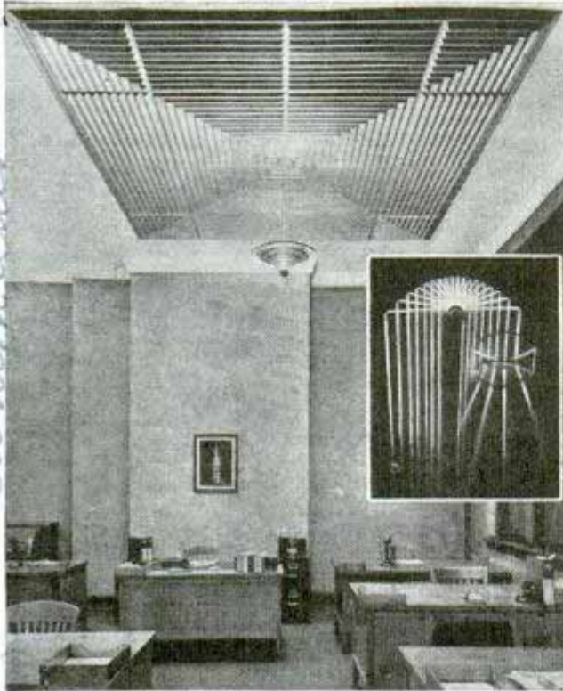
Parabolic reflector distributes light evenly from flat ceiling. Inset shows path of light beams
