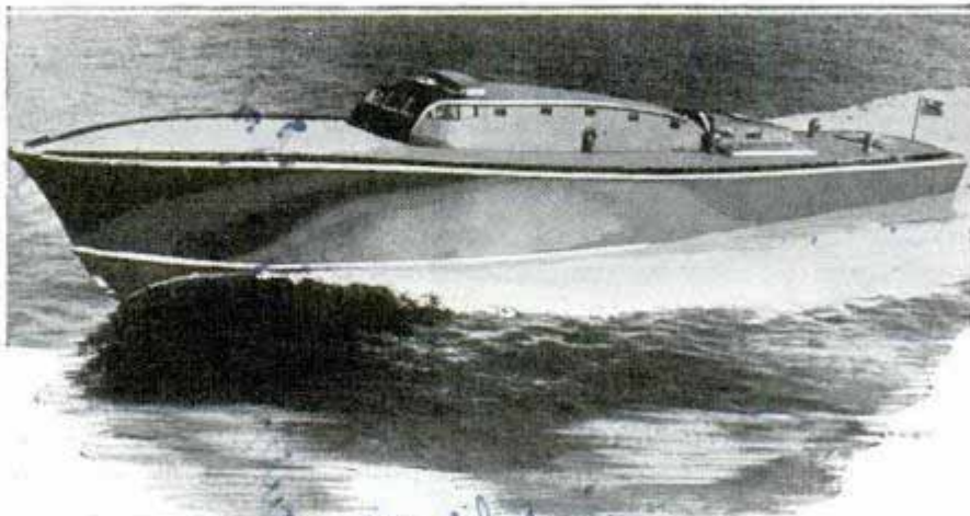
Britain's high-speed streamline torpedo boat without mast or funnels, said to be world's fastest warship, made fifty miles an hour in trials. It is powered by three 1,000-horsepower engines
