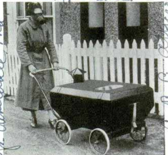
Pressure of rubber bulb expels stale air and sends new supply of filtered air into gasproof pram
