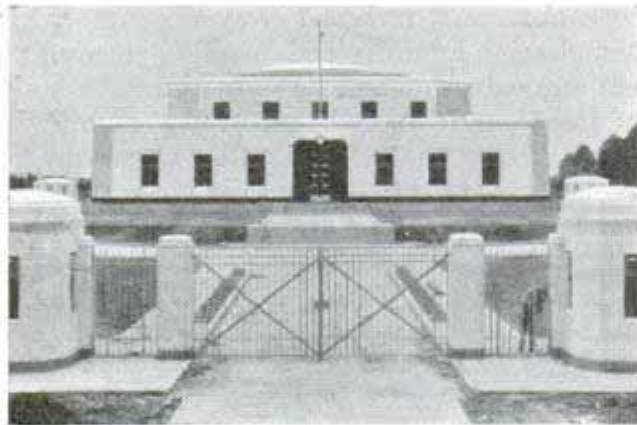
Beyond the well-guarded gate lies Fort Knox Depository, "strongbox" for six billion dollars in gold
