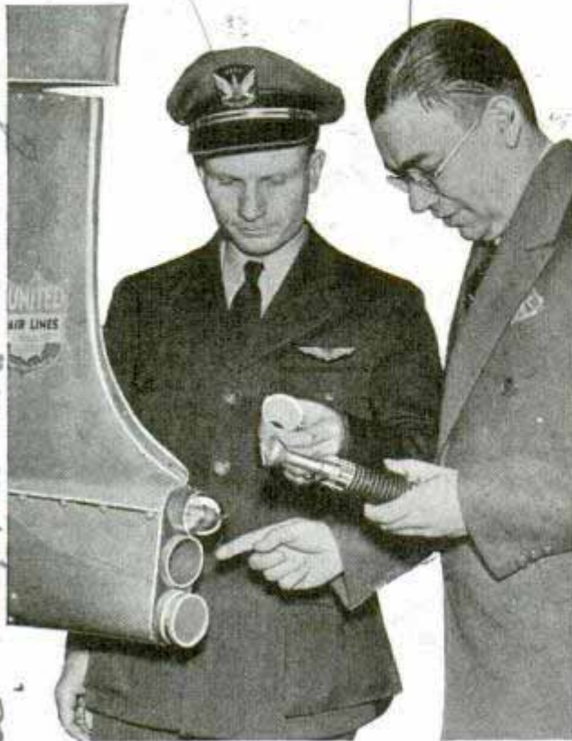
Long wire which "drains" static from airplane is shot from socket in tail at touch of button in cockpit
