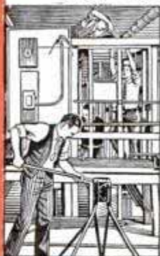
HOUSE WIRING only one of the many branches you "Learn By Doing."
