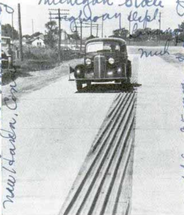
Safety grooves down middle of highway nudge car back to right side of road by gripping the wheels
