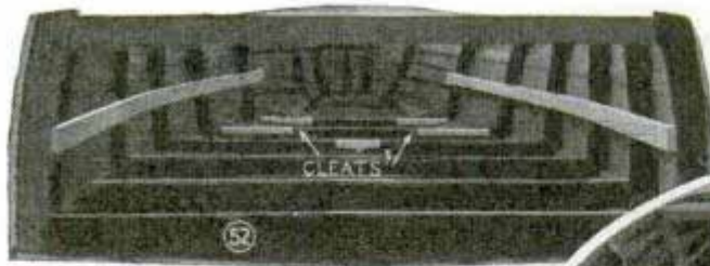
Above, seat risers and floor cleats in place. Photo at right shows flooring nailed in place
