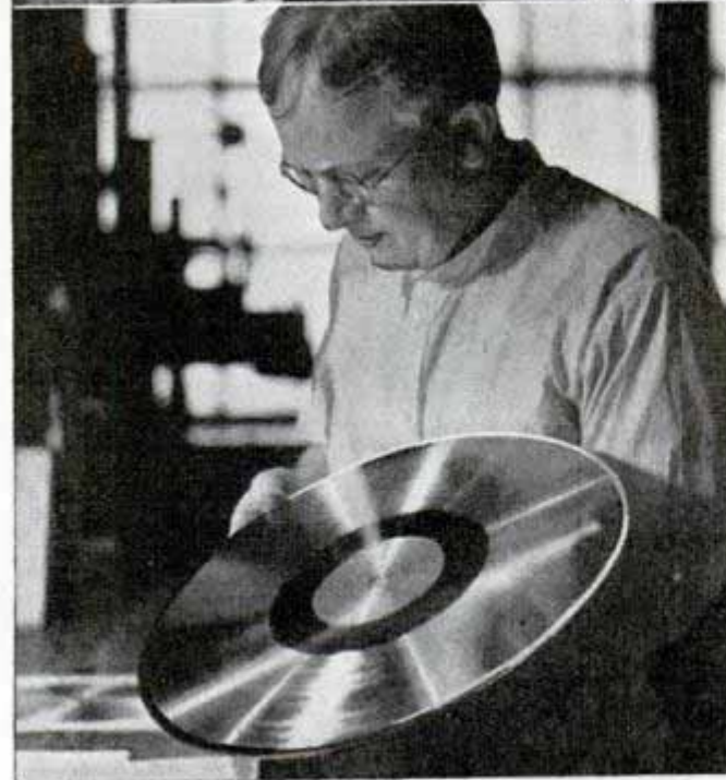
In taking off "lost voice" from fragile original record with aid of delicately cut sapphire, cylinder is played through amplifier to modern master disk, top. Center, record taken to R.C.A. laboratory is recorded on wax disk. Bottom, modern record on which voice is reproduced for posterity, and, right, Victor record just pressed and still retaining excess "dough" on edges
