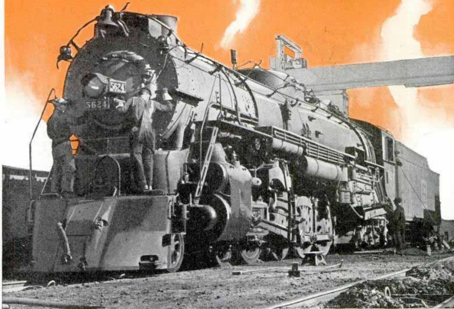
Just in from Minneapolis, No. 5624 submits to thorough inspection by electricians and mechanics in Chicago yard while fire is "pulled." Note ash buckets in adjoining track
