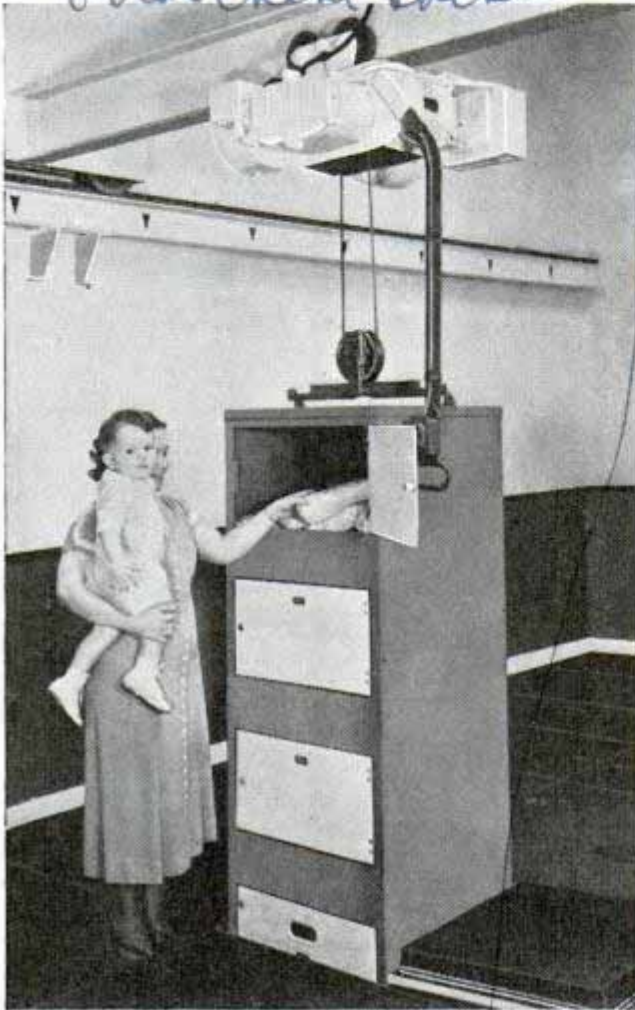
Cold-storage locker is hoisted by overhead lift from refrigeration chamber into warm room for customer
