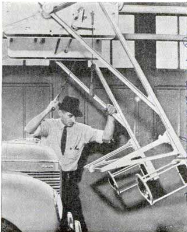
Pulling the optical tester on its hundred-foot trestle into position for focusing car headlights
