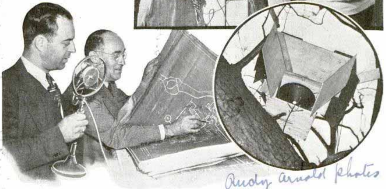
Bottom, issuing building order over the office "mike." Circle, loud speaker in tree carries message to all workers on the job. Top, field engineer calls back on tree 'phone for further instructions
