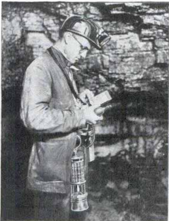
Left, sampling air at working face of mine with detector to find if gas is present. Right, sampling line and mechanical nose in use to discover gaseous condition in manhole
