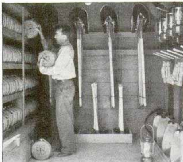
Interior of forest-service "firebox" shows equipment for fighting the flames
