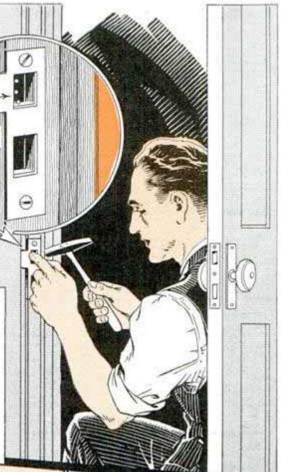
SMALL BRADS DRIVEN FLUSH WITH PLATE
