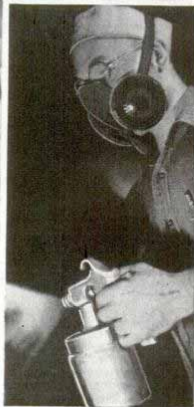
Left, scattered spots of light in the huge RCA building in New York show where hard-working women are scrubbing offices, another task in the process of keeping the skyscraper polished. Right, bronze cleaner, wearing mask, uses electric gun to spray on polishing fluid. The mask protects his lungs against fumes
