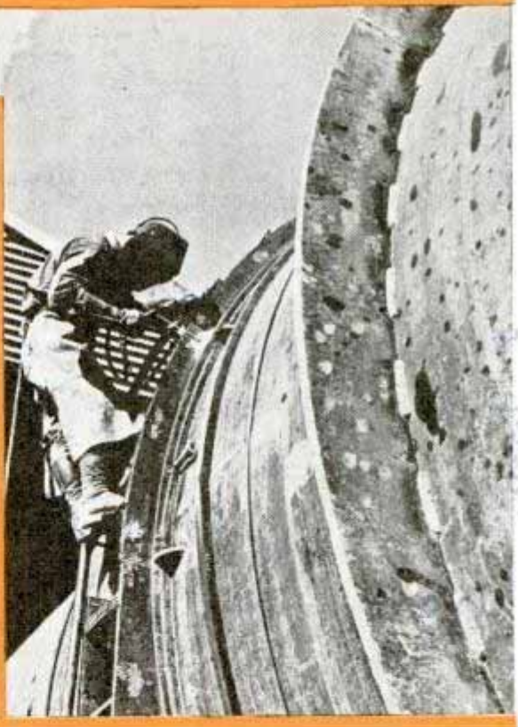
When Grand Coulee dam is completed it will be man's mightiest structure, a monument to engineers and workmen who risked life every day on dizzy heights of its skeleton. Its 550-foot wall will back up a lake 151 miles long, nearly a mile wide, developing 2,520,000 horsepower and irrigating 1,200,000 acres. At left, top, workman attaches a line to compressed-air "main"; right, crane swings men over foamy water to base of dam. Bottom, latest view of dam, and welder on penstock
