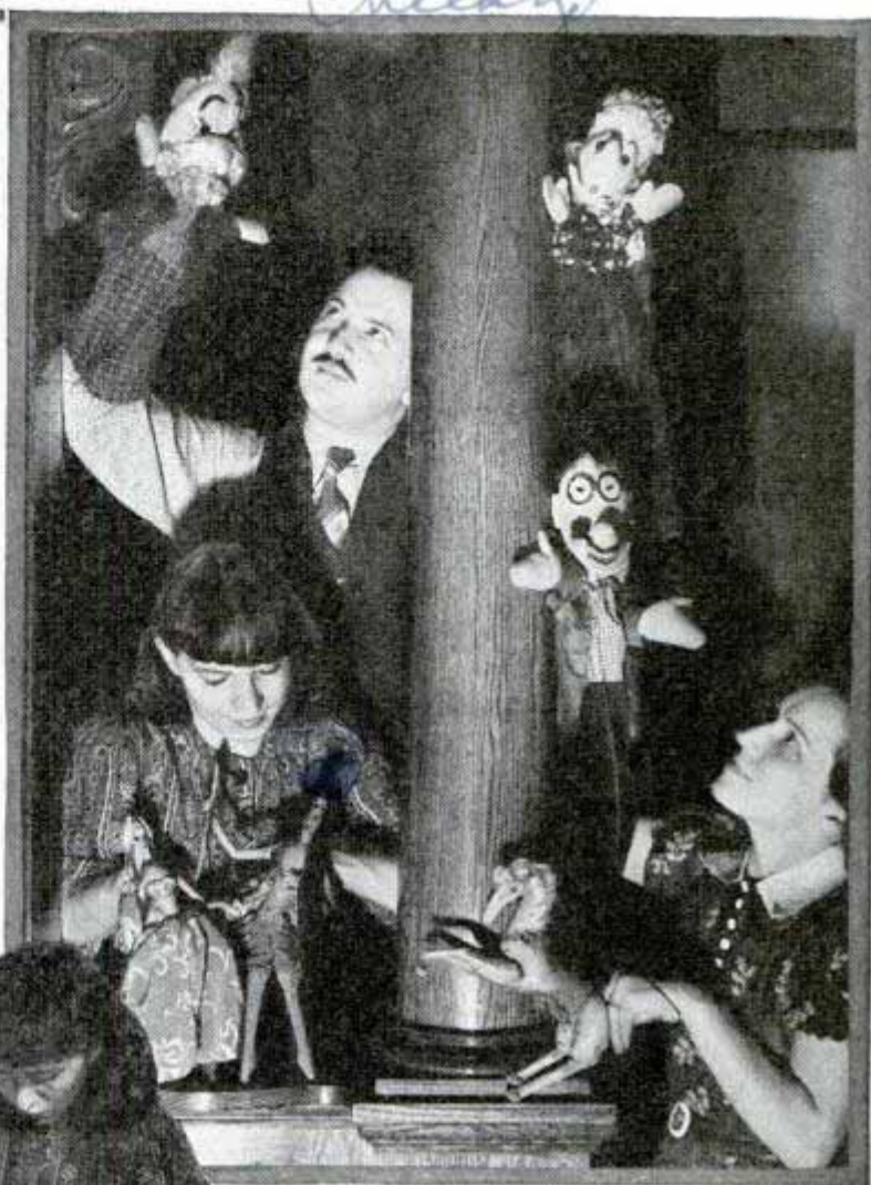
Black backdrop near table edge brings out light-costumed dolls by contrast and operator's arms, wrapped in black, are almost invisible. When room is darkened for show, ordinary battery flashlight provides spotlight effects. Operator at left is holding colored glass in front of flashlight
