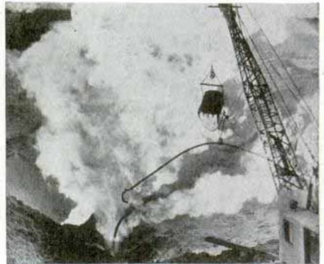
Dredge trying to catch piece of broken casing with hook to pull it from crater
