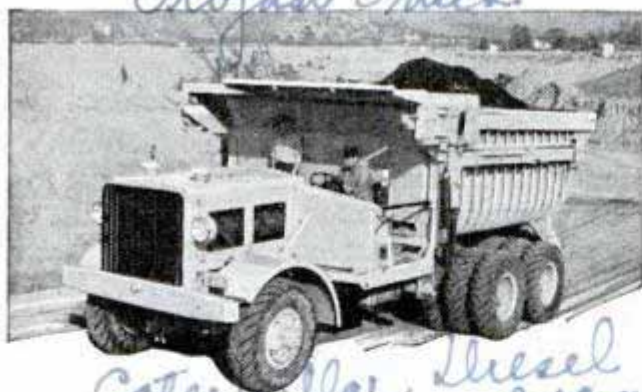
One of the biggest trucks ever made for earth movement moves eighty-five cubic yards per hour
