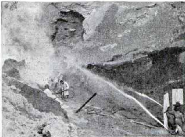
Asbestos-clad men making cable fast to casing at the bottom of the crater
