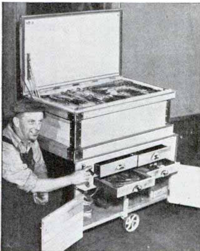
Compressed air, controlled by three levers, opens lid and drawers of this maple tool chest
