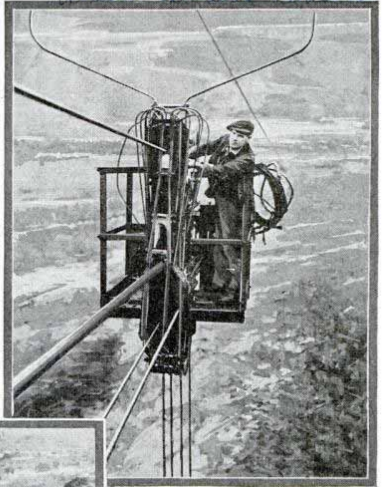
Here another daring worker appears unworried by the fact that he is oiling a skip carrier on a cableway 150 feet above the site of a large dam
