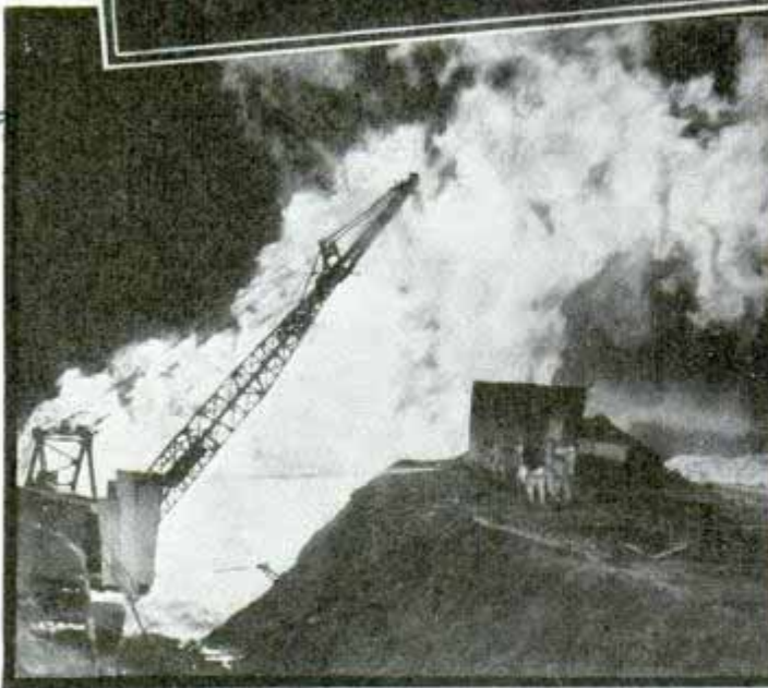
Top, fire fighters inspect flaming oil well from behind tin shields. Bottom, left, dredge being sprayed with water as it digs away dirt from buried casing. Right, casing being pulled into position with cables. Note size of the crater. In this photo the fire has been extinguished, but stream of gas and oil rushing from casing is visible
