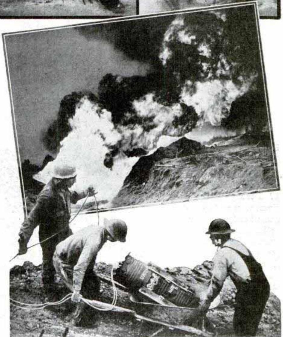
Top, left, Patton's capping machine in crater with manifold enveloped by flames. Center, men in tin-shielded boat on boiling lake. Right, dropping swedge into casing. Below, fire breaks out in new spot as swedge restricts flow in casing. Bottom, wheeling nitroglycerine into crater
