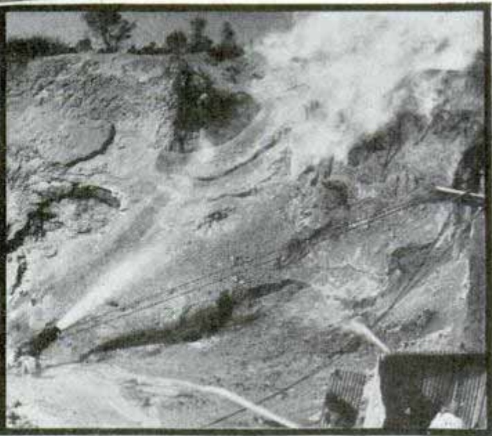
Top, fire fighters inspect flaming oil well from behind tin shields. Bottom, left, dredge being sprayed with water as it digs away dirt from buried casing. Right, casing being pulled into position with cables. Note size of the crater. In this photo the fire has been extinguished, but stream of gas and oil rushing from casing is visible
